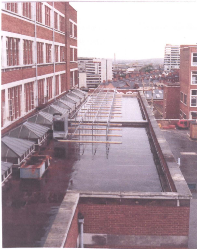
Plate 3.3: Completed Construction of the Framework
