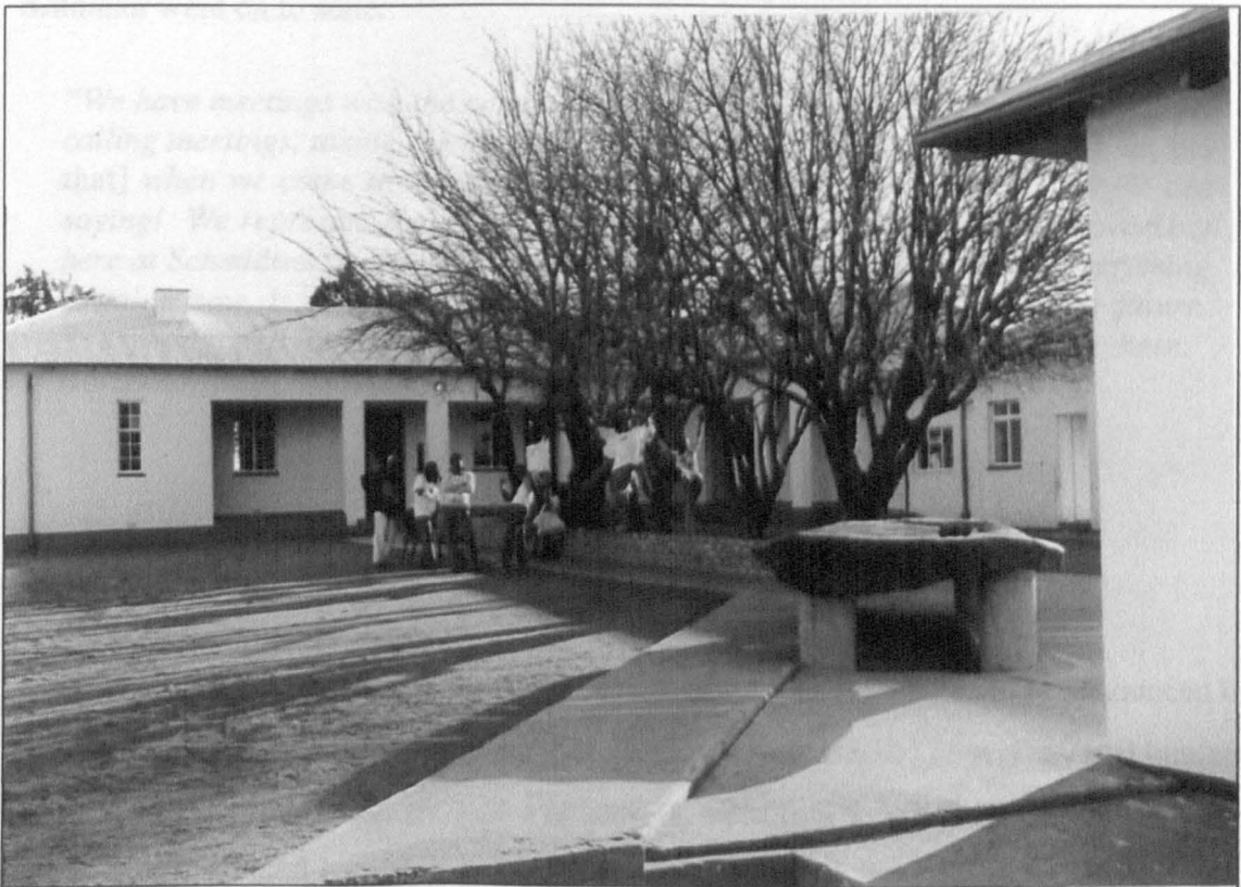
Schmidtsdrift administration offices in the converted SADF buildings, 2001
