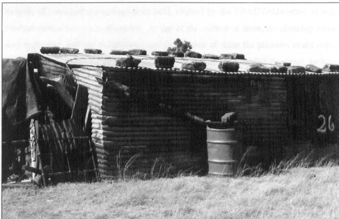
Typical dwelling erected by returnees at Mogopa, 1991
