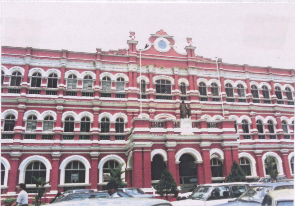
Figure 4.17: St. John's Institution (1904) is one of the first schools to be built in Kuala Lumpur.
