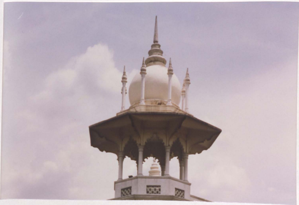
Figure 4.38: A dome surrounded with pinnacles in the Kuala Lumpur Railway Station.
