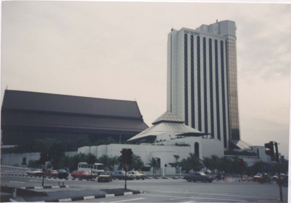
Figure 5.11: The Putra World Trade Centre complex (1985).
