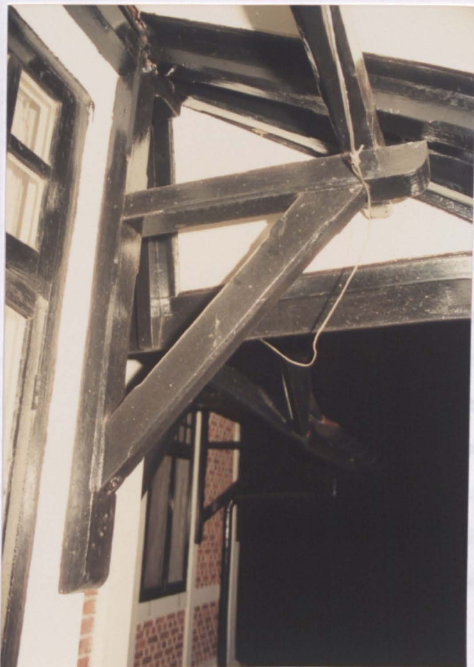
Figure 4.32: Example of a timber bracket in a colonial house.
