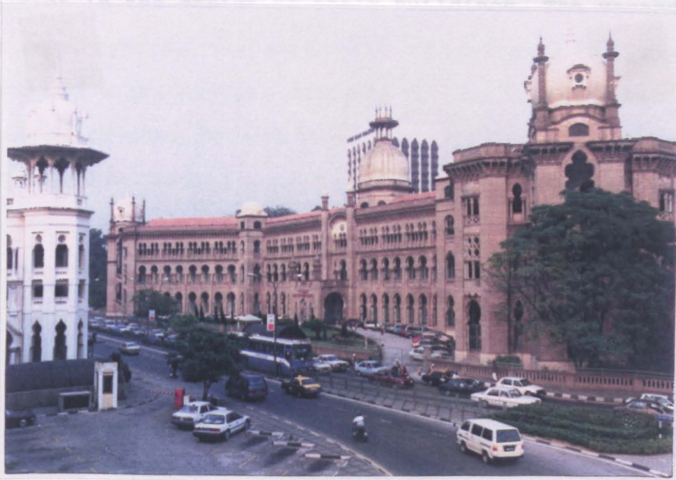
Figure 4.30: KTM Administration Headquarters, Kuala Lumpur (1917). Its facade displays an extensive use of loggia.
