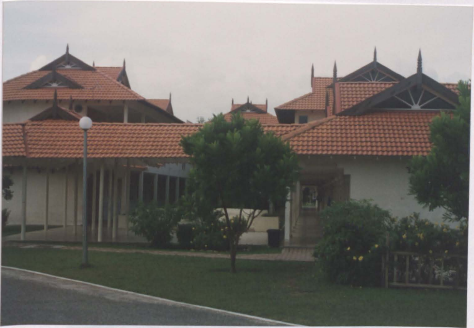
Figure 5.22: The interplay of 'bumbung perabung lima' with finials creates an interesting visual form.
