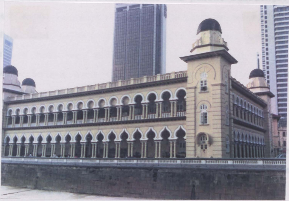
Figure 4.27: Round and pointed arches in the High Court building, Kuala Lumpur. (1909)
