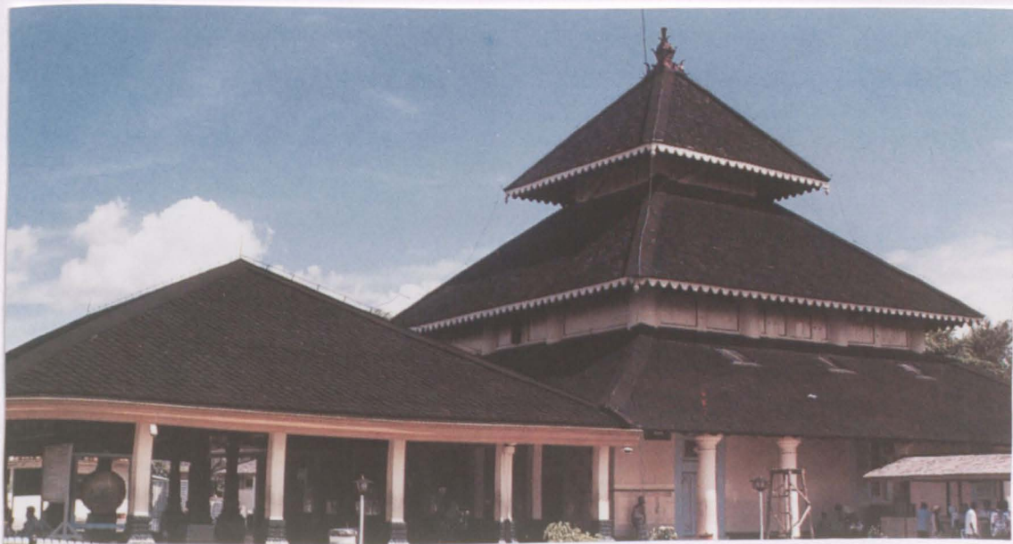
Figure 2.9: The Royal mosque of Demak, near Semarang, Java. Built around 1480, it was repaired time and again, extended and restored in recent years. 17
