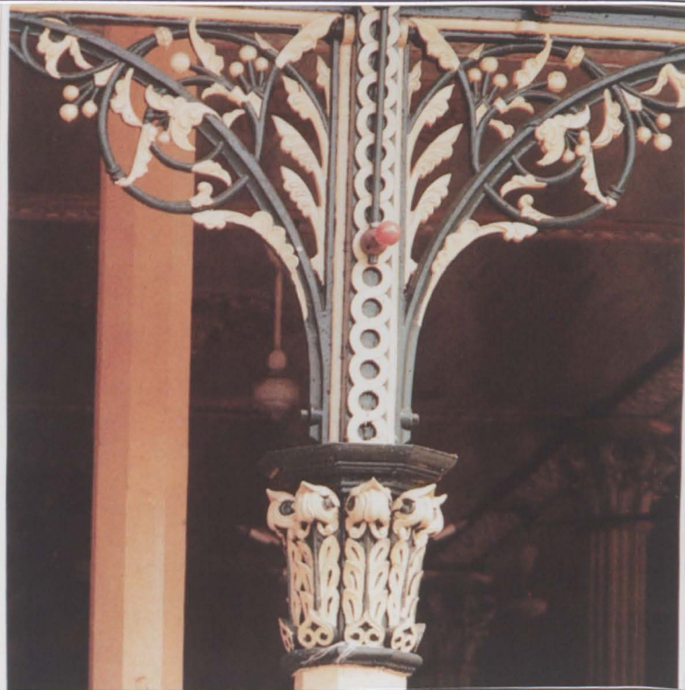
Figure 2.19: Details of a column which supports the main roof of the Balai Besar. 41
