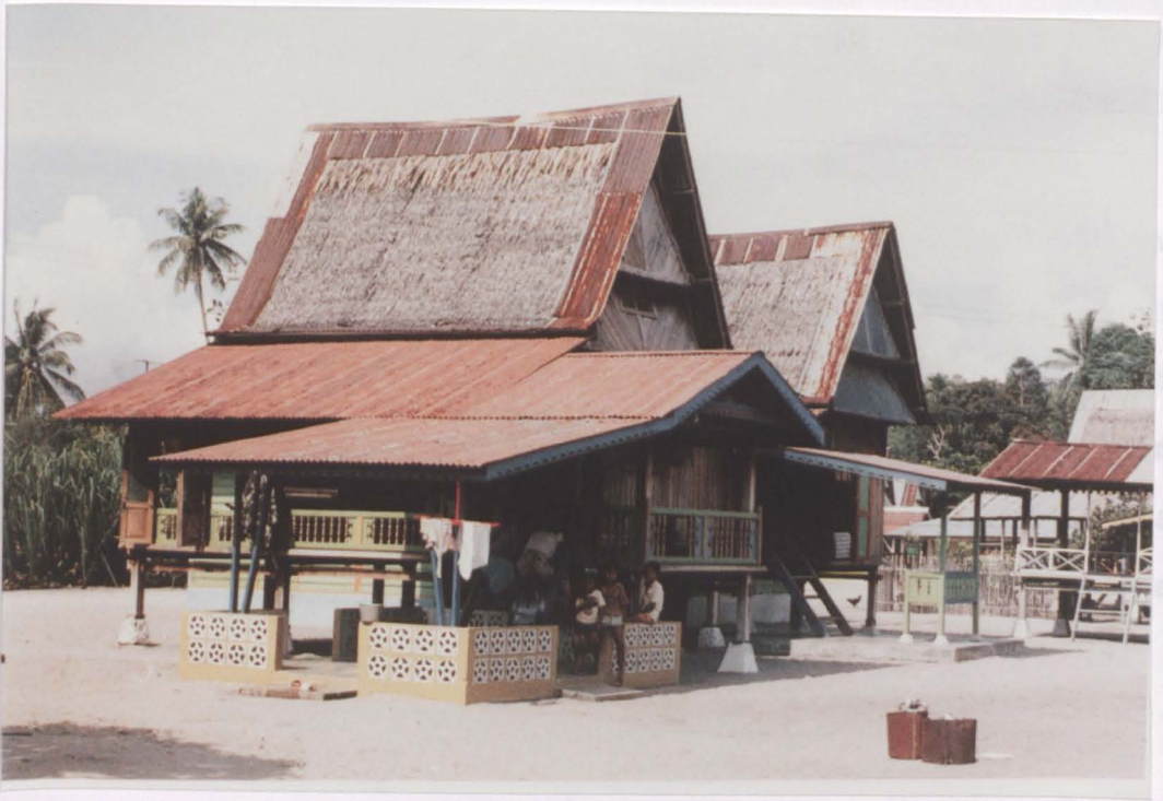
Figure 2.13: 'Bumbung Panjang' (gable roof) with 'Serambi' (attached covered verandah) in a Malaccan house. 28
