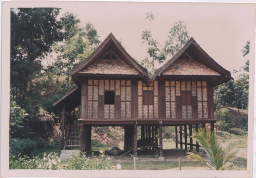
Figure 2.57: Vent holes (clerestory windows) and woven panels facilitate natural ventilation in Malay houses.
