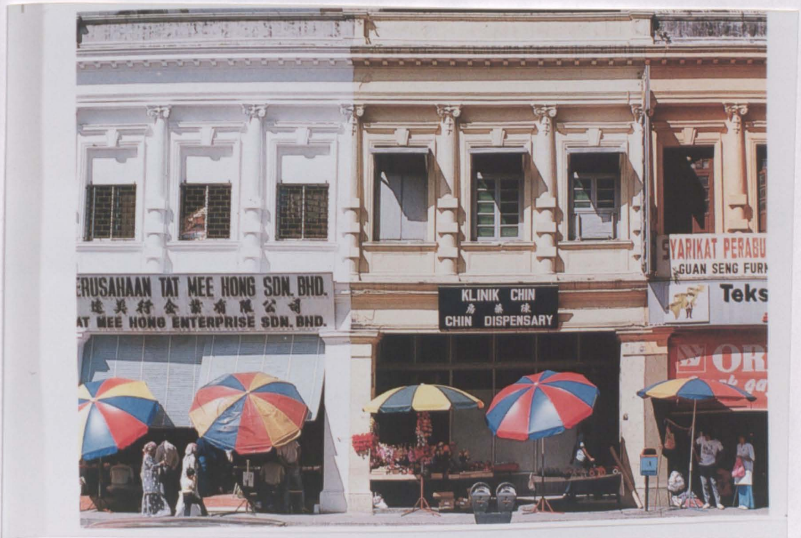
Figure 3.5: A repetitive facade with European features in the design of early twentieth century shophouses in Jalan Tuanku Abdul Rahman, Kuala Lumpur. 52
