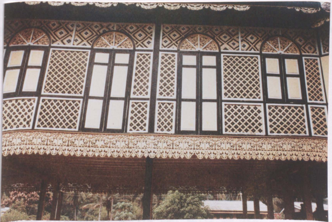
Figure 2.58: Extensive use of woven panels in Istana Kenangan, Kuala Kangsar, Perak.
