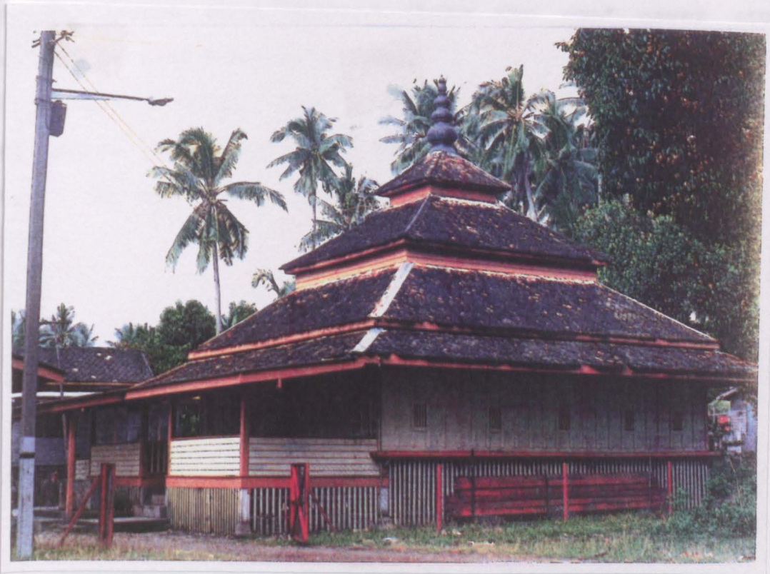
Figure 2.63: 'Mahkota Atap' (roof crown) of Tok Tuan mosque in Kemaman, Terengganu. 119
