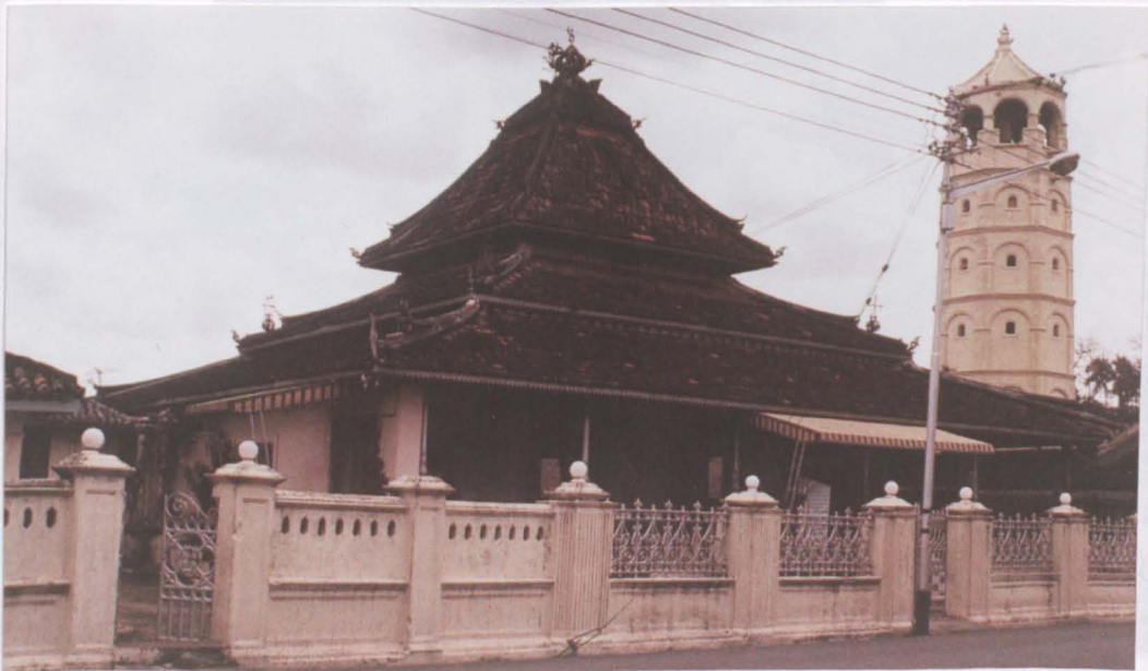
Figure 2.14: 'Atap Meru' of Terengkera mosque in Malacca. The building was built in 1728. 29
