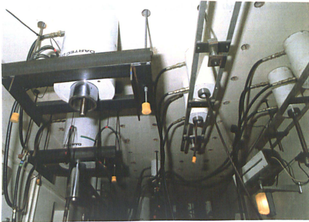
Figure 5.9 : View of the hydraulic loading rams housed in the basement beneath the test area.
