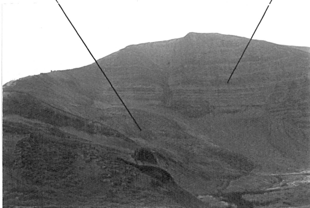
PLATE 3.1 Back scarp and retrogressive scarps of Mam Tor.
