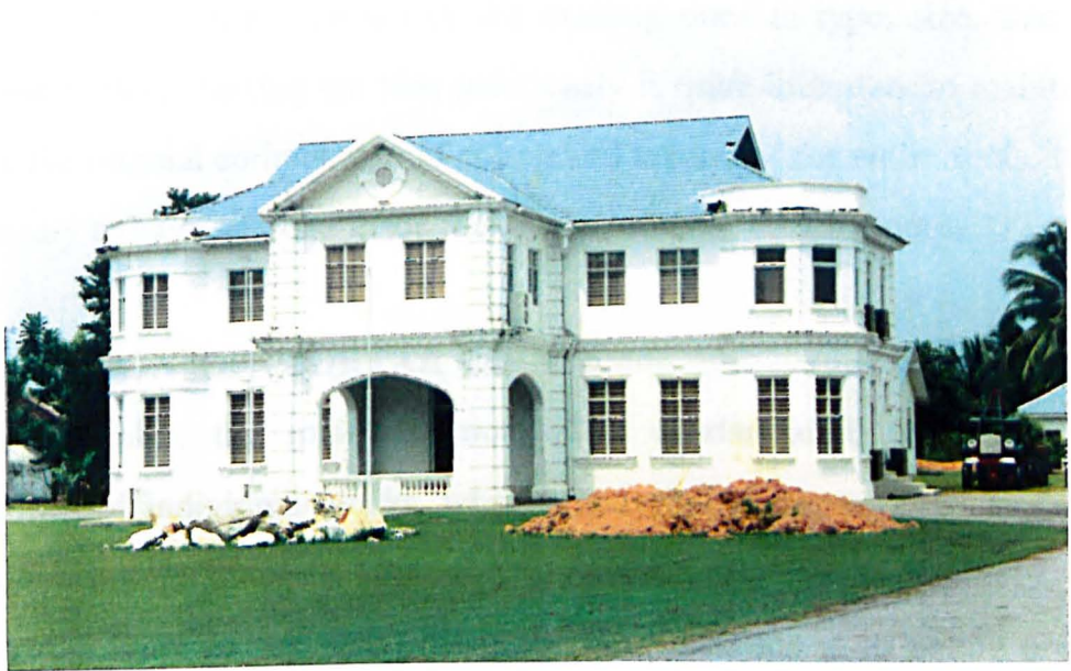
Fig.54 Old and new roof tiles
