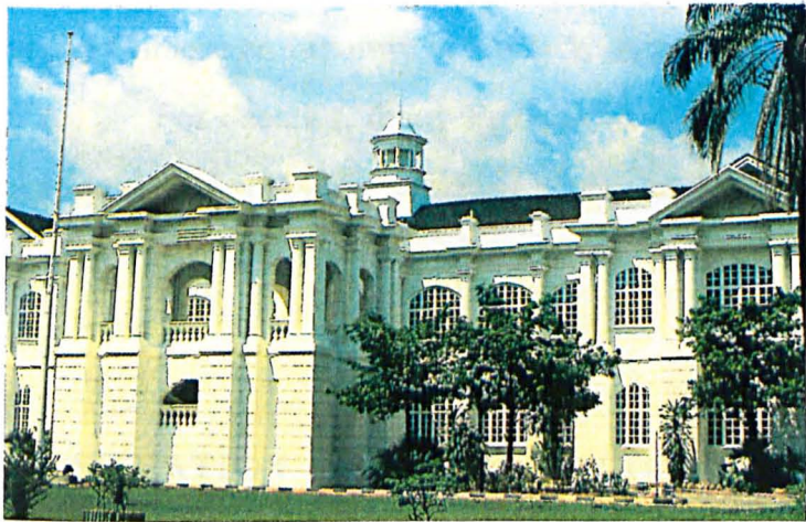
State Library (former State Secretariat building), Seremban (1912)
