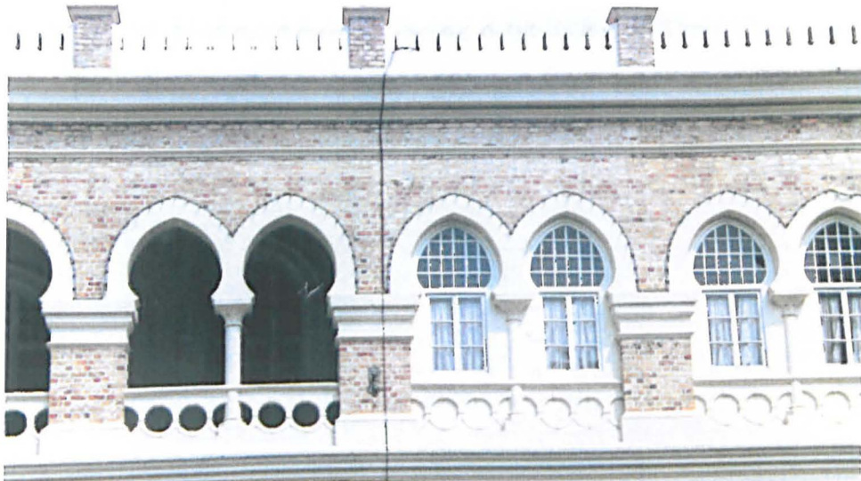
Verandah way was blocked and taken over as waiting area.
