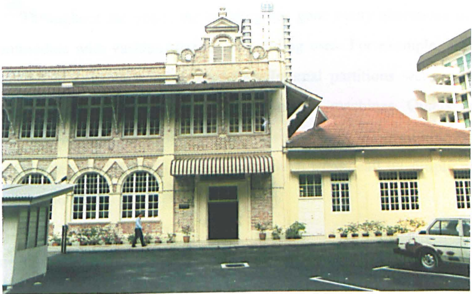
Fig.80 North (above) and west (below) elevations.
