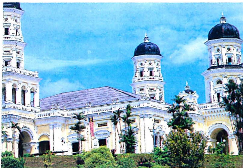
Sultan Abu Bakar Mosque, Johor Bahru (1892)
