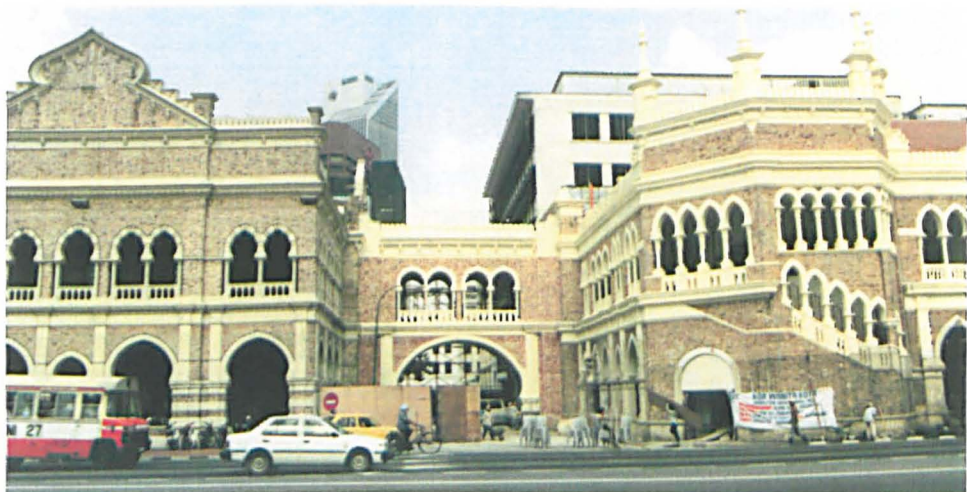
Overhead bridge connecting the building and the Old General Post Office (Right).
