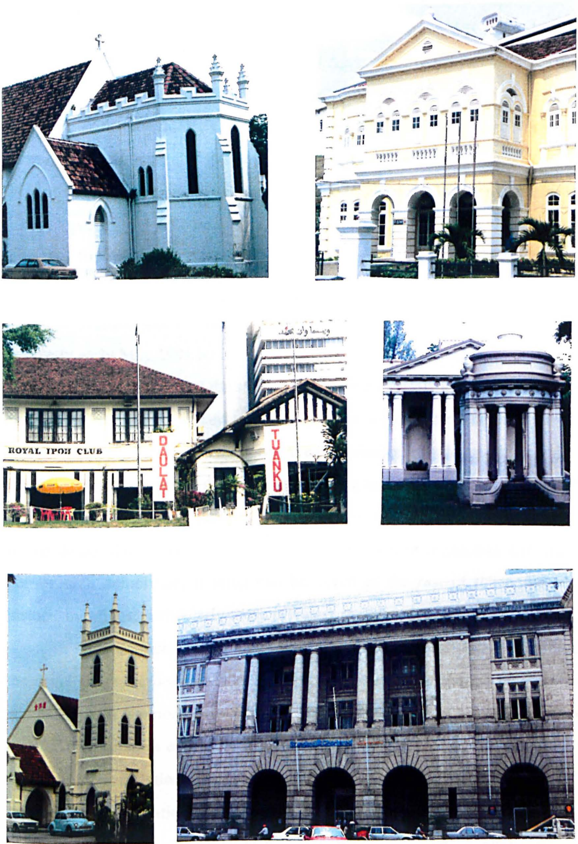
Fig.14 Examples of the privately owned buildings
