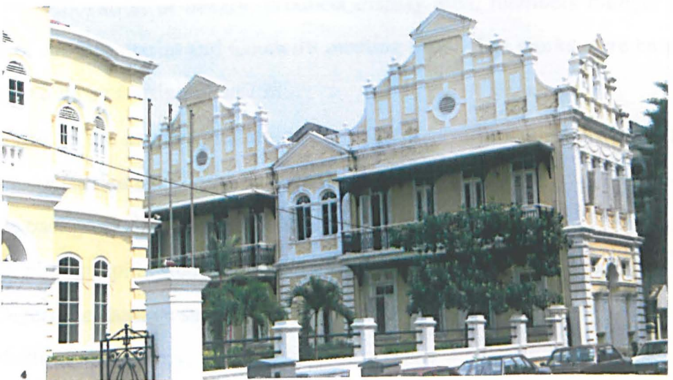
Fig.88 PAM Centre before (above) and after (below) renovation.
