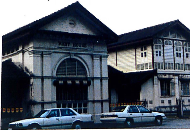
Rest House, Taiping (1894)
