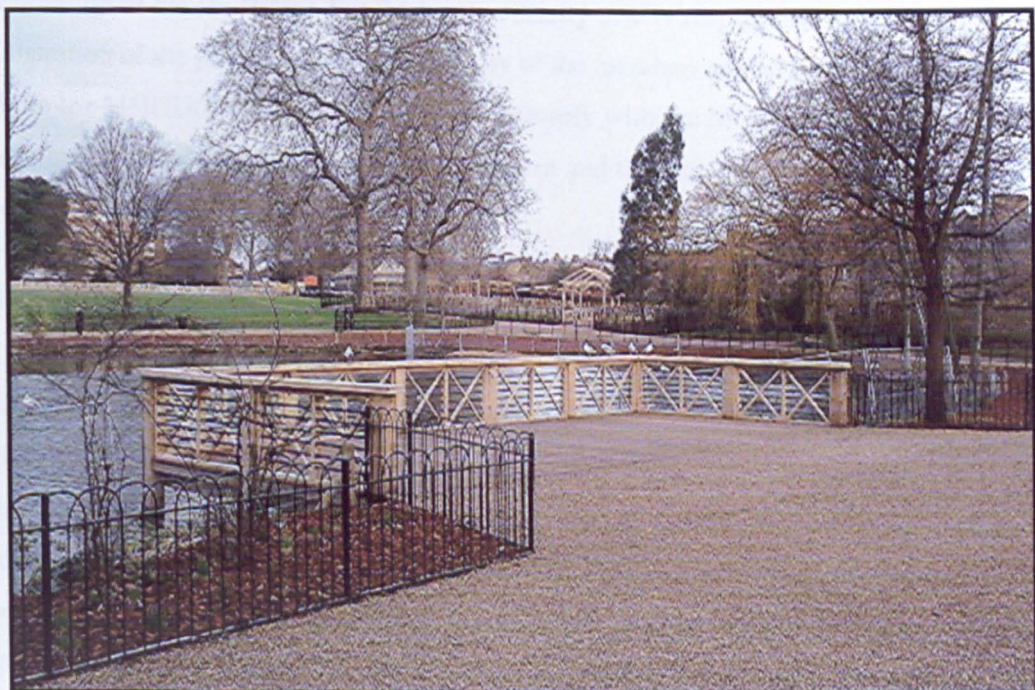
Plate 7.4.3 A new timber deck installed alongside the restored lake, Manor House Gardens
