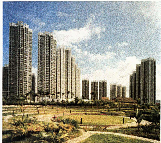
23c. New Housing Estate.
