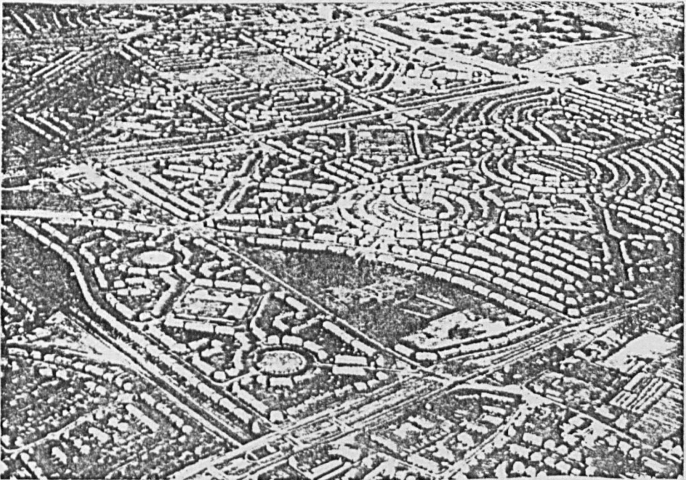
Interwar council estate, Liverpool (Aerofilms)
