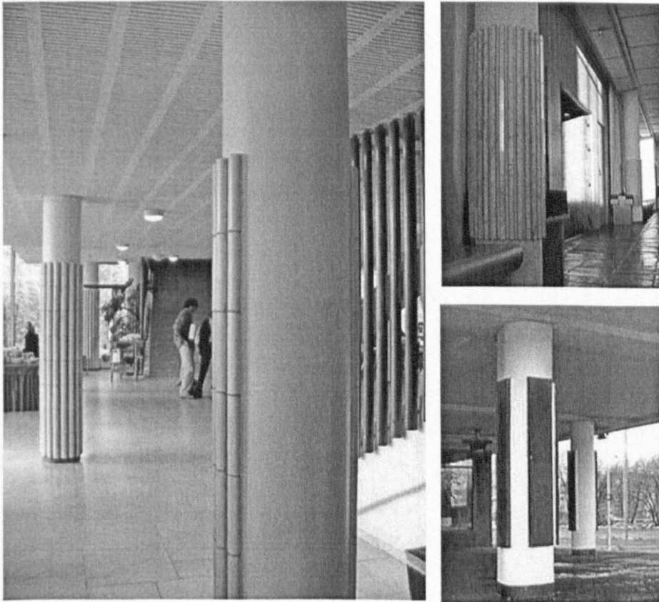
[Fig. 5-73] Different claddings on columns: tile cladding columns in Jyväskylä University, 1950-56 (left), marble slab cladding columns in Seinäjoki Church, 1952-60 (right top) and marble plank cladding columns in Seinäjoki Town Hall, 1961-65 (right bottom)
