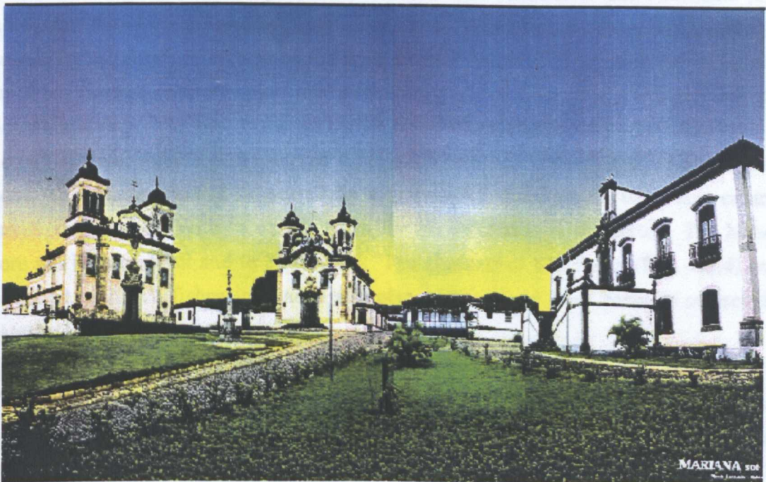
Fig. 4. 5. 3 - the three expressive buildings enclosing one of the only two surviving pillories in the whole of the country (photo by Eustaquio, M.-Itafoto)
