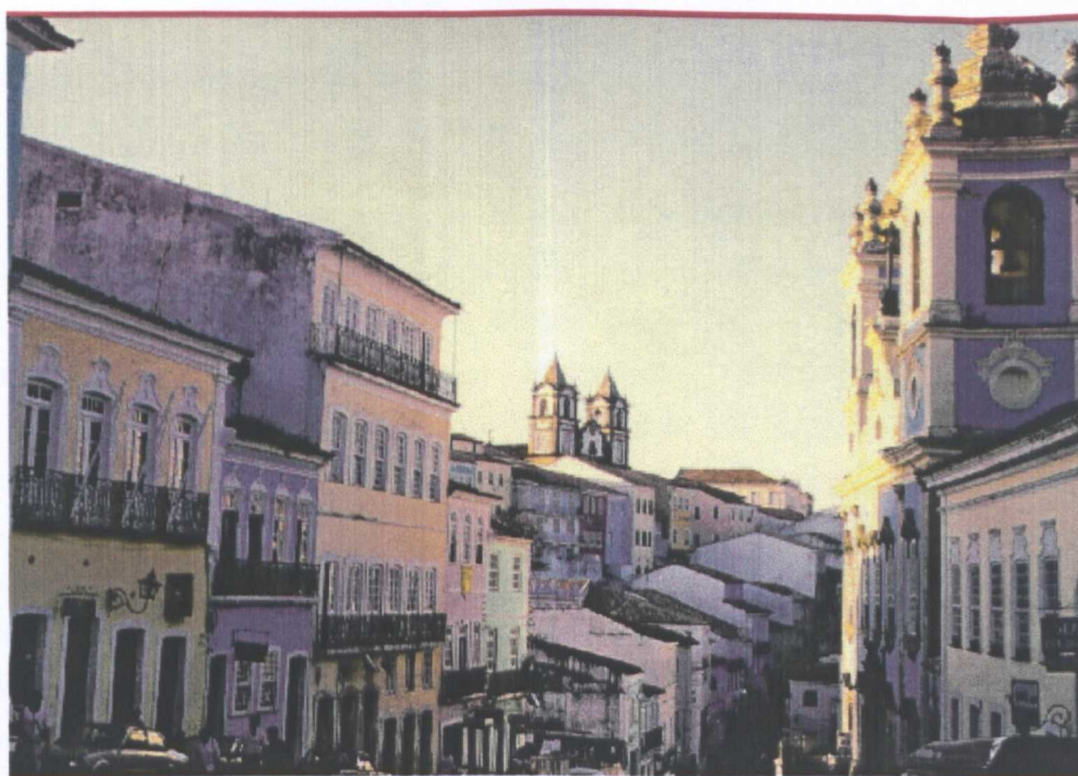
Fig. 1.2.22- the recent restoration of the Pelourinho, in Salvador
