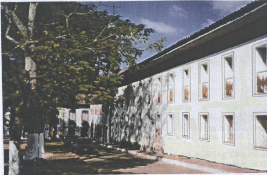
Fig. 6.1.12- the archbishop's house was built in 1989, in Gomes Freire Square
