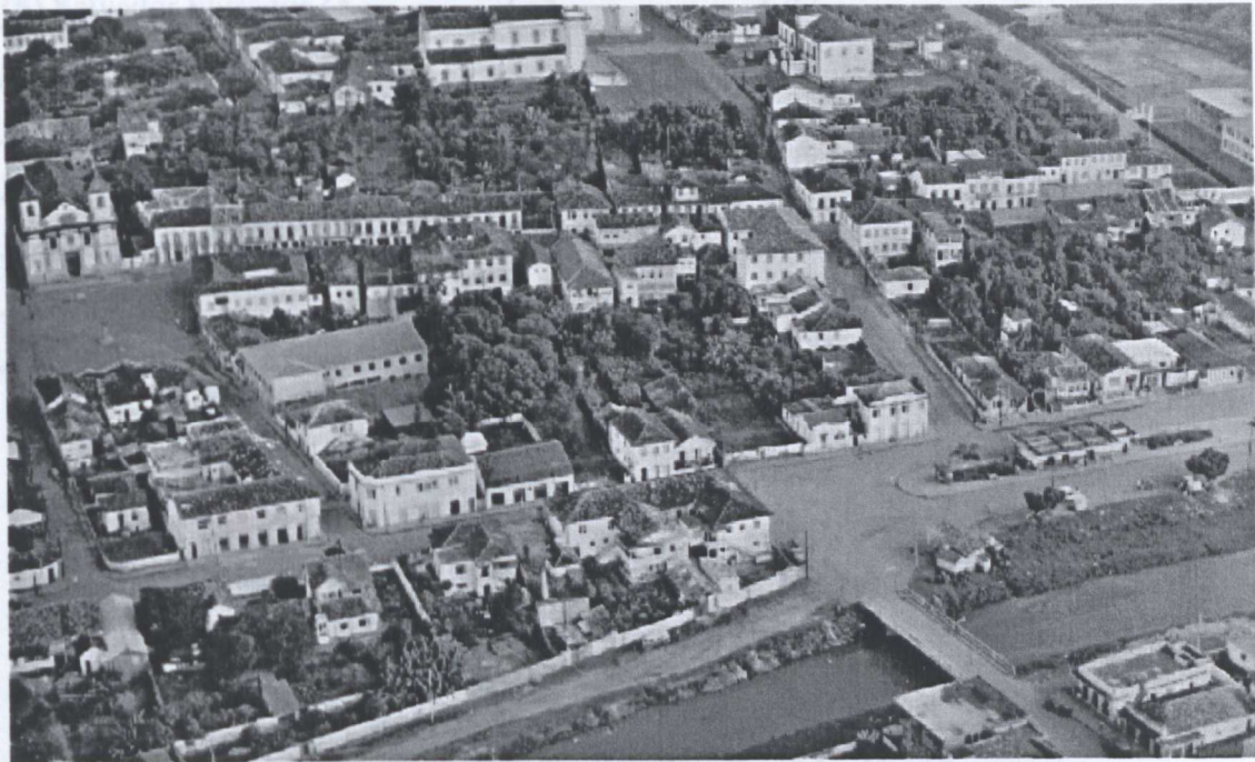
Fig. 7.1.4 - this aerial photo shows the River Bank area
