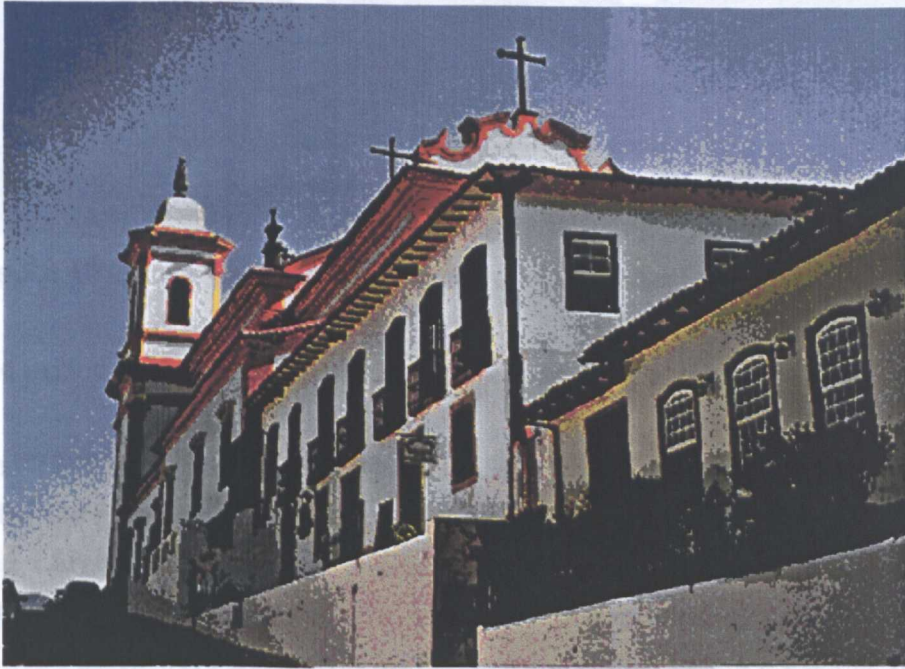
Fig. 5.4.9 - the building situated behind São Francisco Church is known as the Palace of Assumar
