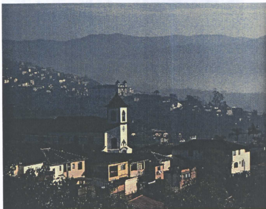
Fig. 5.3.15 -Church of Nossa Senhora dos Anjos or 'Capela da Arquiconfraria' of wood including the roof, floors, ceilings, retables, windows, doors, etc. The handrail is also This church structure is a mix of stone foundation externally supporting stone walls and internally with walls of the large bricks of mud mixed with straw called 'adobe' framed by wooden beams and pillars. Disinfested against termites. Glass needs to be replaced in window frames.
