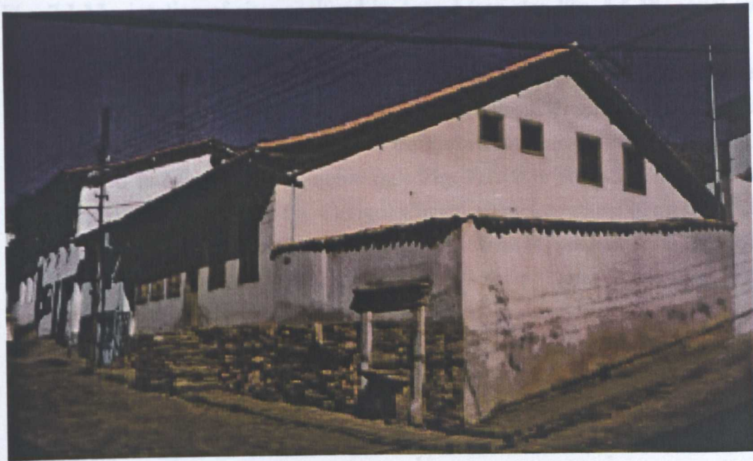
Fig. 7.1.12 - the house shown in photograph above after it had been rebuilt (July 1996)
