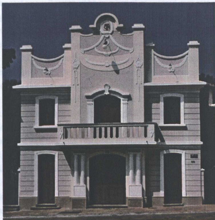
Fig. 6.1.7 - Theatre front facade: the work of restoration was carried out from 1989 to 1991.
