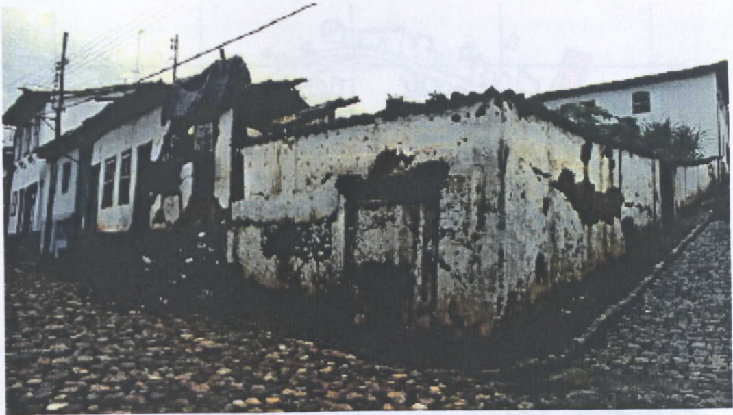
Fig. 7.1.11 - a private building in Barão de Camargos street in January 1991
