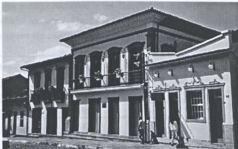
Fig. 6.1.6 - the latest version of the art-deco house (at its left the restored 'Casa de Cultura' which was the old Intendencia building)
