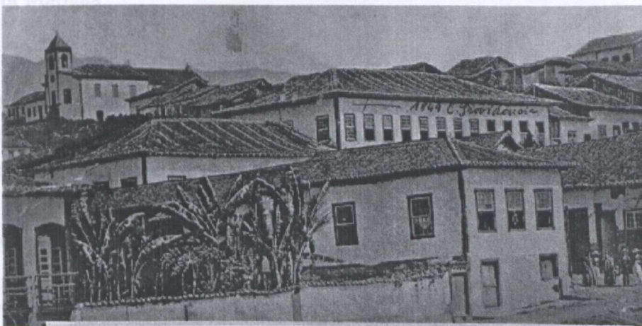
Fig. 5.4.23- The house at the right disappeared after being ruined in the 1960s and the one at the left was demolished. Both were replaced by the Archbishops' Palace
