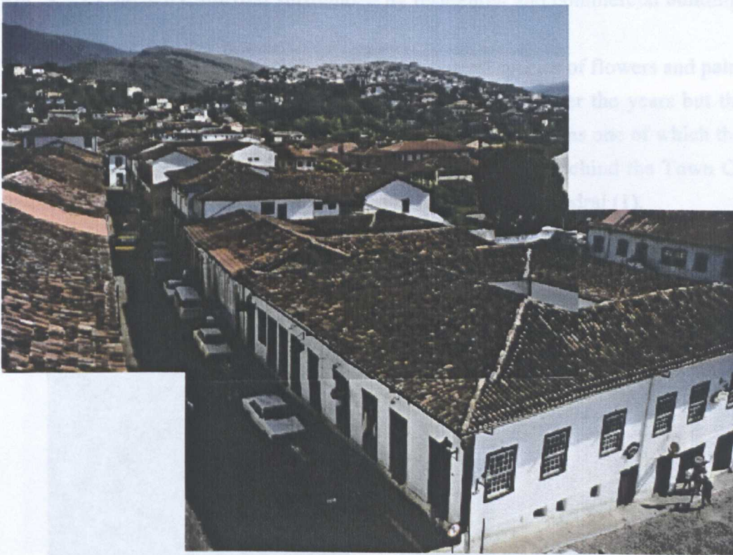
Fig. 5.5.6 - Barão do Pontal's house is the highest roof in the centre of the photograph
