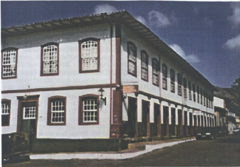
Fig. 6.1.10 - the building of the Central Hotel in 1996 - Grid F7
