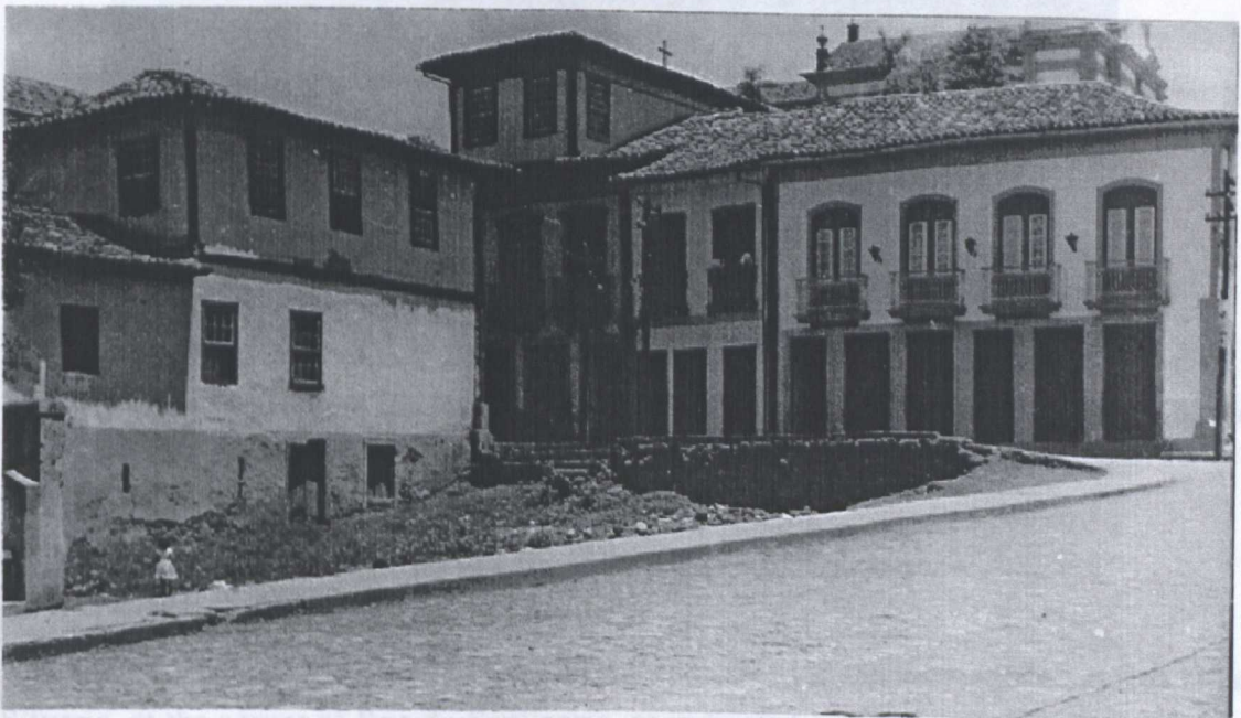
Fig. 5.4.21 - a private property was demolished at the corner of the 'Rua Direita' with 'Josafá Macedo' (Grid D 9)
