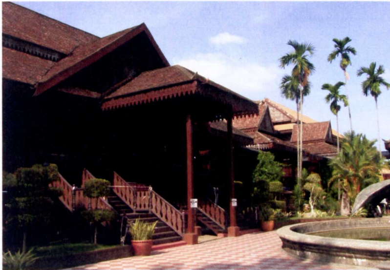
Figure 5.13. The main building of the gallery and museum. Source: photo by the author.
