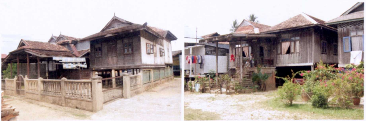
Figure 7.8. Some of the traditional timber Kelantan Malay houses that are still occupied in the rural settlement area. Normally the house is not painted and left as natural timber colour. Source: photos by the author.
