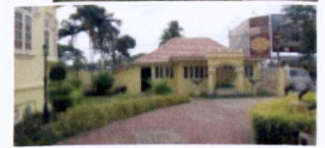
The location of the public toilet at the main entrance. Previously it was used as a guard house.
