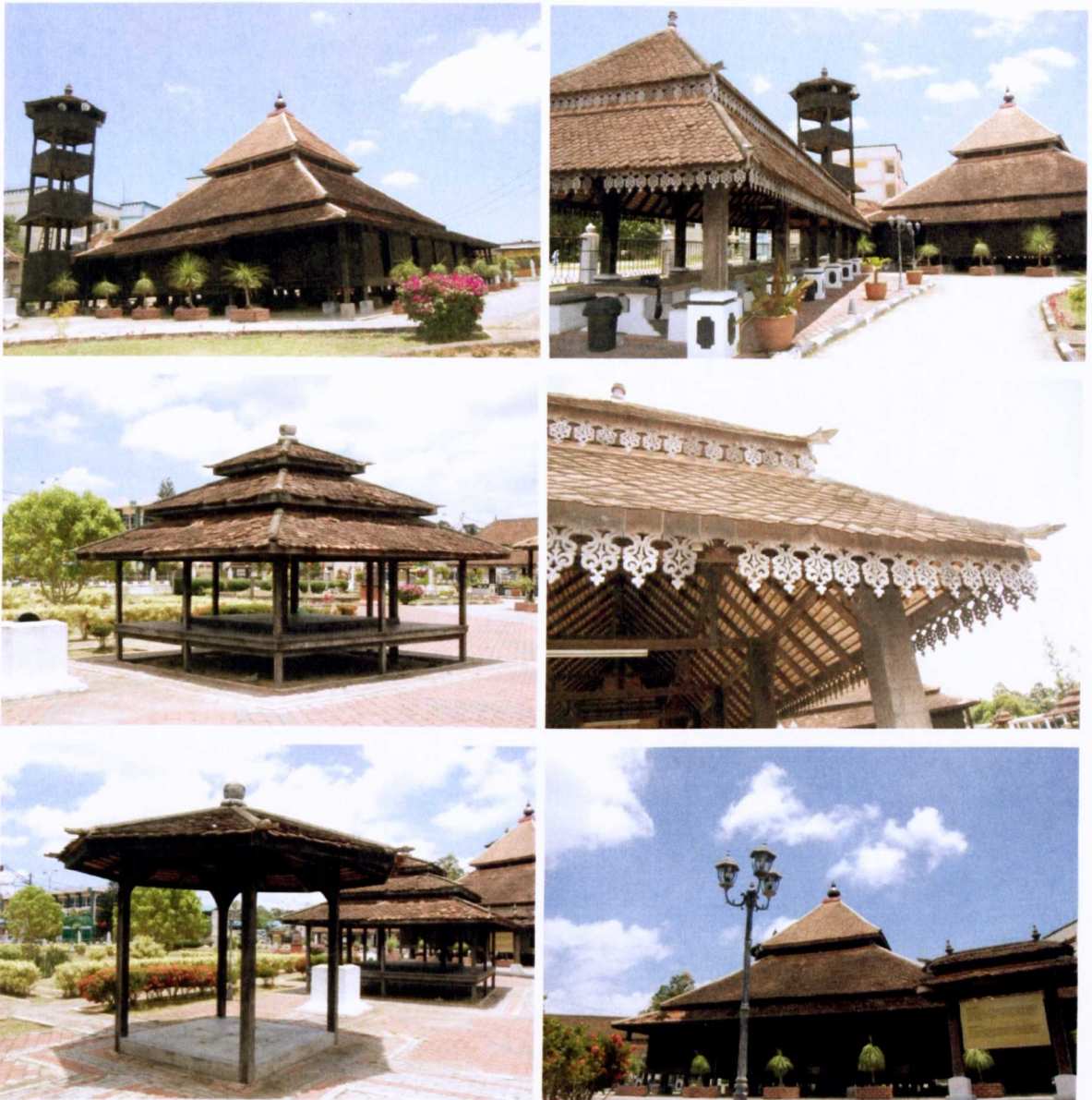
Figure 7.6. Kampung Laut Mosque is well-known as one of the earliest mosques in Kelantan which has been constructed according to the authentic Kelantan Malay vernacular architecture design. The location has been removed to Nilam Puri, Kota Bharu but still remains for performing prayer. The original location was based on Kampung Laut, 32 km away from the current location. Source: photos by the author.
