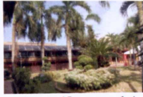
The use of Perspex roof at the food court
