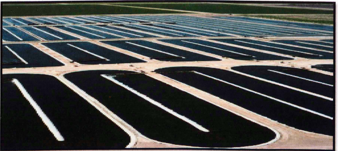
Figure 1.15. Raceway Ponds used for the culture of Spirulina platensis by Earthrise Farms in Calipatria, California (Courtesy A. Belay) ( http://www.scieng.murdoch.edu.au/centres/algae/BEAM-Net/BEAM-App14a.htm ).
