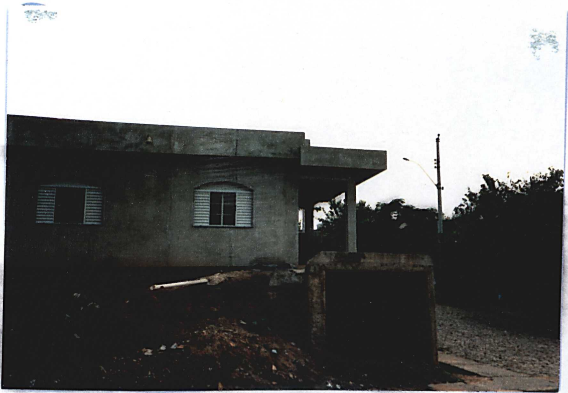
FIG. 8.16 Total modification of a threebedroomed house.
