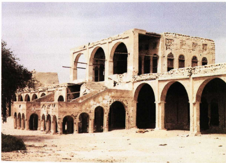
Figure 3.18: An Example of Traditional Buildings in Al-Hufuf (Source: King, 1998)
