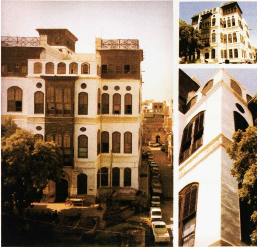
Figure 3.25: Nasif House in Jeddah (Source: Buchan, 1991)
