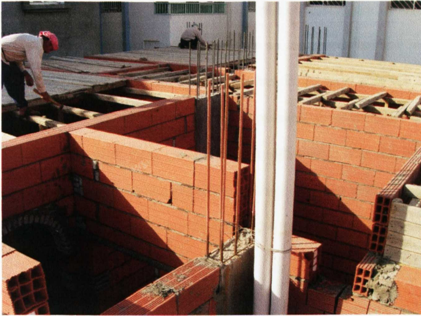
Figure 3.34: A Residential Building under Construction in Saudi Arabia (Source: Author)
