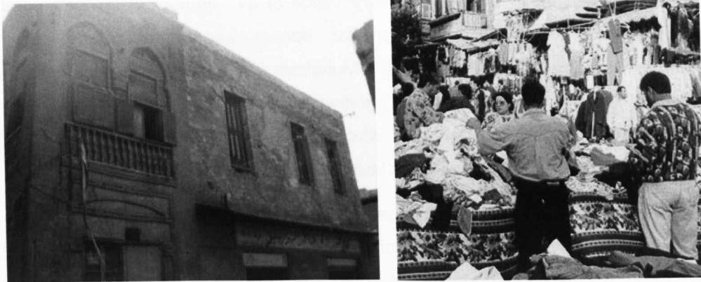
Figure 7.13 Problems of deterioration and unsuitable land use in Bulaq.
