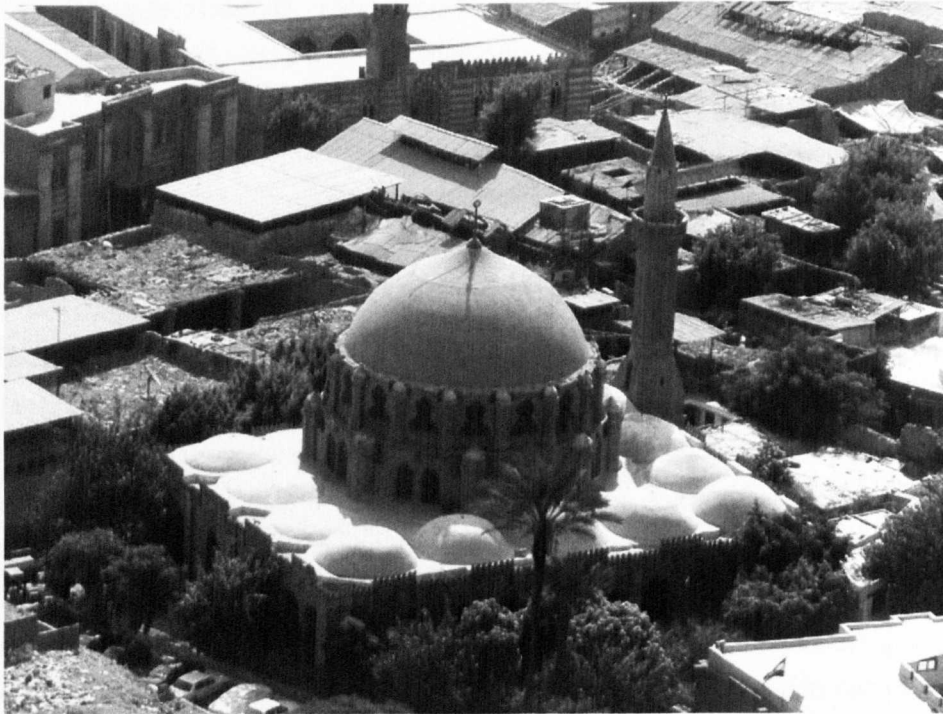
Figure 6.4 The site of the historical Sinan Pasha mosque. The mosque was surrounded by old workshops and warehouses which were subject to demolition.
