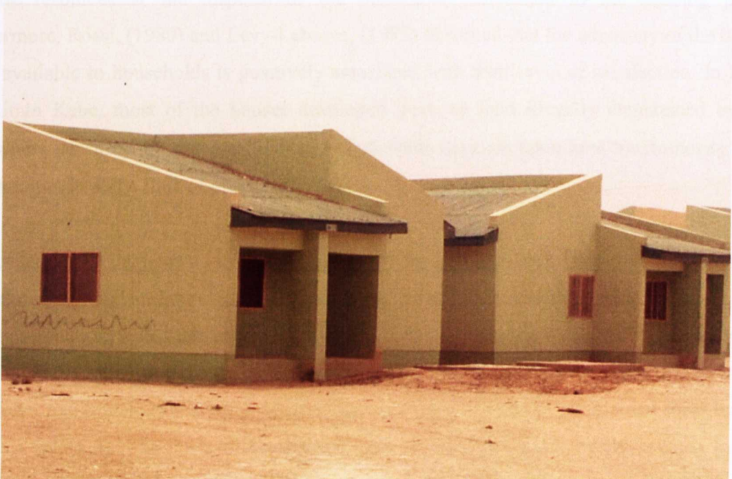
Plate 2: Residential Apartments in Danladi Nasidi Housing Estate
