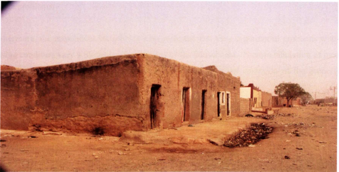
Plate 3: Residential Apartments in Rimin Kebe (Notice the traditional settings of houses).
