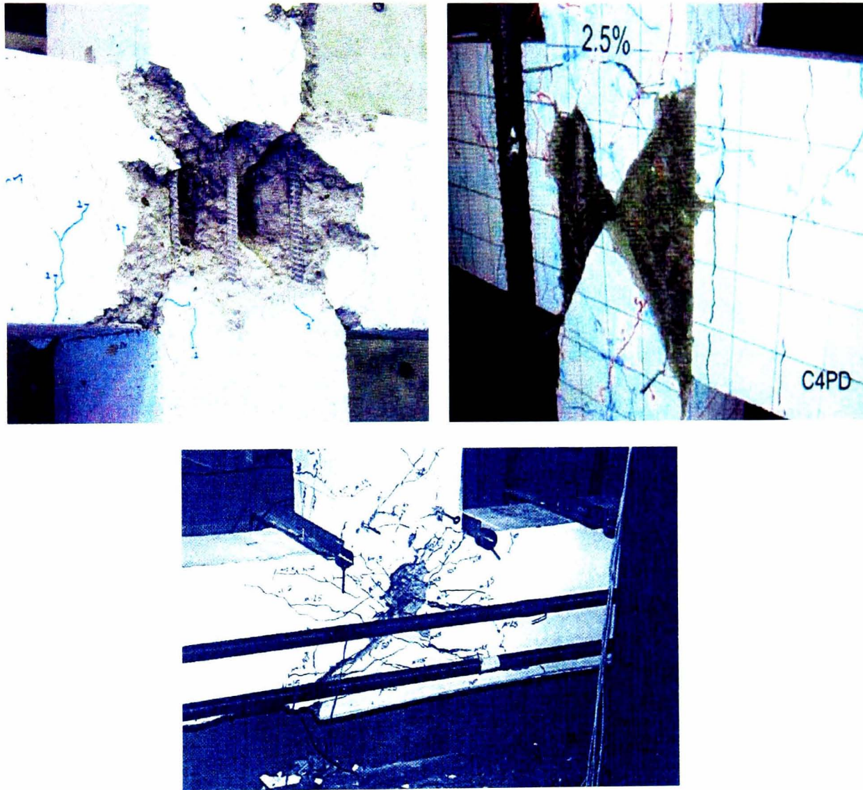
Figure 2.7. Shear failures in joints (Pagni, 2004, Dhakal, 2005 and Pantelides 2000)
