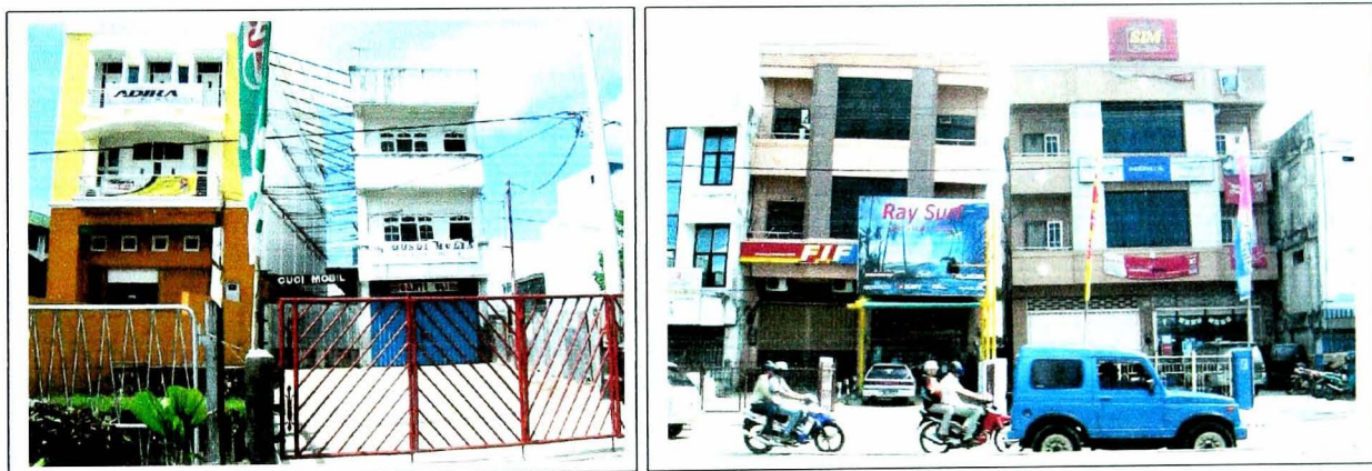
Figure 1.1: Tilting buildings in Banjarmasin City (Indonesia)
