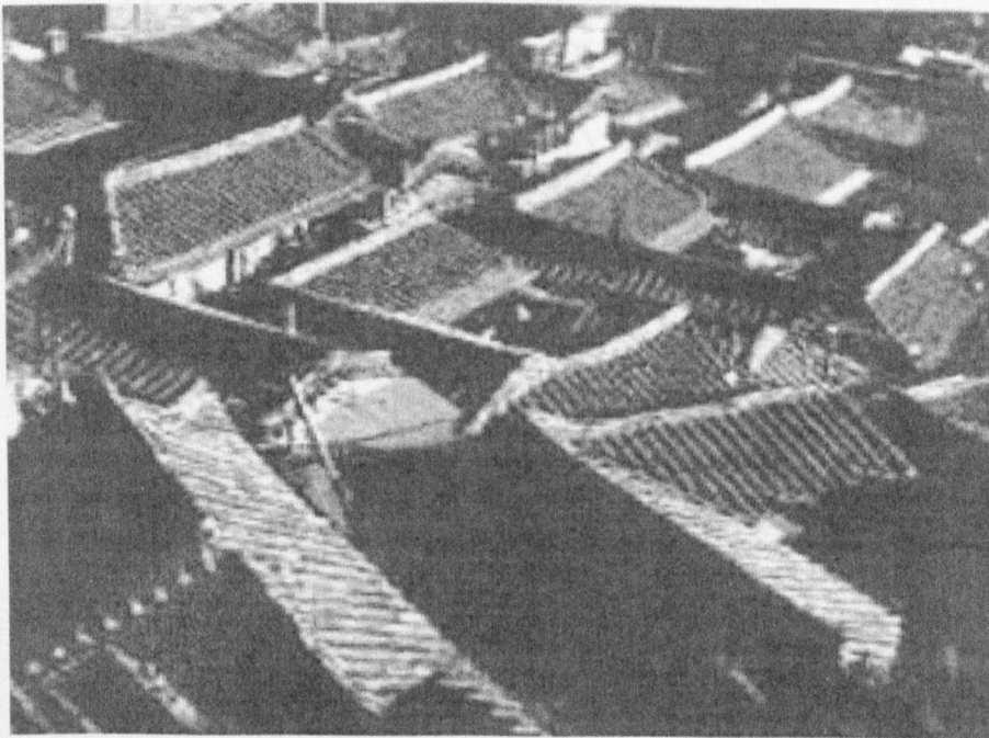
Figure 2-12. Typical view of the semi-enclosed courtyard house of an urban area built during 1930-60
