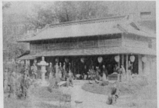
[Figure 9-2] A Double-Eaves of Japanese Tea House (at the Columbia Exhibition held in Chicago in 1893)
