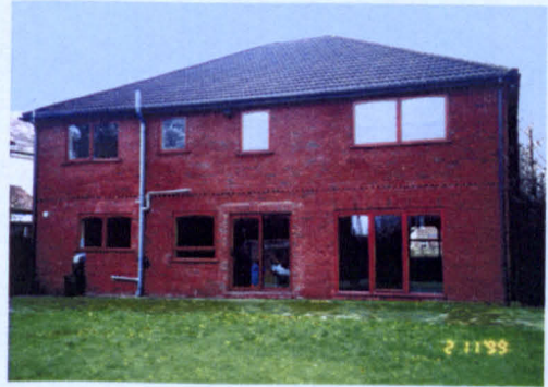
(B) The rear view of: the northeast side.
