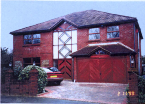
(A) The front view: the southwest side.
