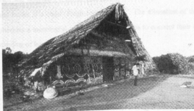
Figure 7- 8 Front view of the Tukanoan longhouse.
