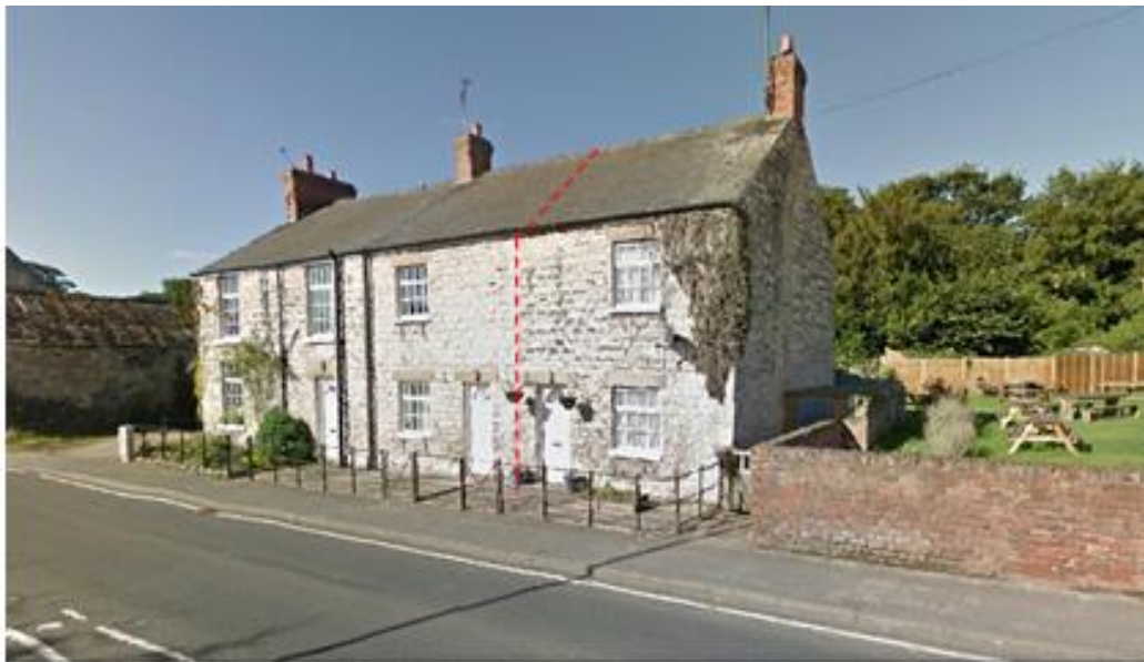
Figure 3.4 External elevation of the manually controlled building (Google, 2015).
