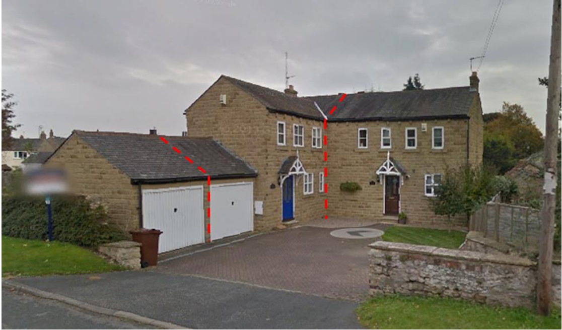
Figure 3.18 External elevation of the temperature controlled building with demarcation line for adjacent building (Google, 2015).
