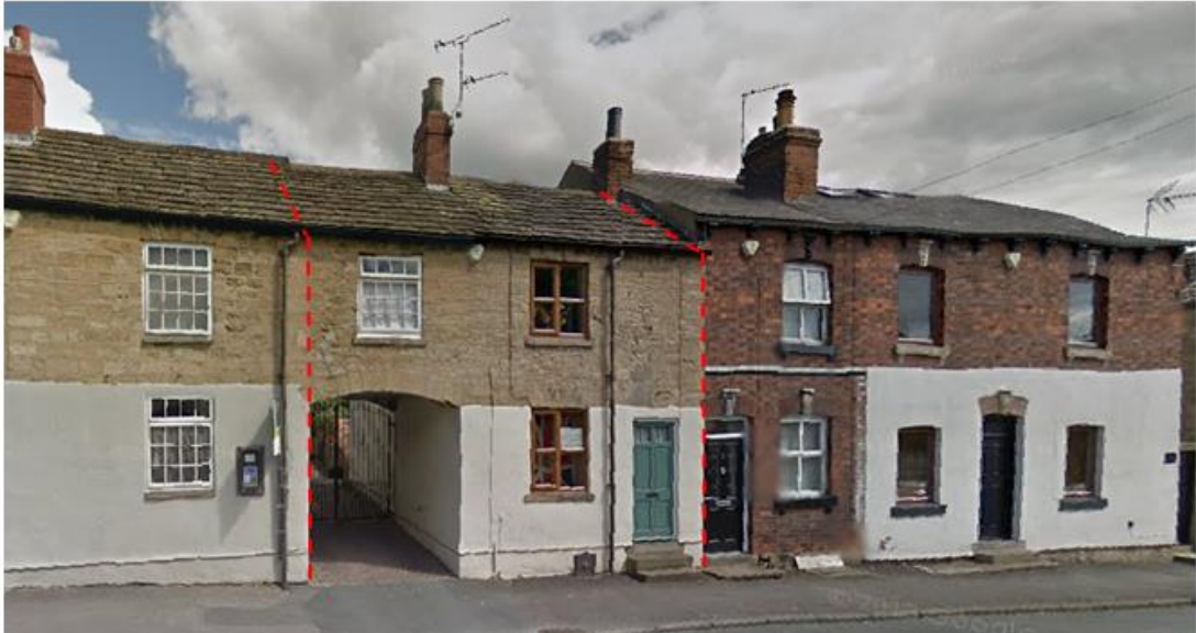
Figure 3.11 External elevation of the timed controlled building (Google, 2015).
