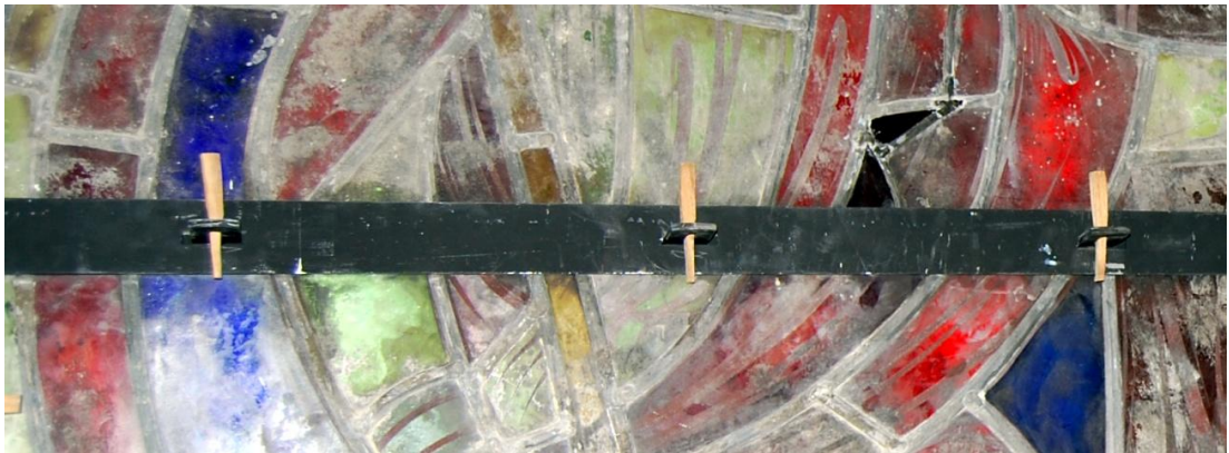
Fig. 14, Chartres Cathedral, lug-bar with wedges.
