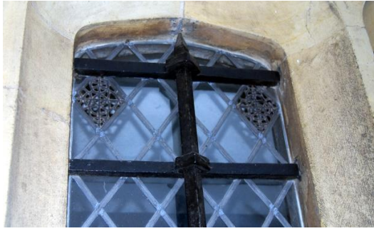
Fig. 10, Hampton Court. Ferramenta in situ. Details of the ferramenta with through bar.
