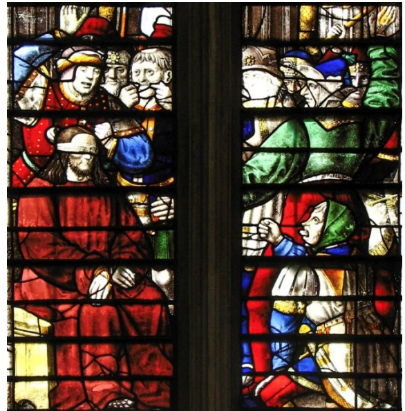
Fig. 11, King's College, Cambridge, ferramenta with double stanchions.
