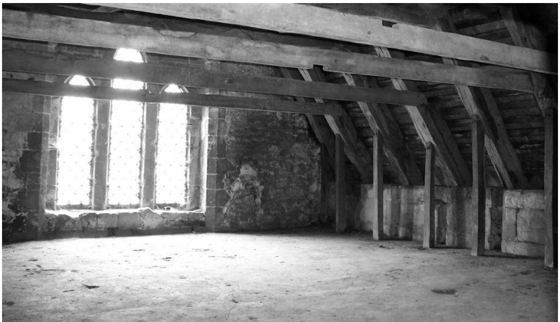
Fig. 16, York Minster, interior view of the tracing room.
