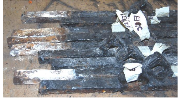
Fig. 10, Hampton Court. Ferramenta in situ. Details of the ferramenta with through bar.
