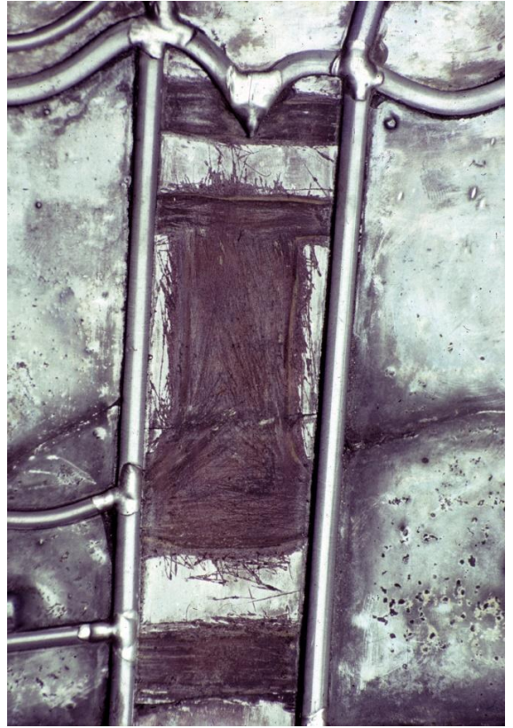
Fig. 52, Fairford NIV light b, a persecutor of the faith and detail from the scabbard. Inside in transmitted light and outside showing the free hand abrasion.
