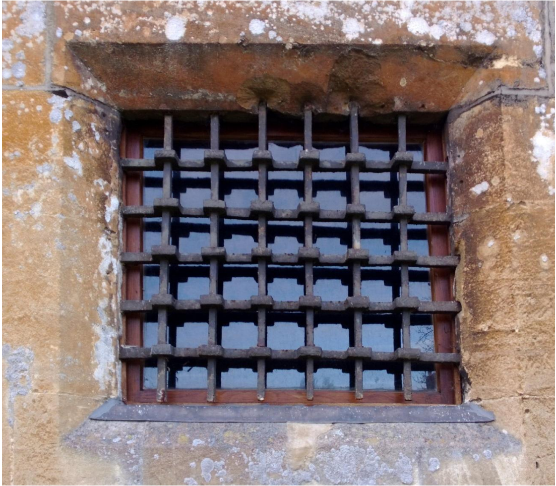
Fig. 13, Fairford, ferramenta on vestry window.
