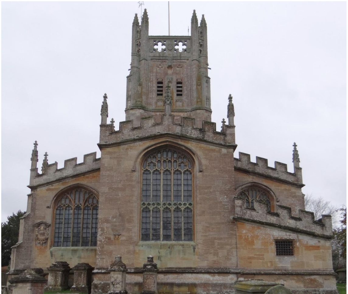
Fig. 5, Fairford, East elevation, external ferramenta support systems.
