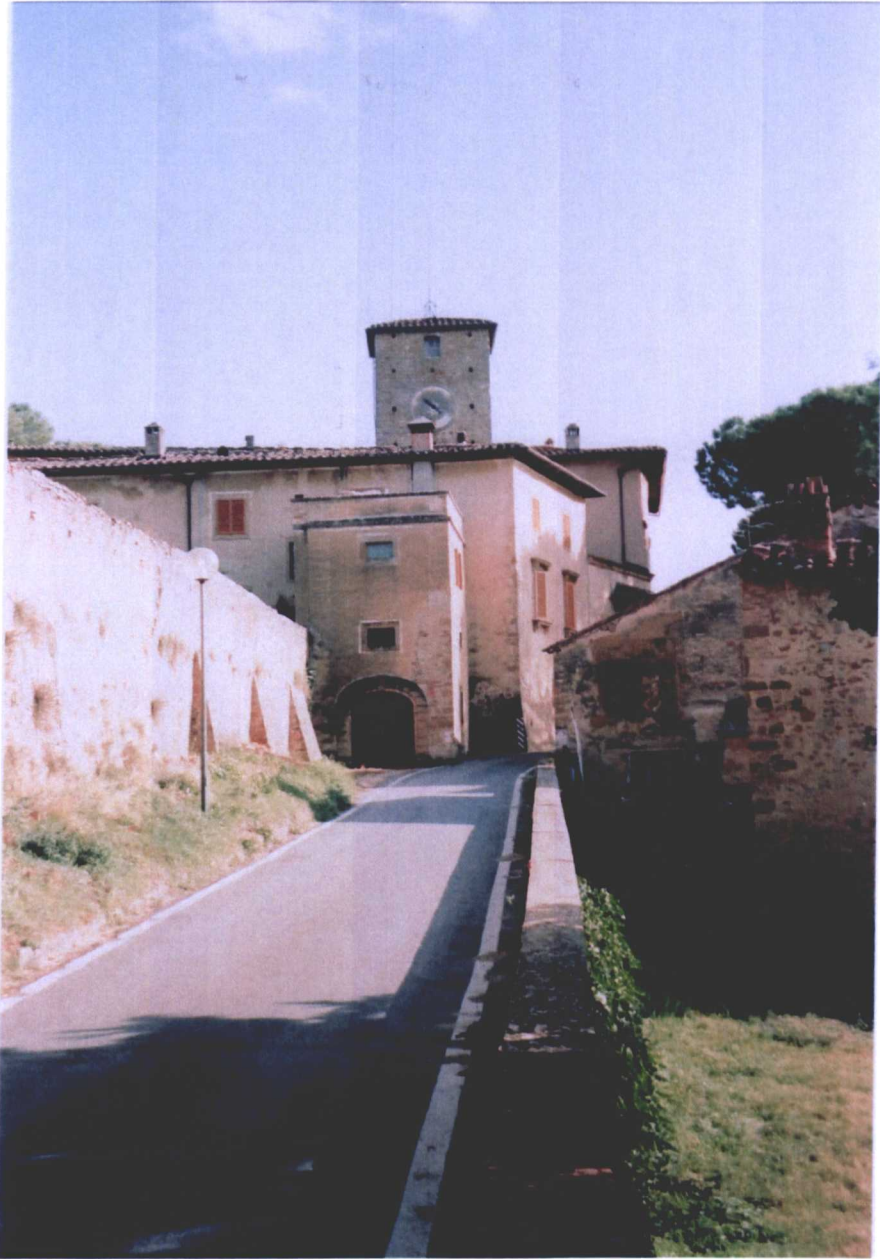
Figure 5.35 Villa compound of Petrognano; view facing south-east showing clock tower.
