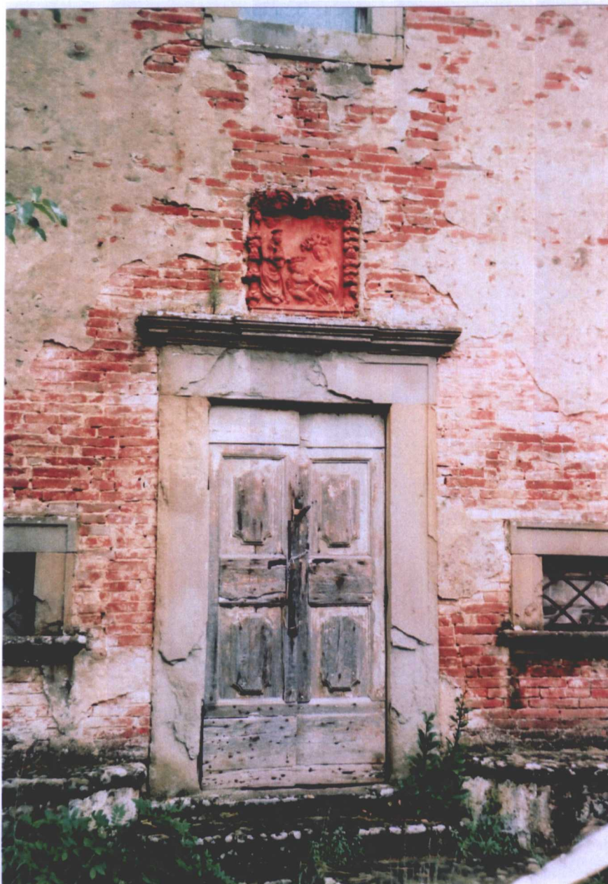
Figure 5.34 Exterior of early seventeenth-century chapel of the Annunciation at the Capponi estate of Petrognano, in Barberino, Val d'Elsa. The chapel is located within the walls of the villa estate to the north-west.
