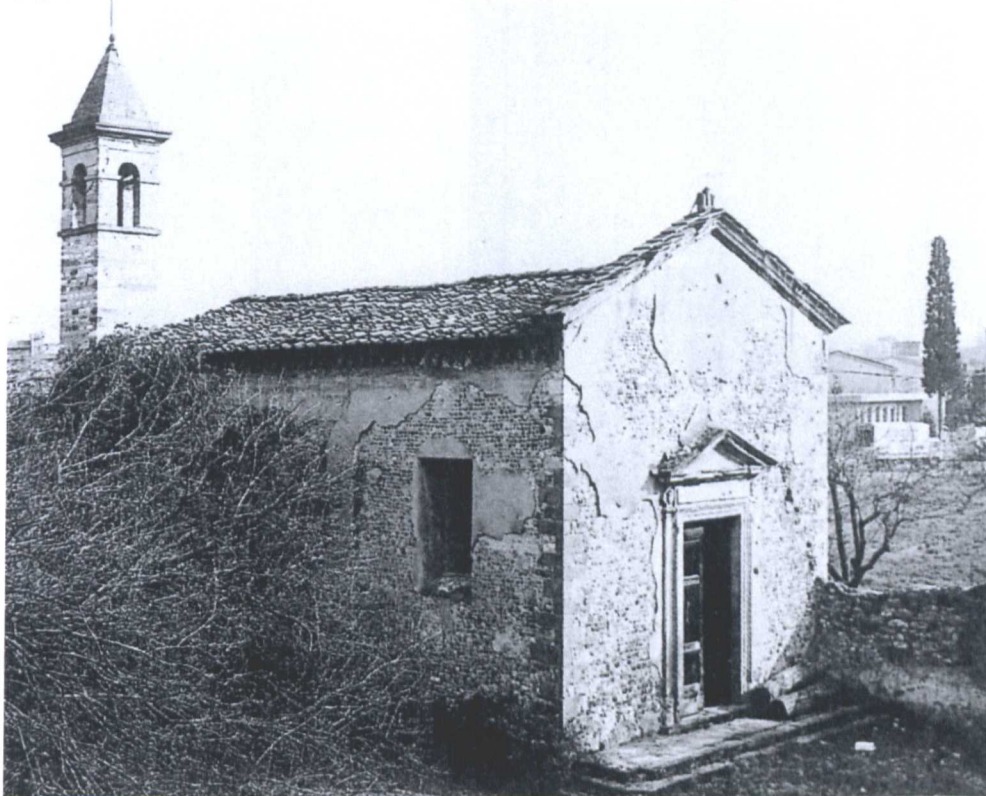
Figure 5.57 Villa Spini, chapel, exterior (reproduced from Mannini 1994).
