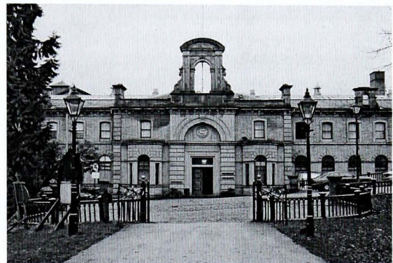
Plate 122 Principal facade of office block, Saltaire Mills, Saltaire
