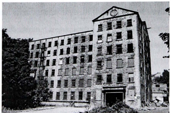
Plate 126 South elevation of Old Lane Mill, Northowram, facing the town of Halifax
