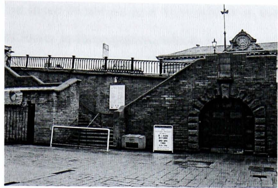
Plate 90 There was direct access from the mill yard at Saltaire Mills, Saltaire, to the mill canteen via the tunnel on the right
