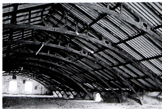
Plate 59 Attic space at Old Lane Mill, Northowram
