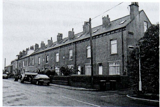
Plate 92 Workers' housing built by Thomas Ambler & Sons, adjacent to their mill, Ardsley Mills, East Ardsley
