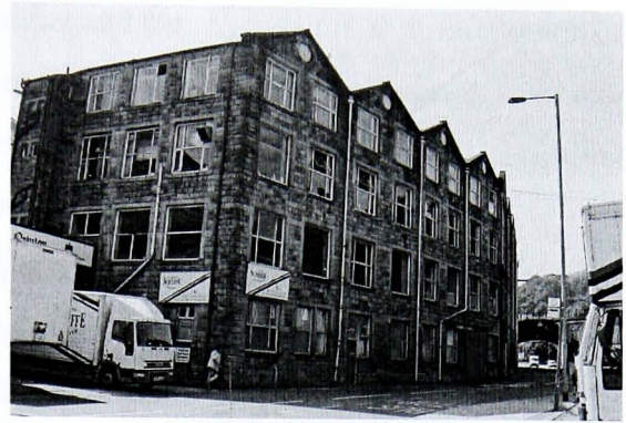
Plate 124 North elevation of Frostholve Mill, Cornholme
