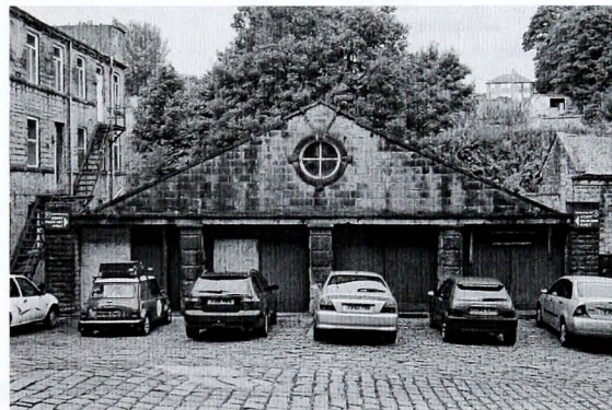
Plate 37 At Ebor Mill, Haworth, the detached boiler house was located away from the engine house to take advantage of easy access from the mill yard
