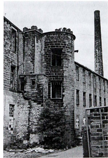
Plate 80 Projecting staircase tower added to Aireworth Mills, Keighley in the mid-19th century
