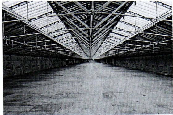
Plate 120 The vast attic floor, Saltaire Mills, Saltaire
