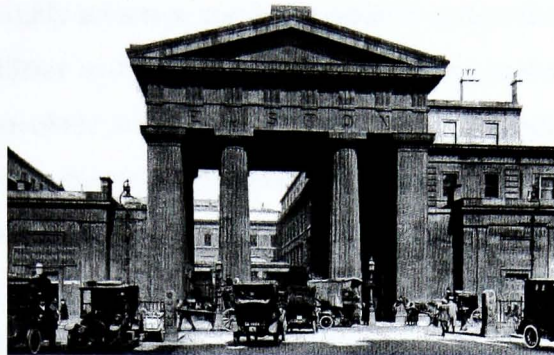
Plate 2 The demolition of the Euston Railway Arch in 1962 aroused widespread interest in industrial monuments (Buchanan 2000, 18)
