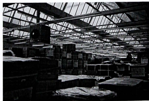
Plate 54 The superstructure of Park View Mills, North Bierley was not designed to support a system of power transmission as the site was built to be electric powered
