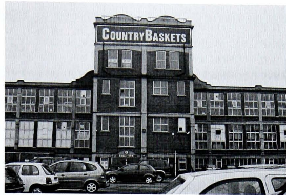
Plate 63 The tower at Ardsley Mills, East Ardsley housed privies, offices, a hoist and the main staircase for the mill
