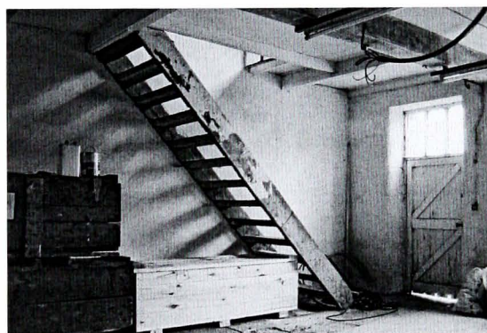
Plate 84 Open internal staircase, Dunkirk Mill, Oxenhope
