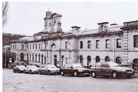
Plate 94 Attached office block fronting Victoria Roads at Saltaire Mills, Saltaire
