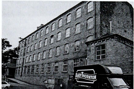
Plate 102 Victoria Mills, Elland, is built of local sandstone with red-brick dressings
