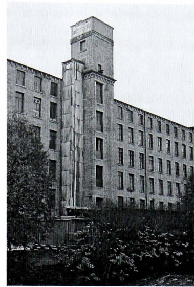
Plate 79 Projecting staircase tower, Britannia Mill, Lockwood
