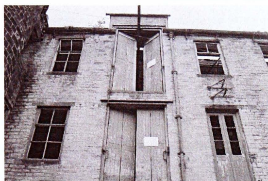
Plate 69 Inserted hoist and taking-in doors, Aireworth Mill, Keighley
