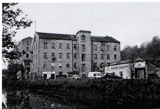
Plate 66 The projecting staircase tower at Firth's Mill, Lockwood, incorporated taking-in doors at each floor level
