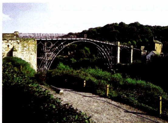
Plate 1 Major monuments like the Iron Bridge, Coalbrookdale, were the first to attract the attention of the industrial preservation movement (English Heritage 2003)
