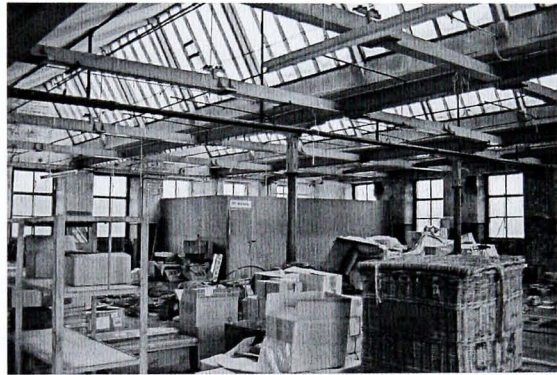
Plate 61 North-lit top storey, 'New Mill, Ebor Mill, Haworth
