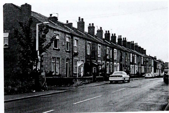
Plate 129 Workers' housing to the north of Ardsley Mills, East Ardsley
