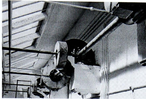
Plate 47 Principal horizontal shaft at rear of weaving shed, Queen Street Mill, Burnley
