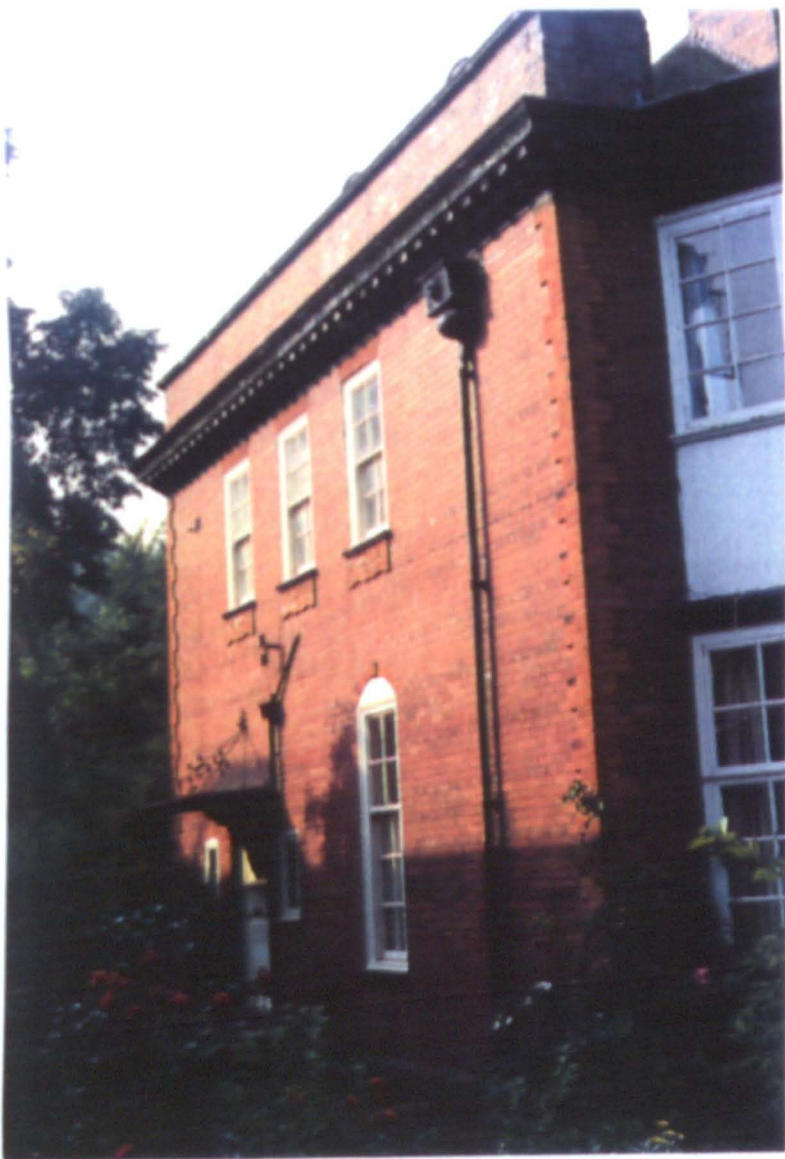
4.46 Main (side) entrance.
