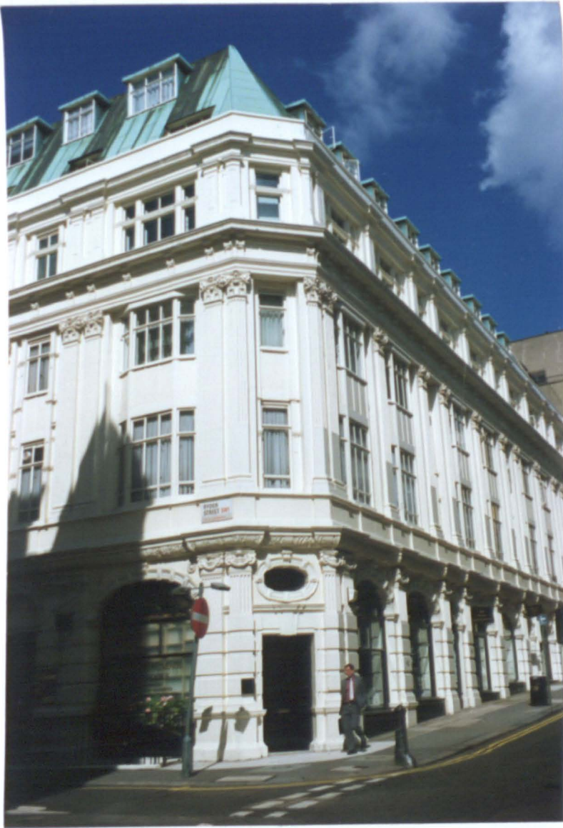
5.1 Corner of Ryder and Duke Street, St. James's in 1992, the block in which C.A. Hunt's apartment and the Carfax Gallery were situated.
