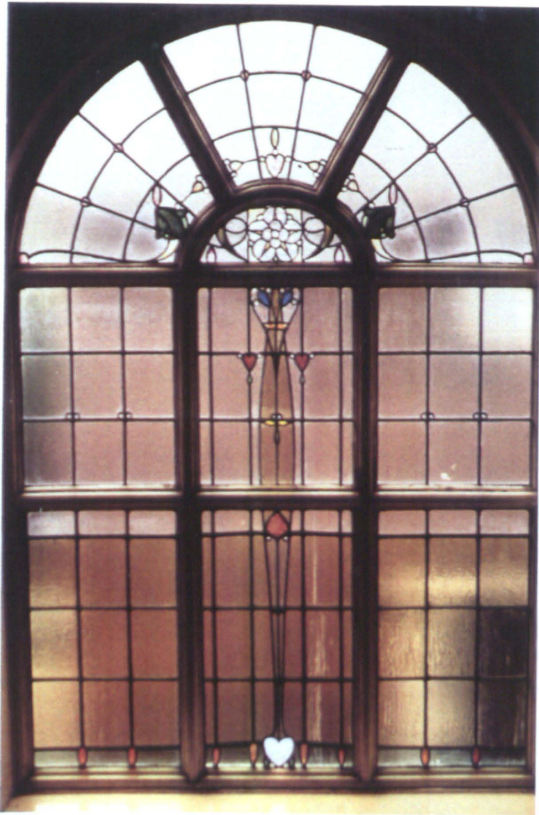
4.90 Staircase window by George Walton, in 1991.
