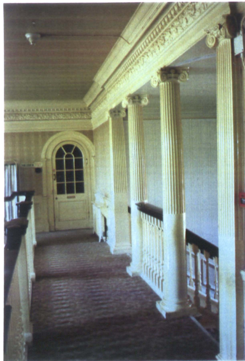
4.83 Landing and hall gallery to bedroom suites in 1991.
