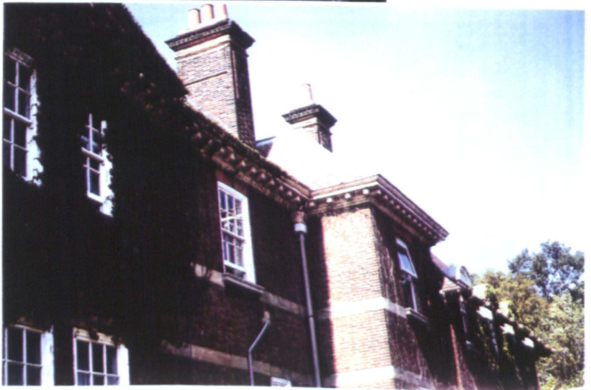
4.95 Cornice and fenestration of east front in 1991.
