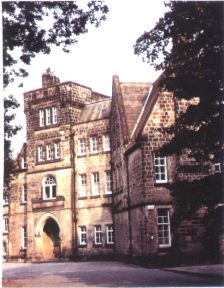
4.129 Entrance front with extension to right in 1992.
