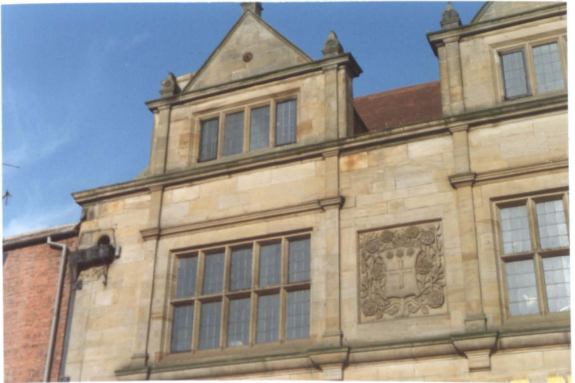
4.114 The Yorkshire Bank, Thirsk, armoial panel and gables.
