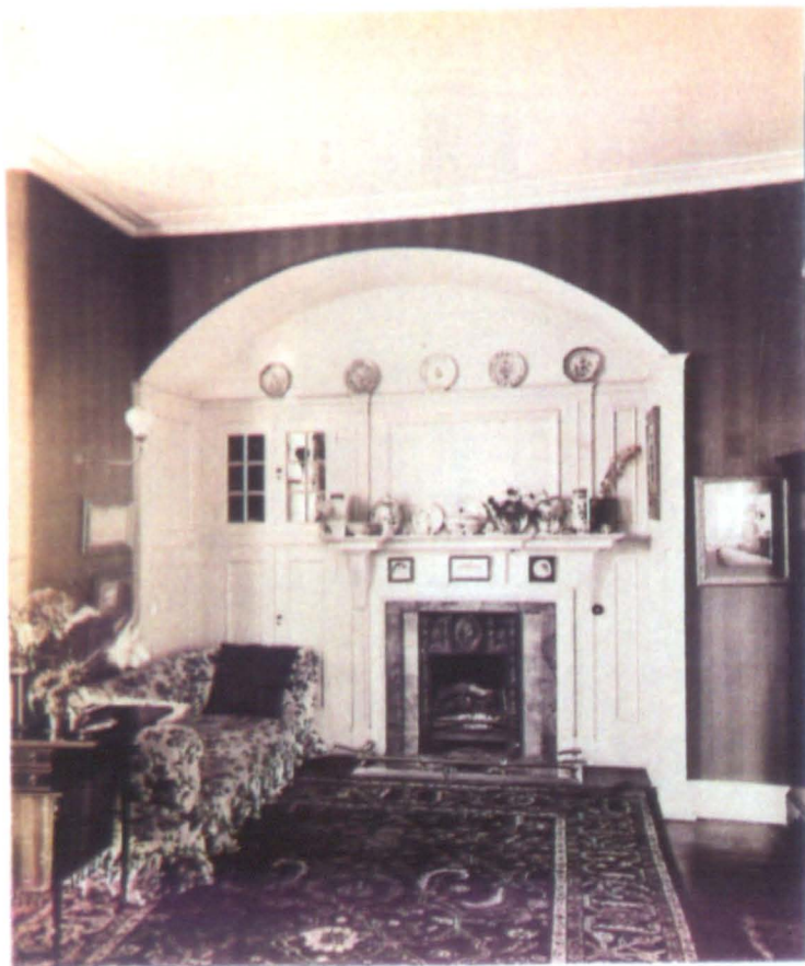
4.64 Inglenook in c.1900 (Photo at K and P ).
