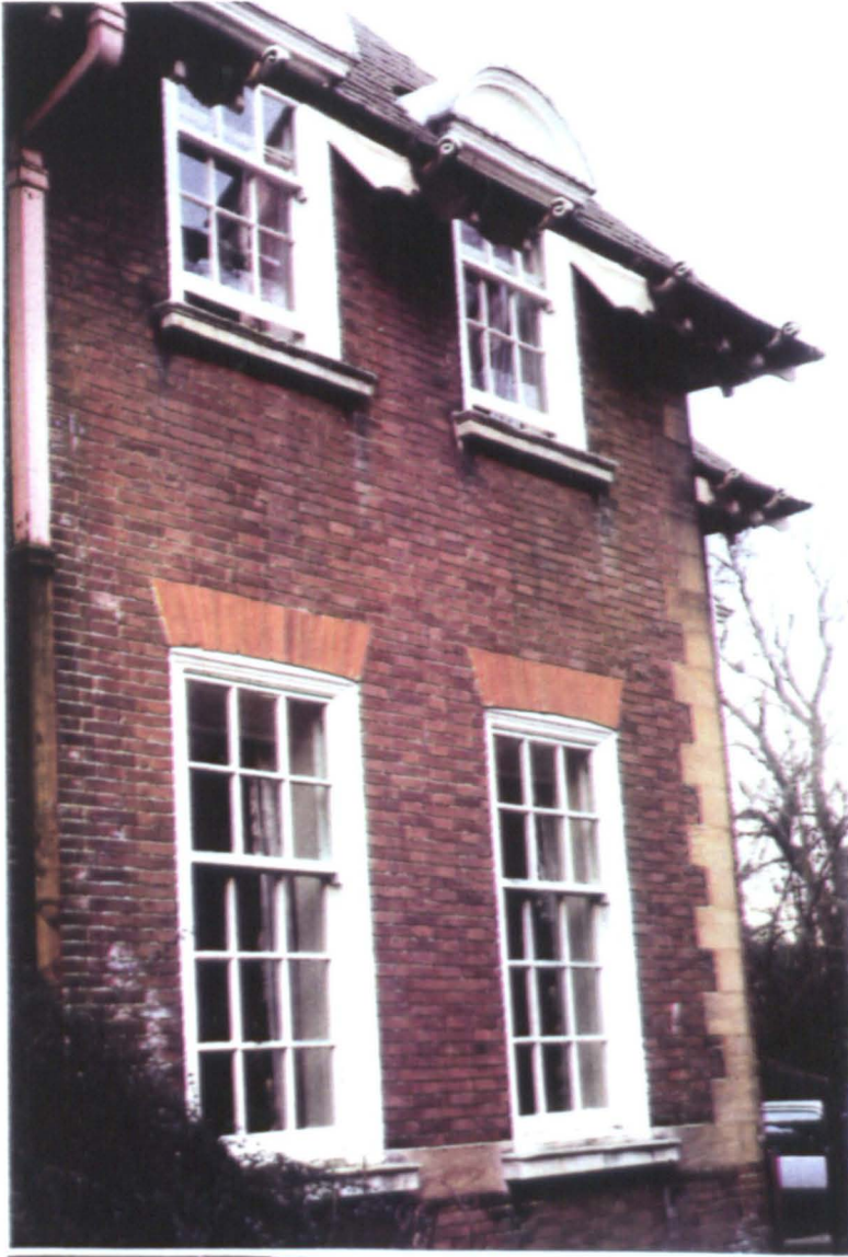
4.94 Fenestration and guttering of service wing on east front in 1991.
