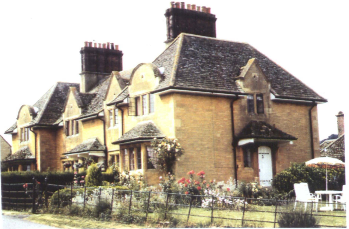
4.148 Four stone cottages (termed The Palaces by Eyres-Monsell) (1903) by B and K , in 1994.
