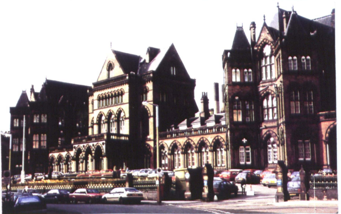
2.2 Leeds General Infirmary (1862-1868) by Sir George Gilbert Scott; administration block and wards in 1992.
