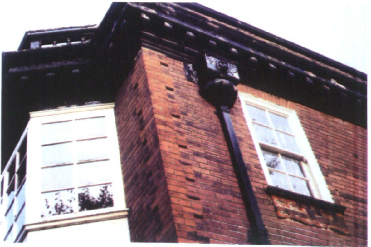
4.45 No.3 Shireoak Road, Bay window, quoins and cornice with balustrade.
