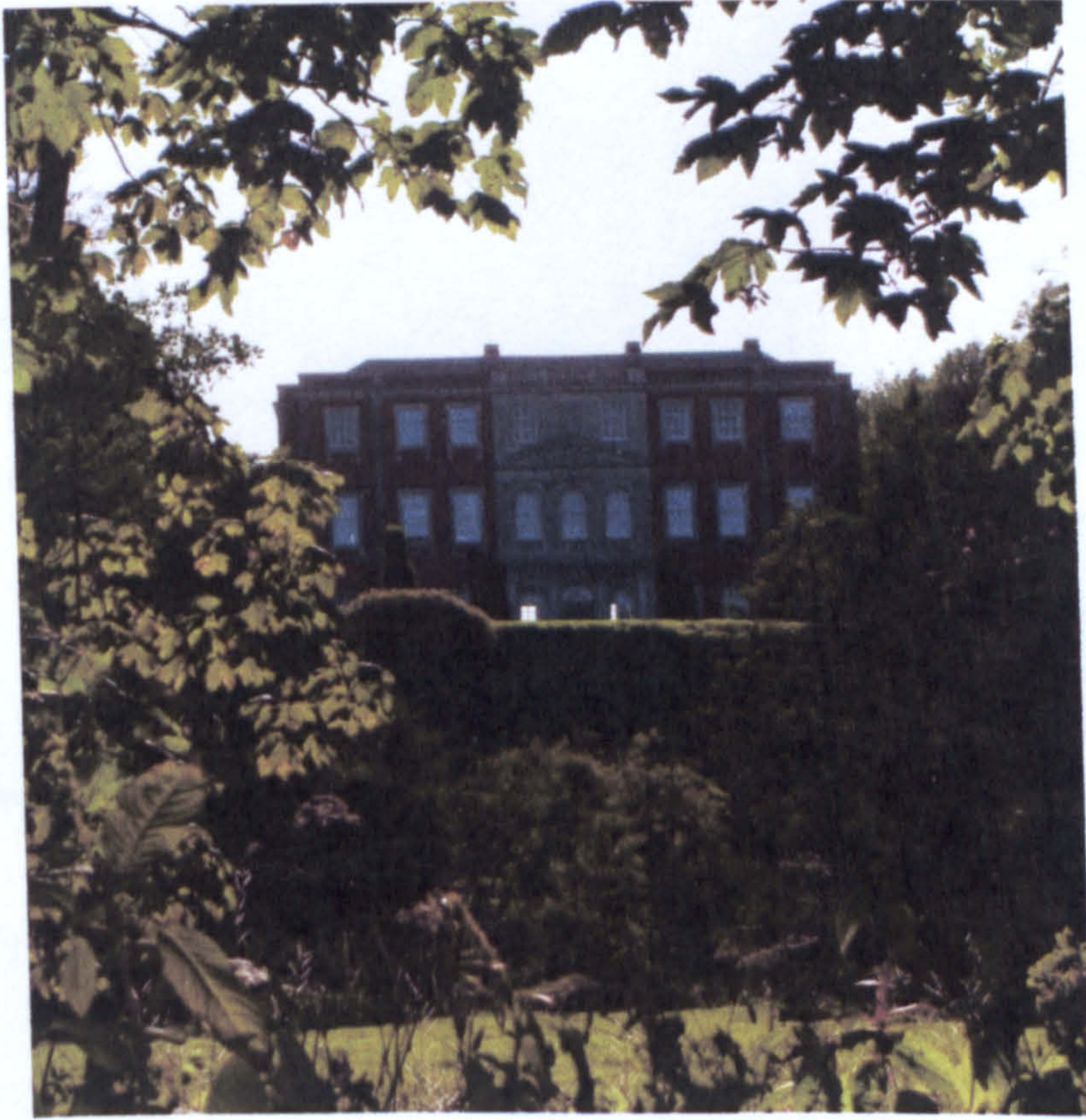
Plate 142: Aldby Park: Photo of the west terraces
