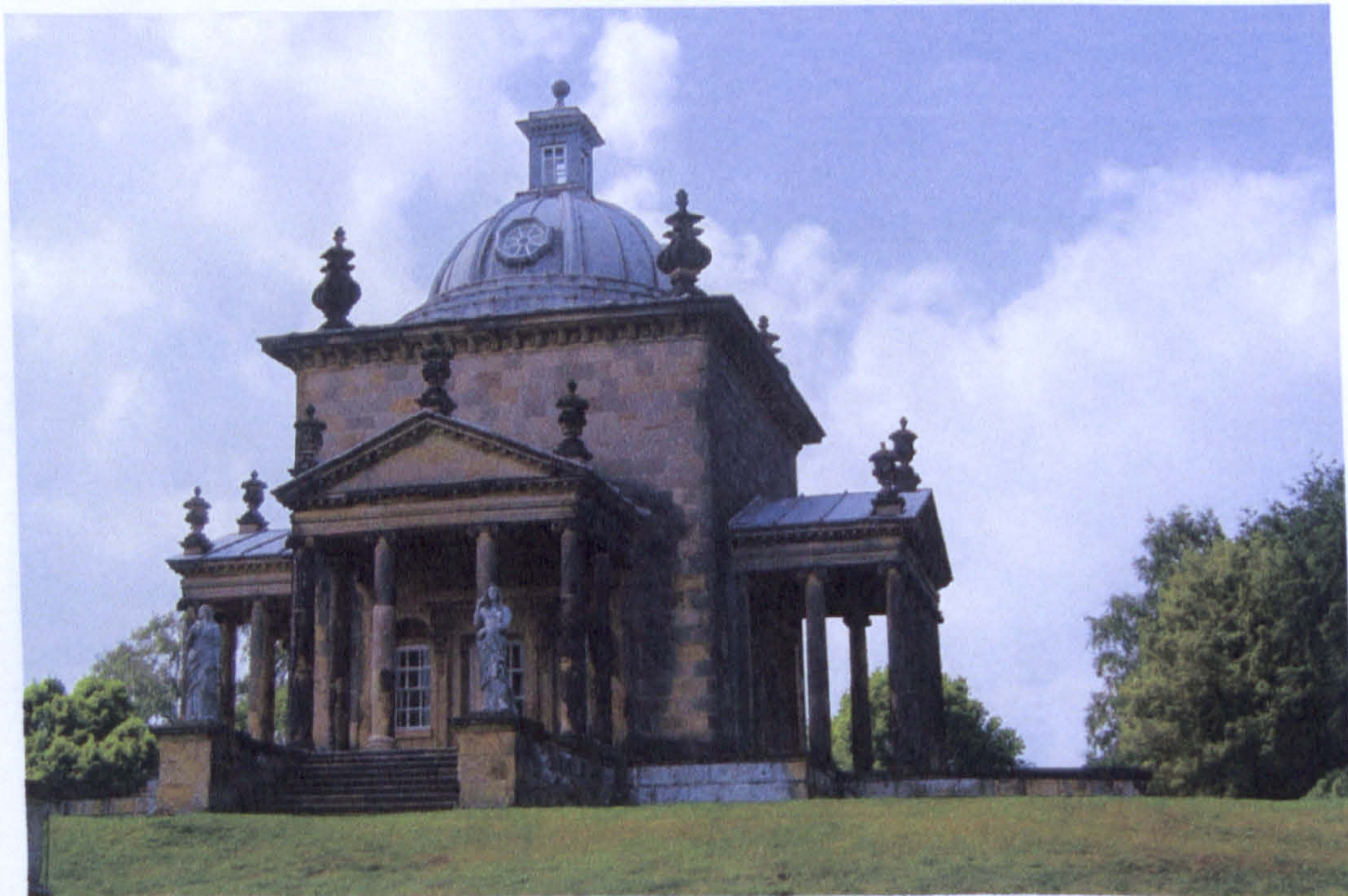
Plate 31: Castle Howard: Temple of Four Winds built by Vanbrugh 1724-8.
