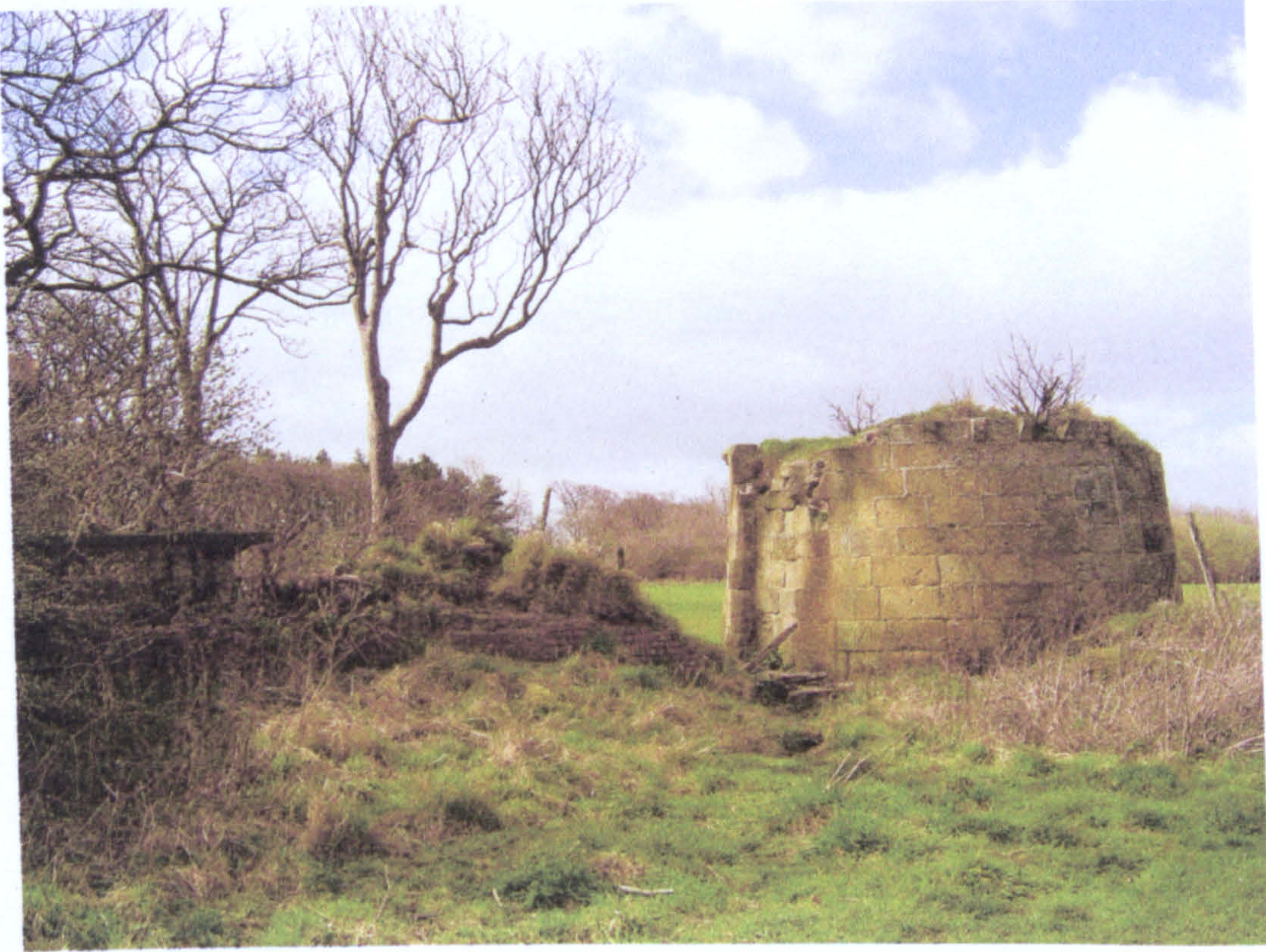
Plate 76: Kirkleatham Hall: Current condition of bastion.
