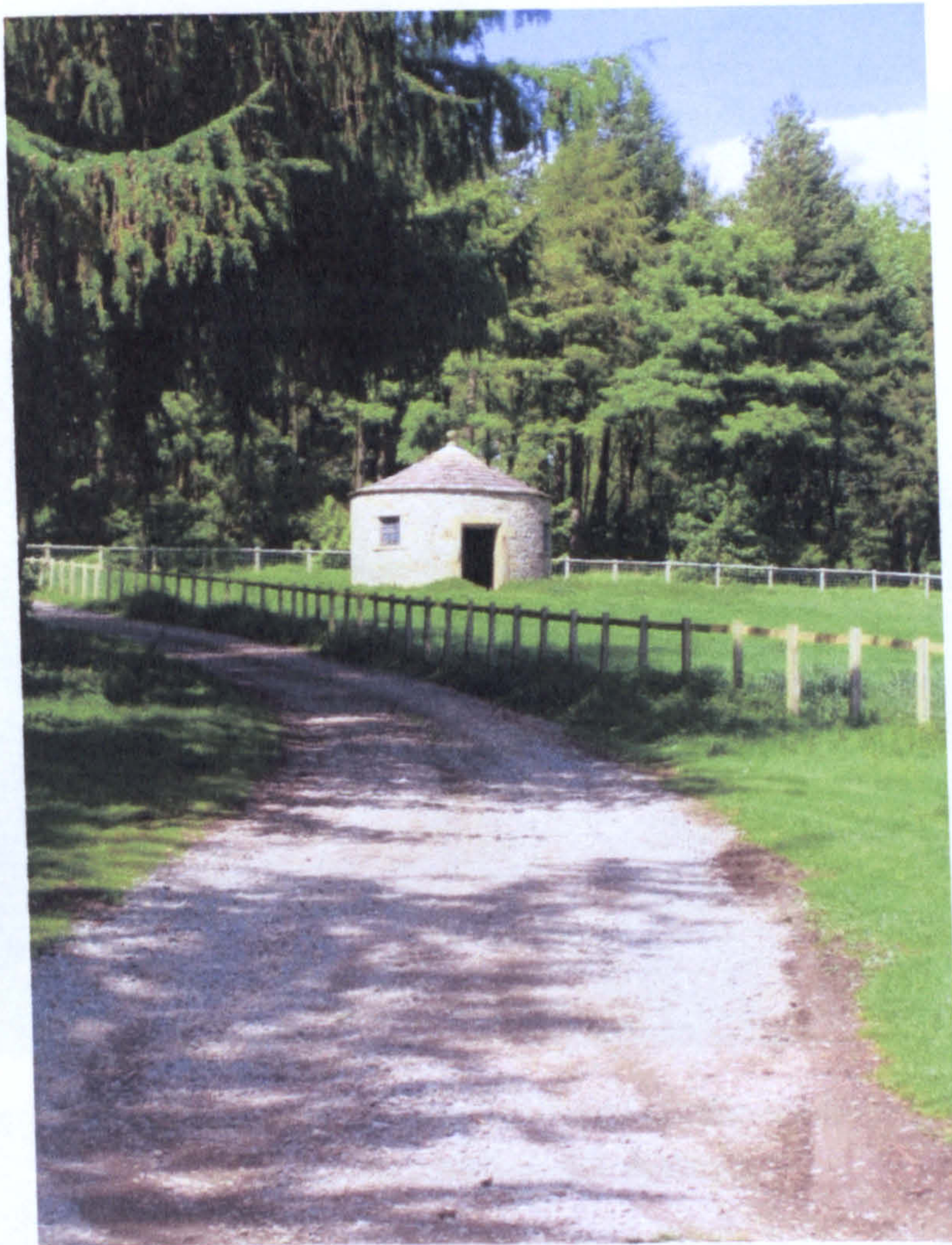
Plate 22: Bolton Hall: Stables to north-east of house.
