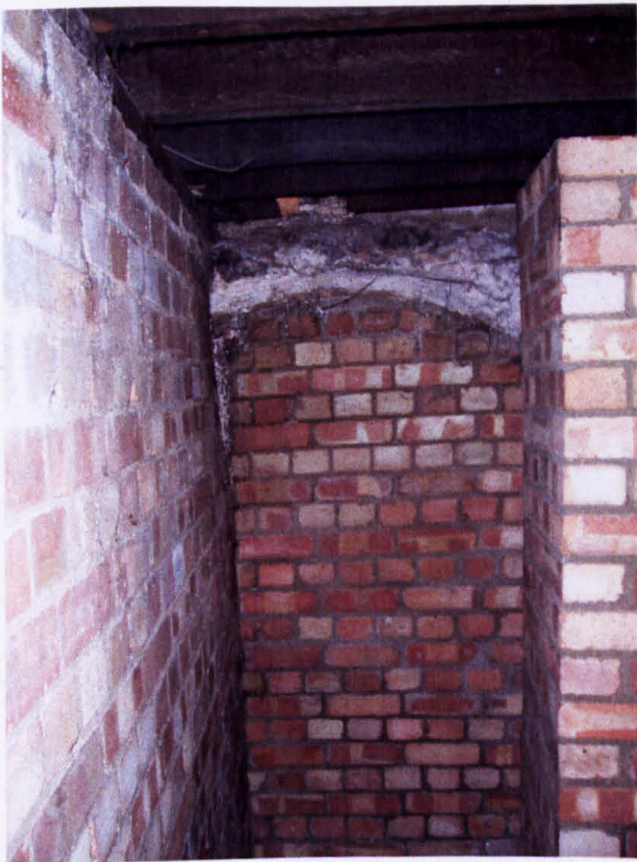
Fig. 45. 8 Charing Cross: north-east corner, showing blocked-up arched entranceway in east wall.
