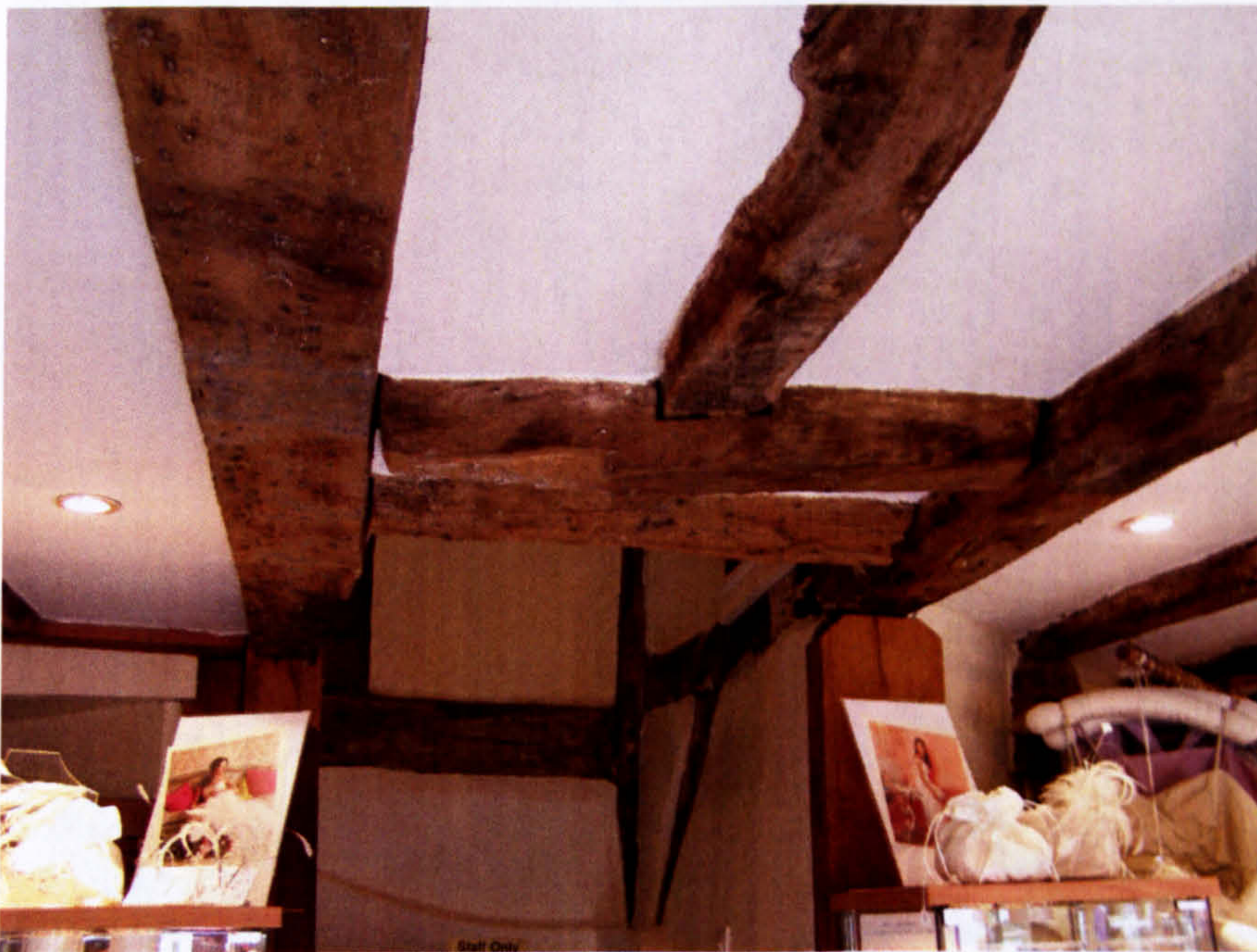
Fig. 75. 64 Goodramgate: staircase opening in the south bay, leading to first-floor level.
