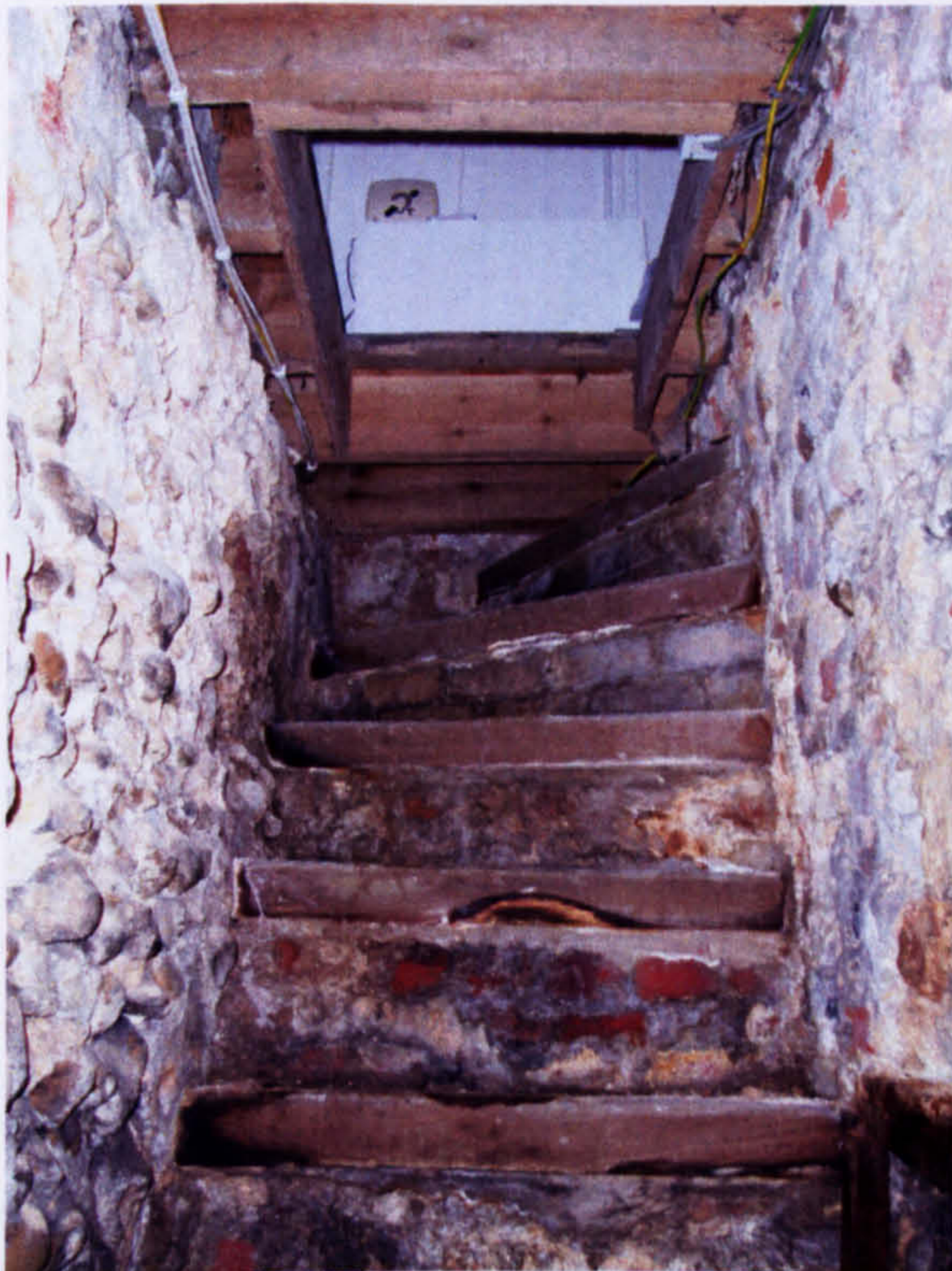
Fig. 30. 15 Bedford Street: stairway into undercroft.
