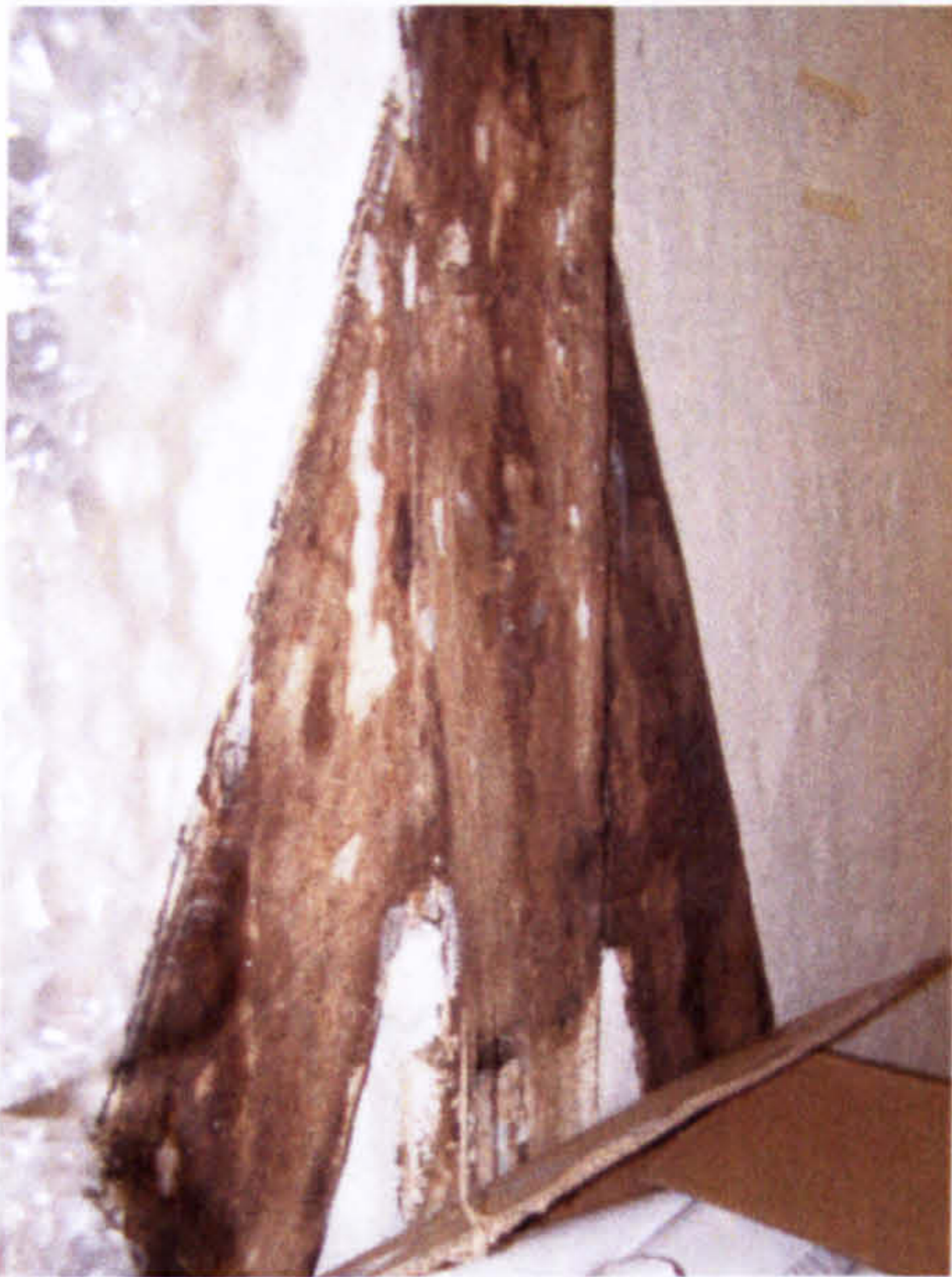
Fig. 79. 64 Goodramgate: tie-beams and crown post trusses exposed in loft.
