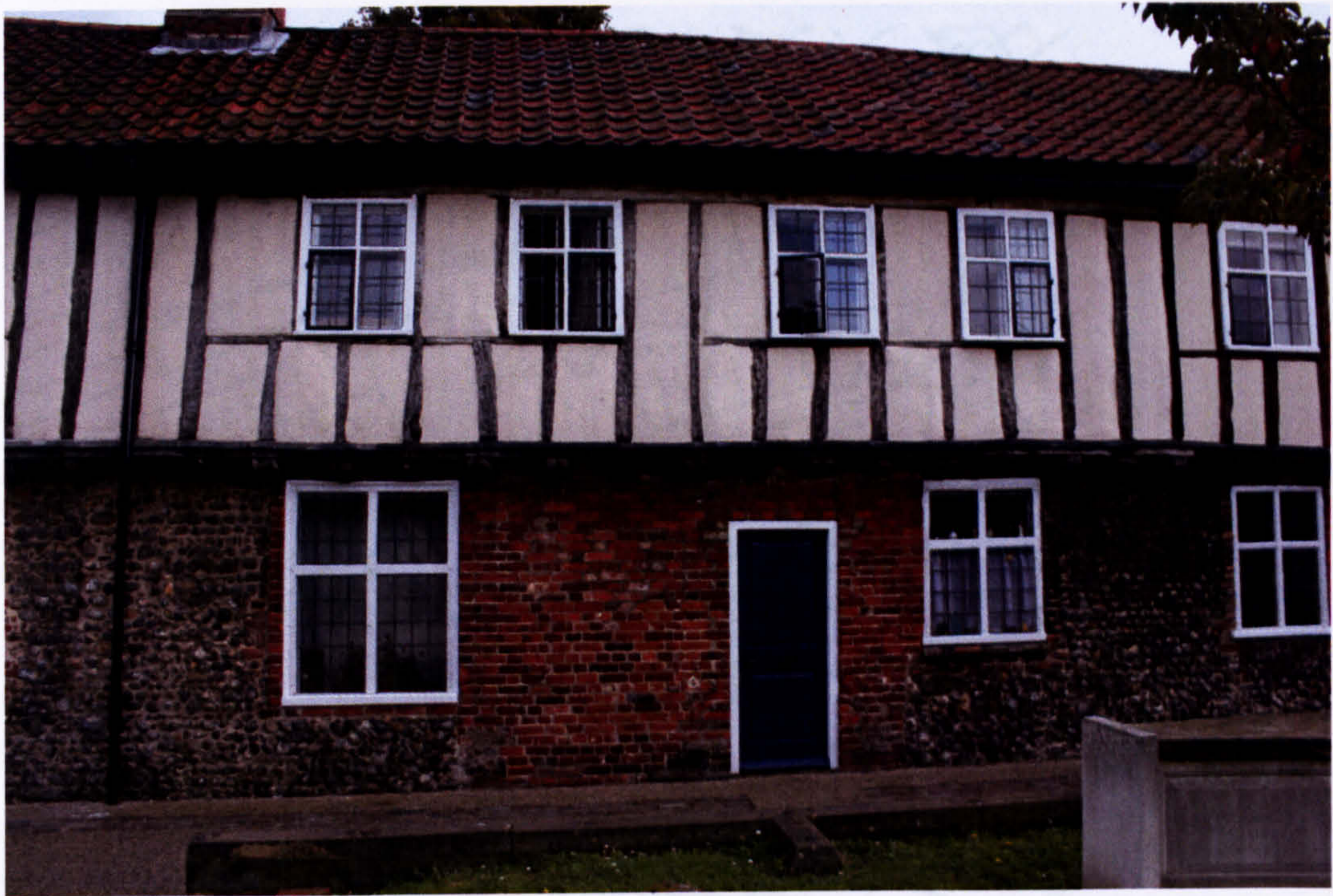
Fig. 49. 6 Gildencroft: remains of former timber window-sills at first-floor level.
