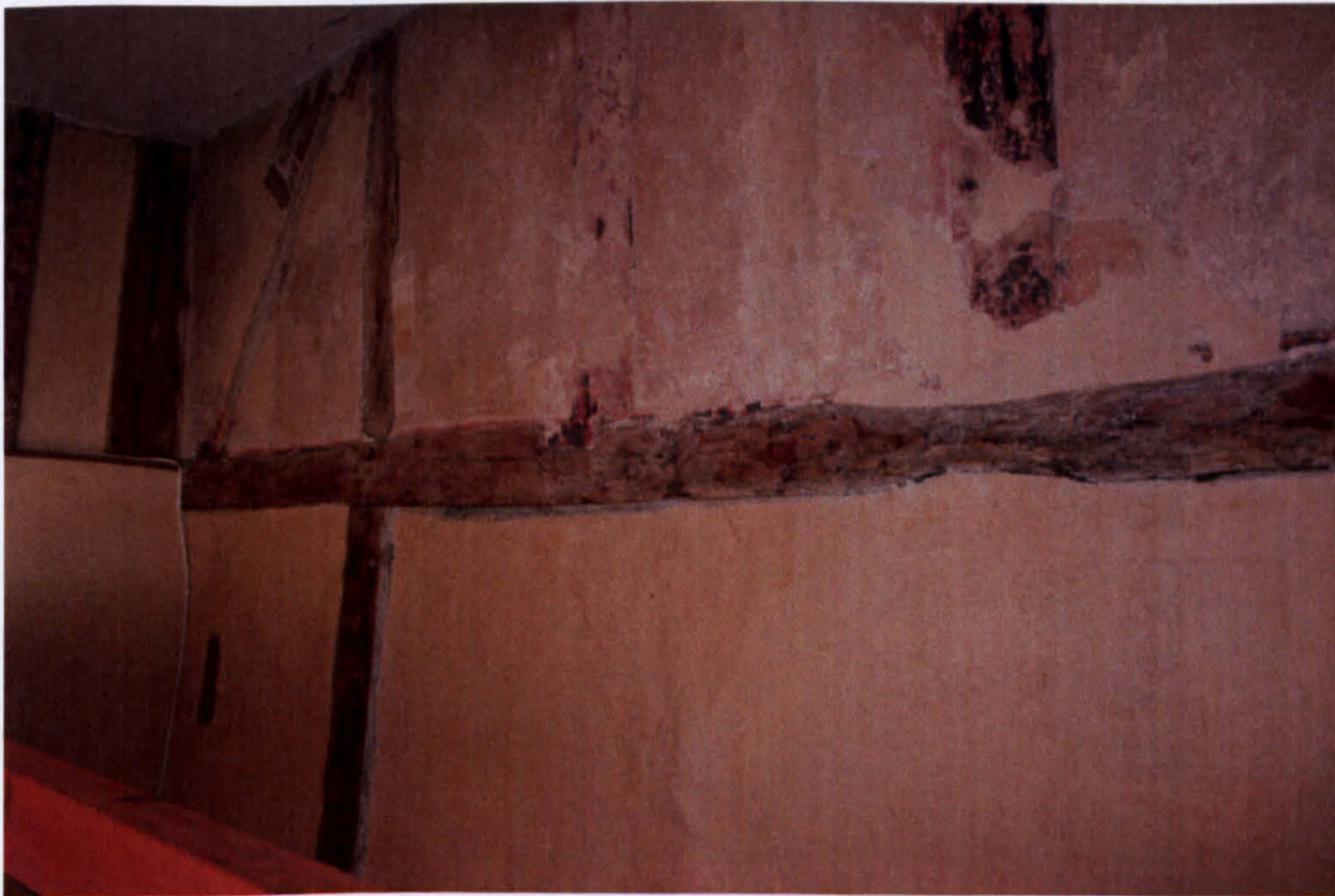
Fig. 41. 8 Charing Cross: first-floor level, west partition.
