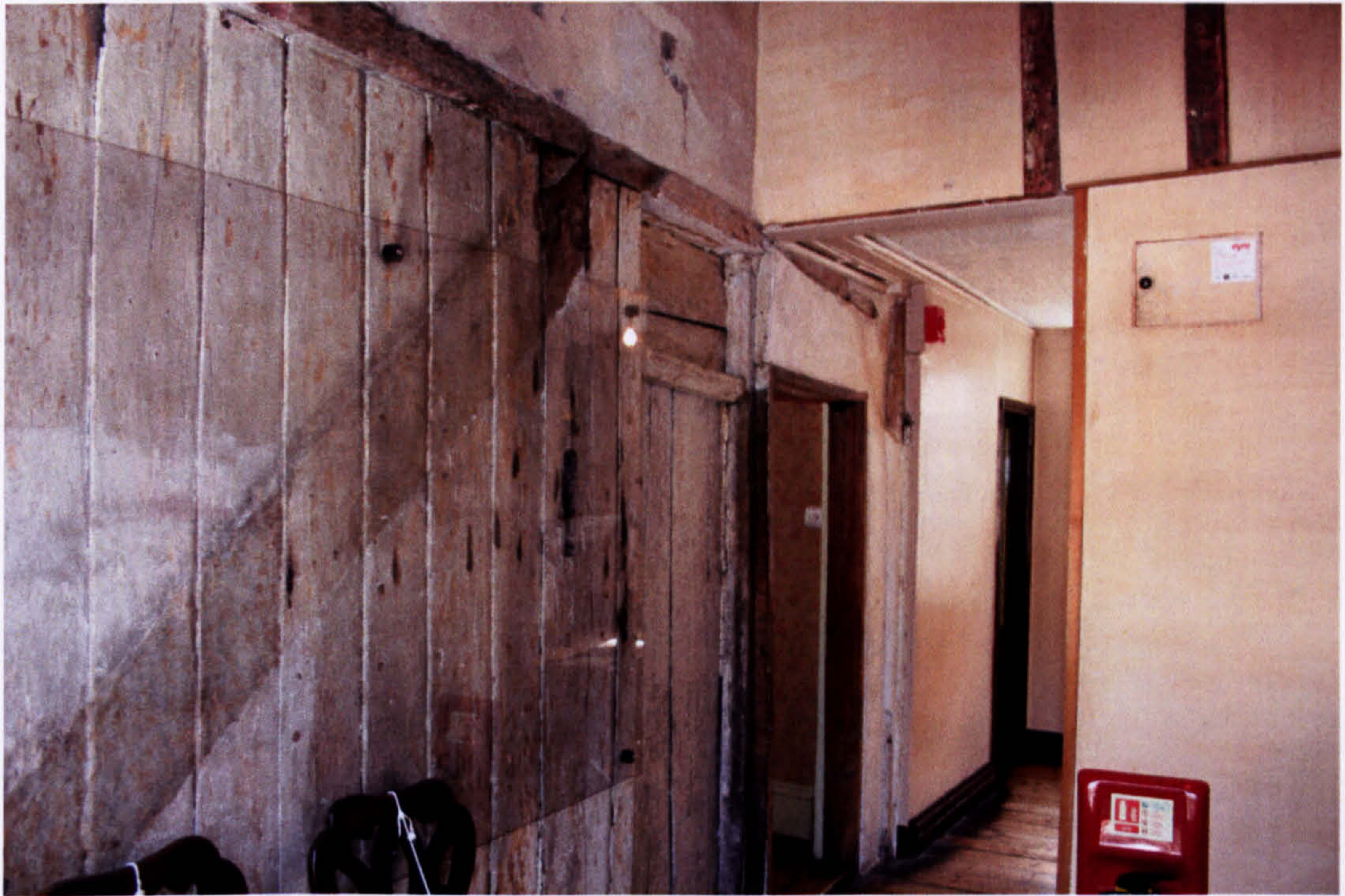
Fig. 43. 8 Charing Cross: first-floor level, east wall, showing panelling and old door.
