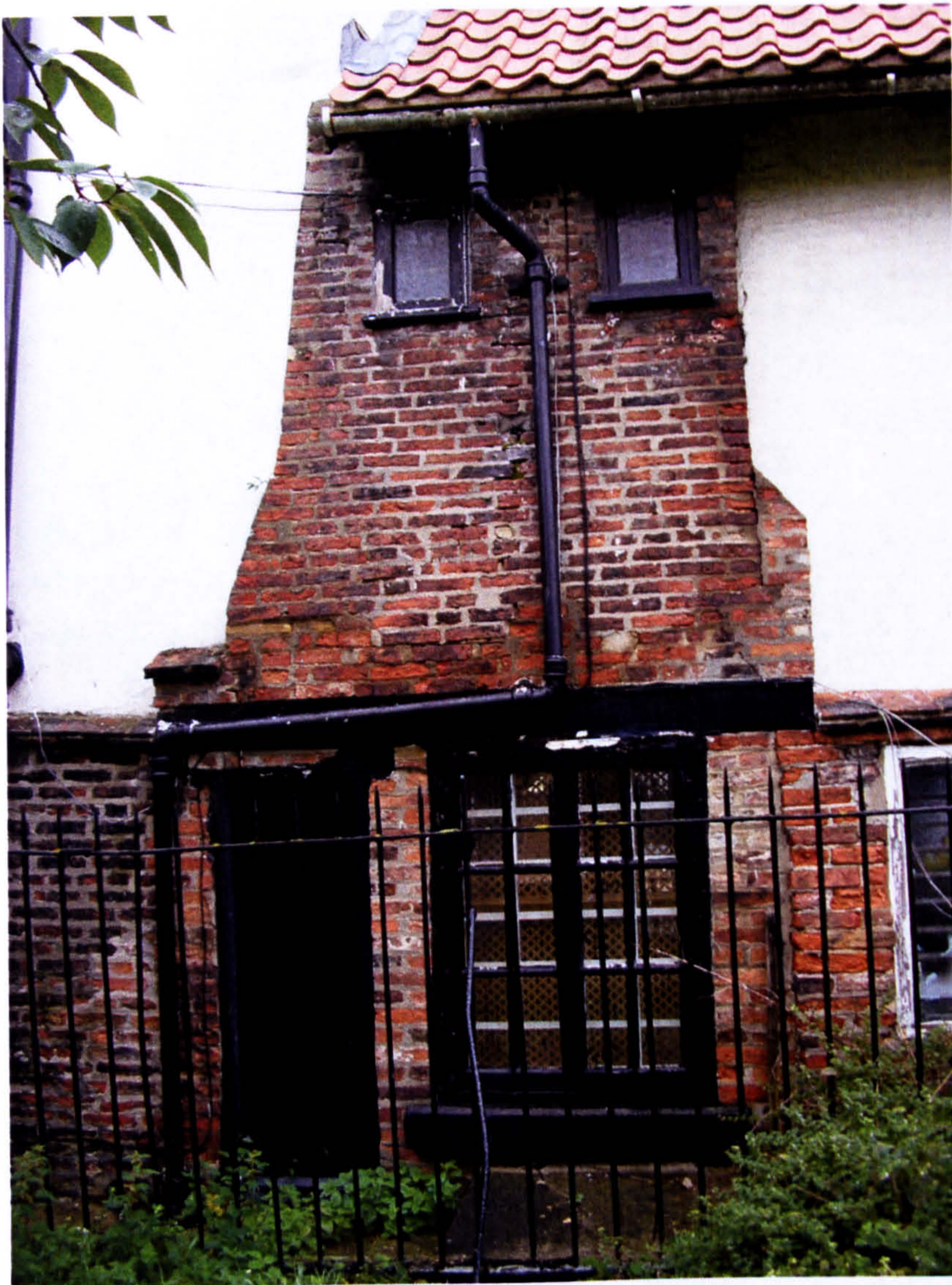
Fig. 63a. 68 Goodramgate: remains of chimney stack on west wall.
