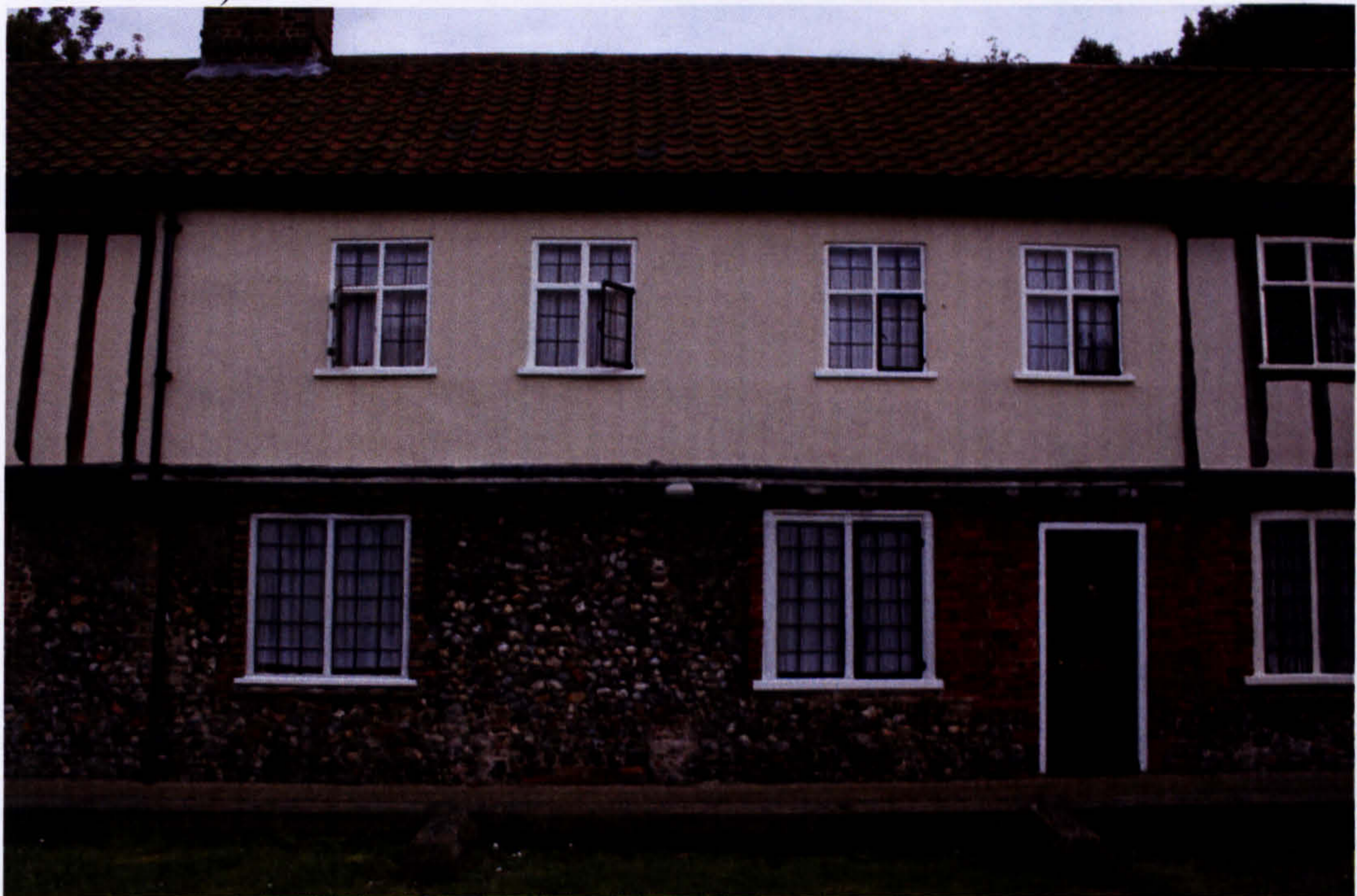
Fig. 48d. 10 Gildencroft: current and blocked-up ground-floor doorways (between the two windows).
