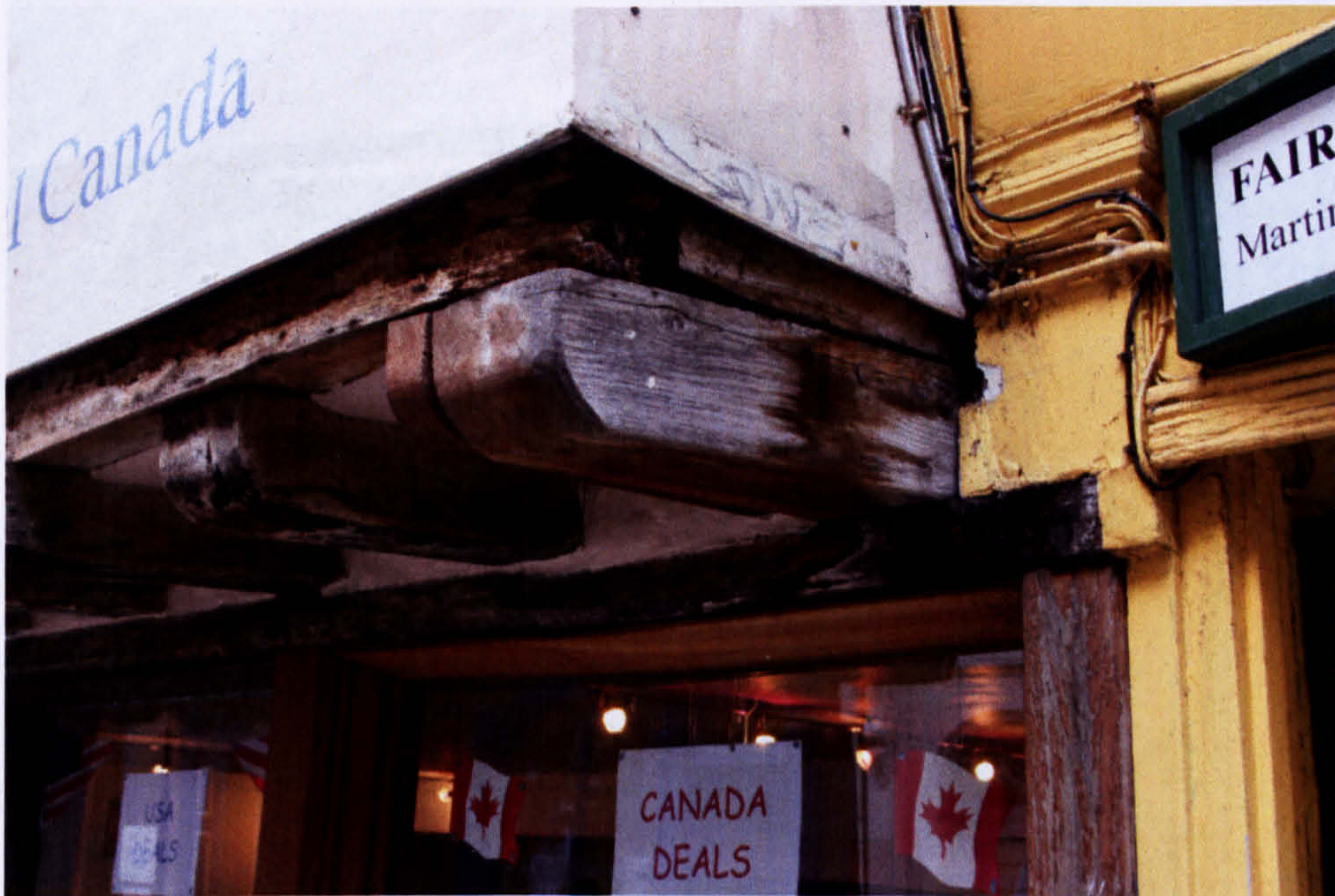
Fig. 20. 15 Bedford Street: east end of jetty.
