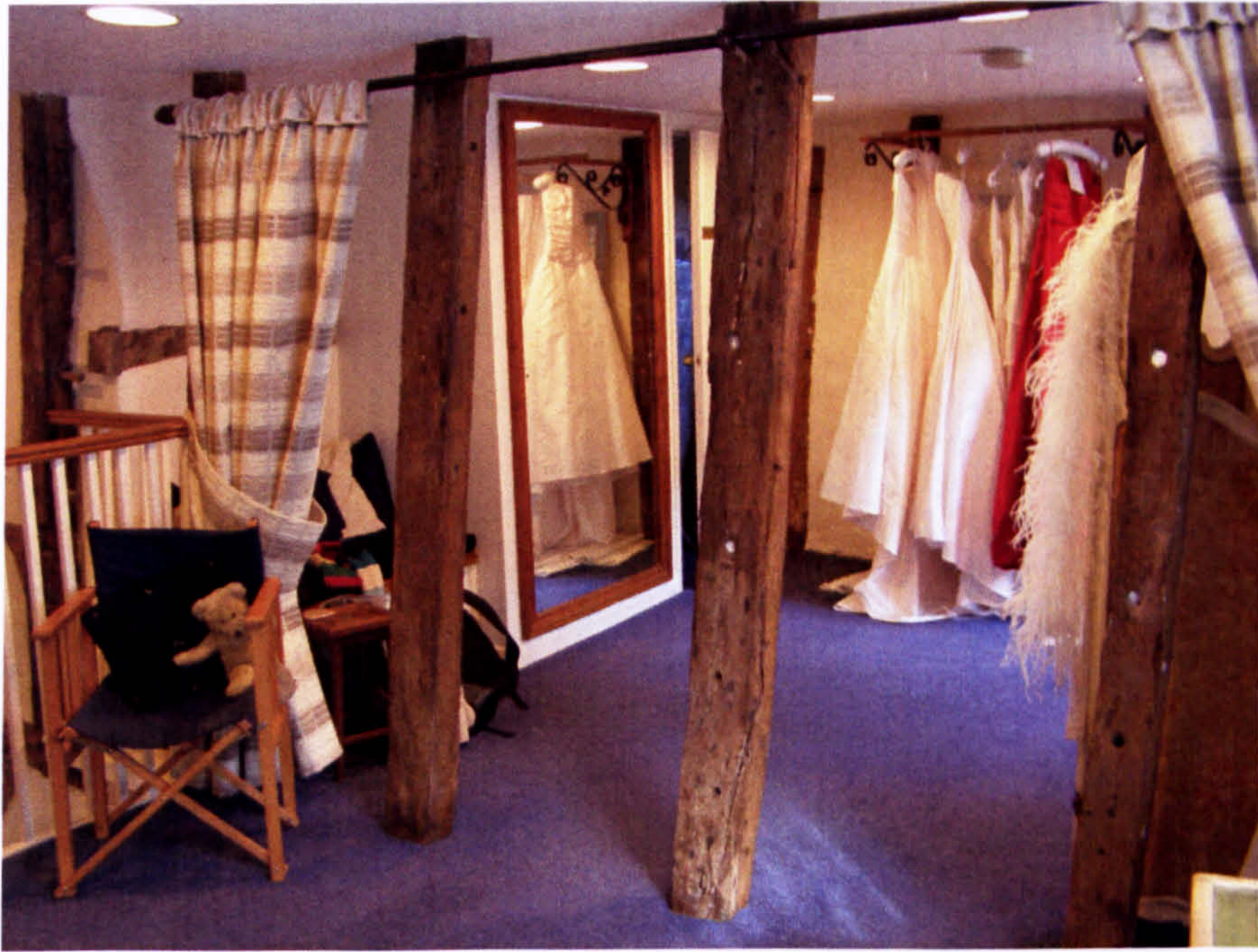
Fig. 76. 64 Goodramgate: first-floor level, central truss studs.
