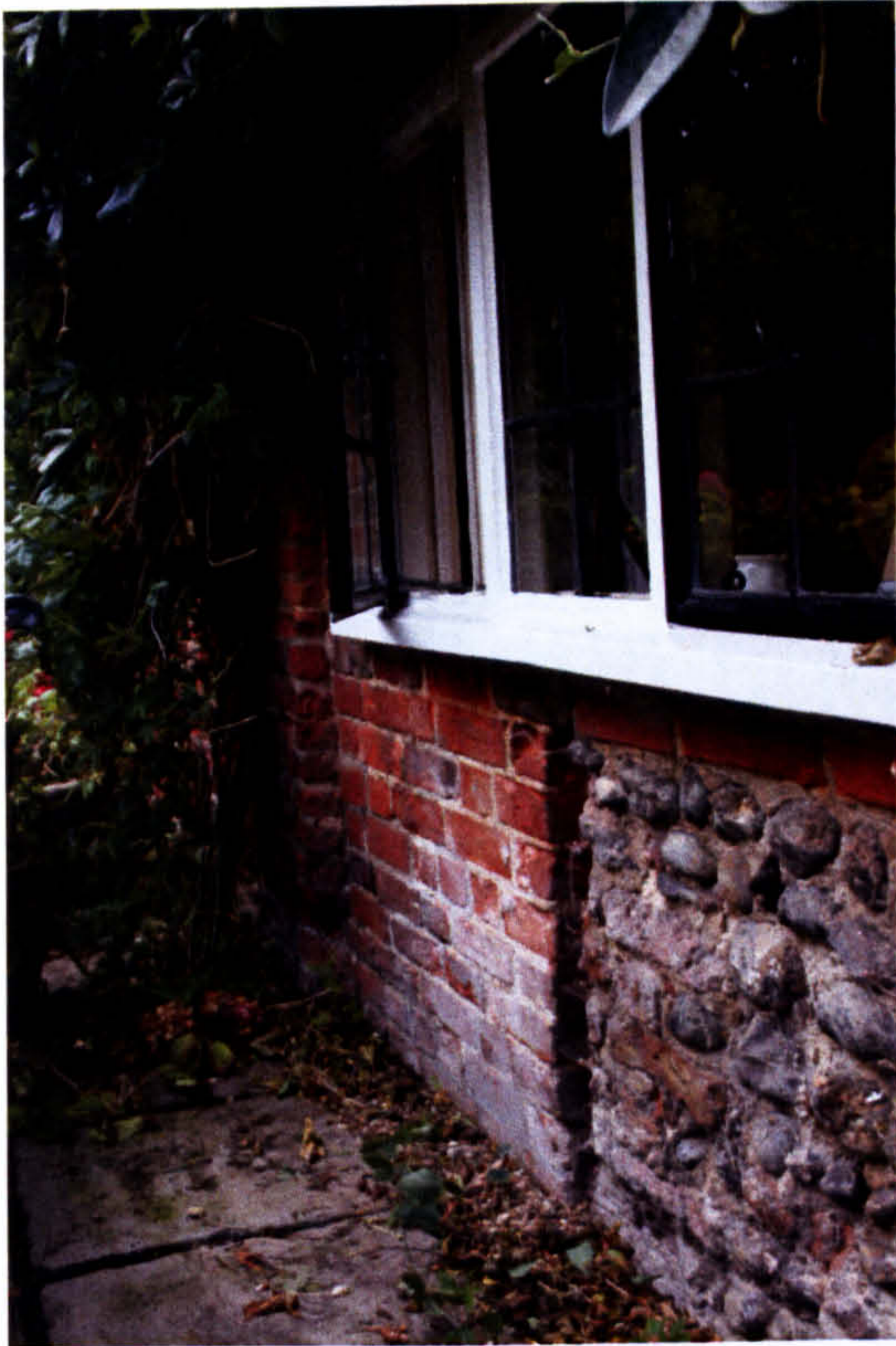
Fig. 57a. 10 Gildencroft: ground-floor level, blocked-up doorway on south (rear) wall.
