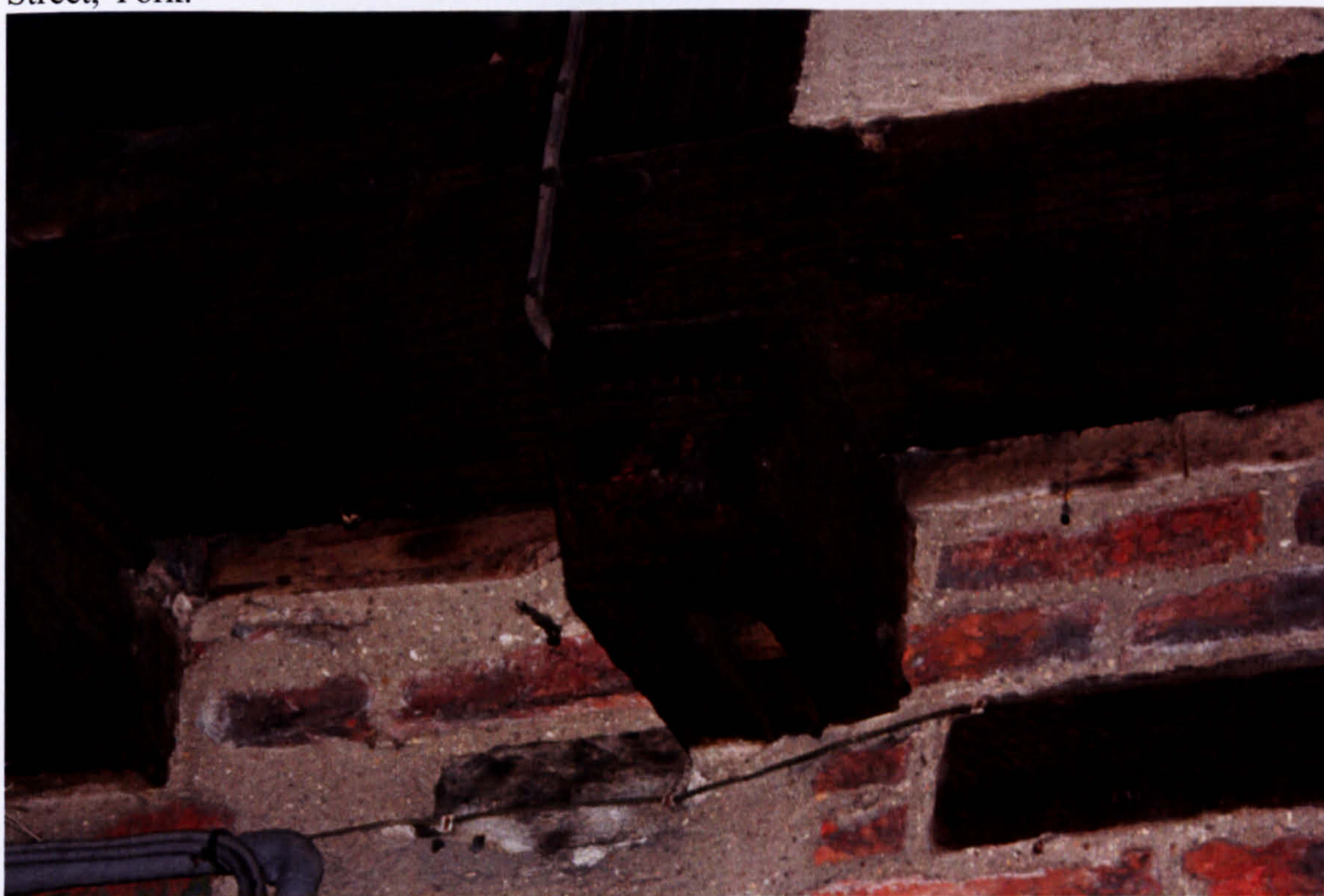
Fig. 12b. Detail of the pellet decorations on the joist-ends of the jetty at 11-12 College Street, York.
