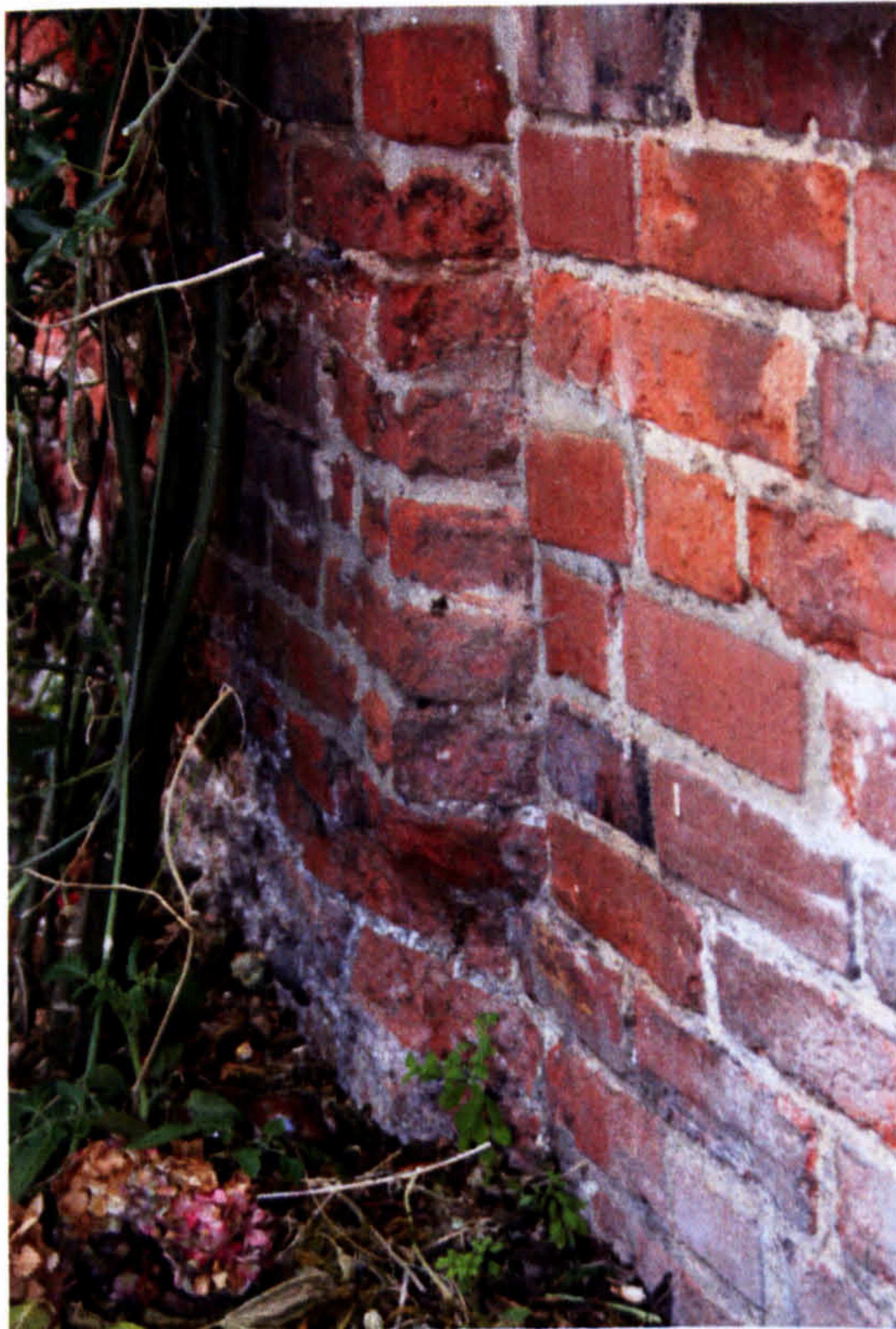
Fig 57b. 10 Gildencroft: detail of blocked-up doorway on south (rear) wall.
