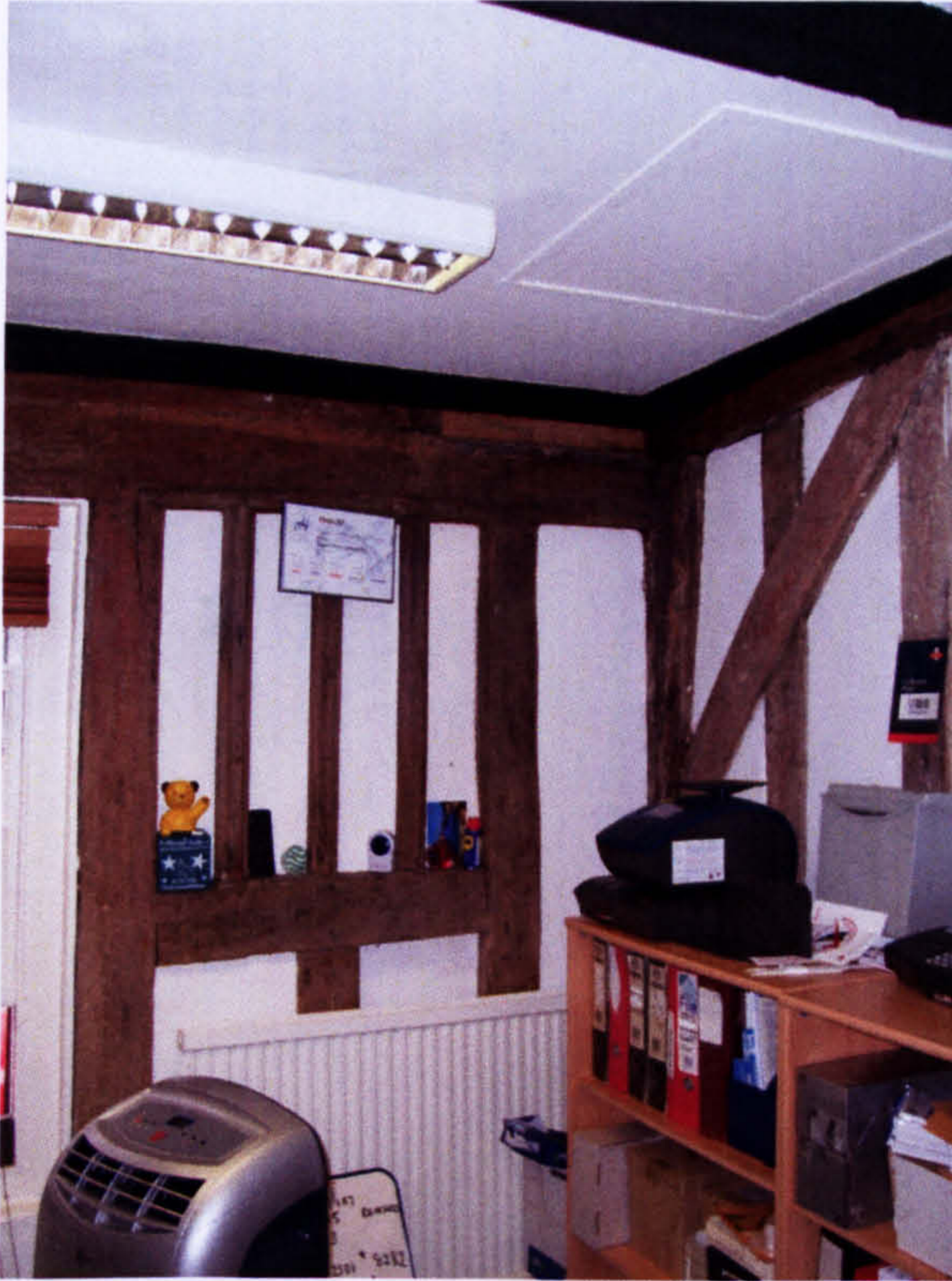
Fig. 23. 15 Bedford Street: mullioned window on south wall.
