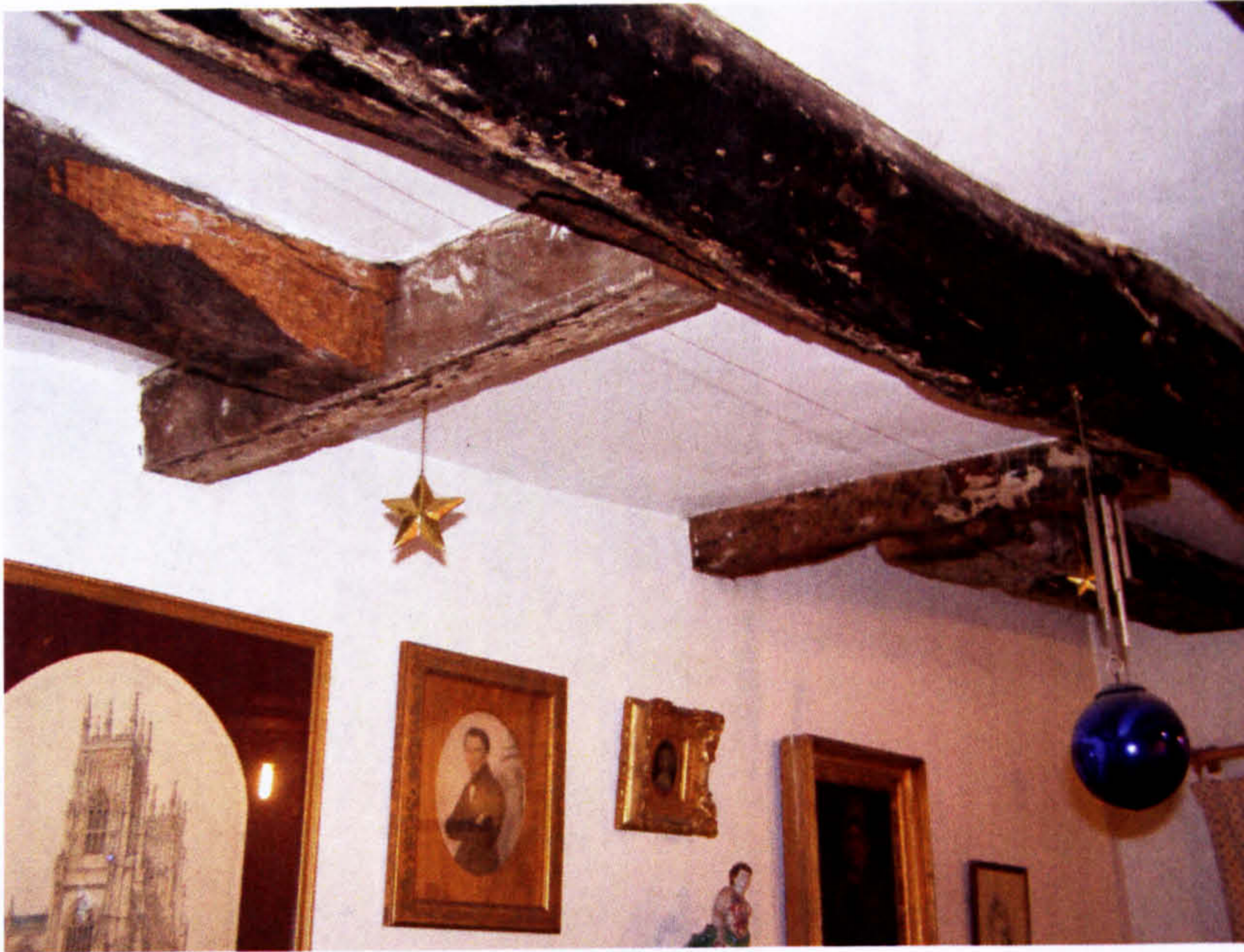
Fig. 89. 2 All Saints' Lane: ground-floor level, position of inserted chimney stack to the east of the unit.
