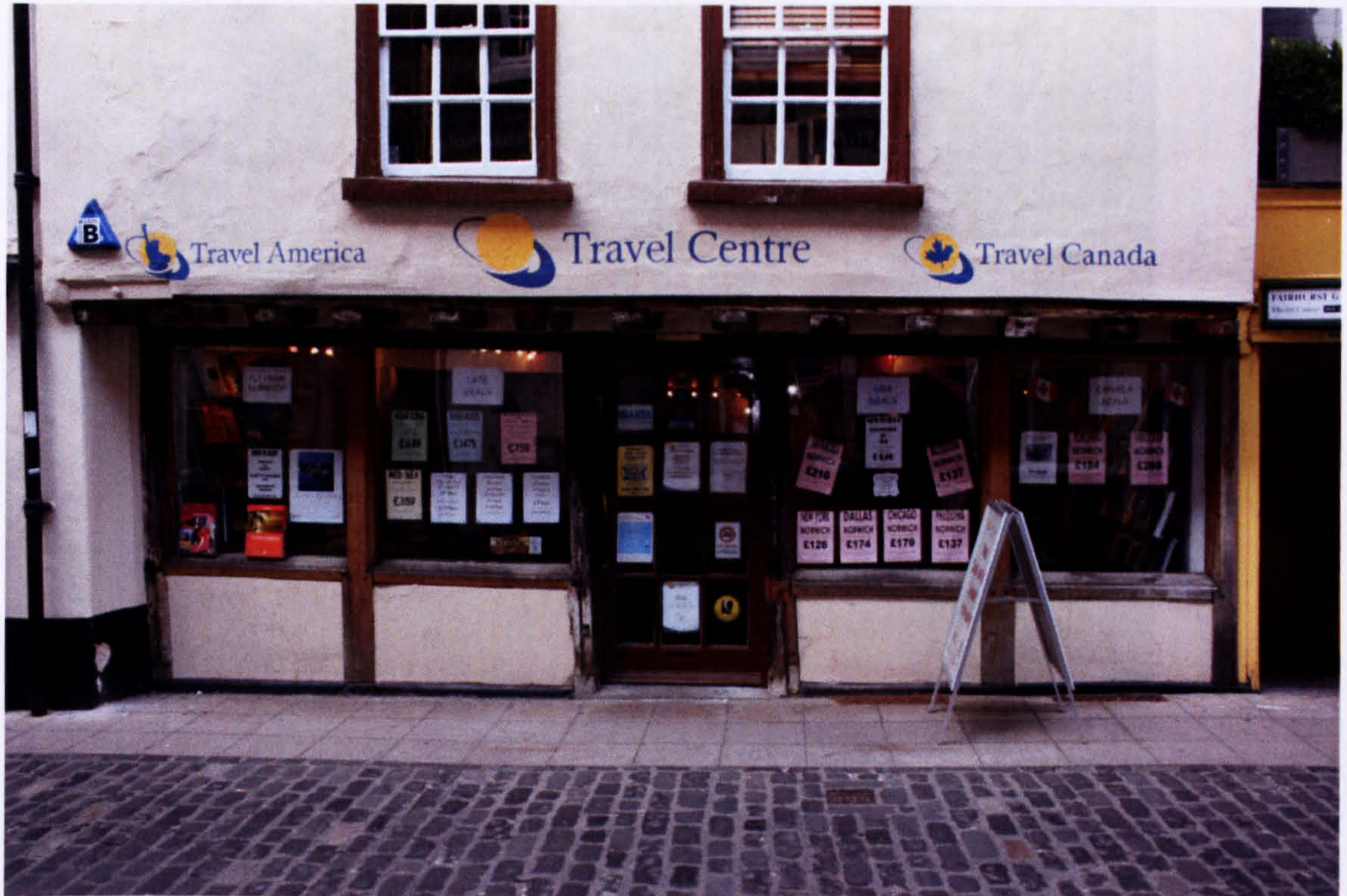
Fig. 17. 15 Bedford Street: shop front.
