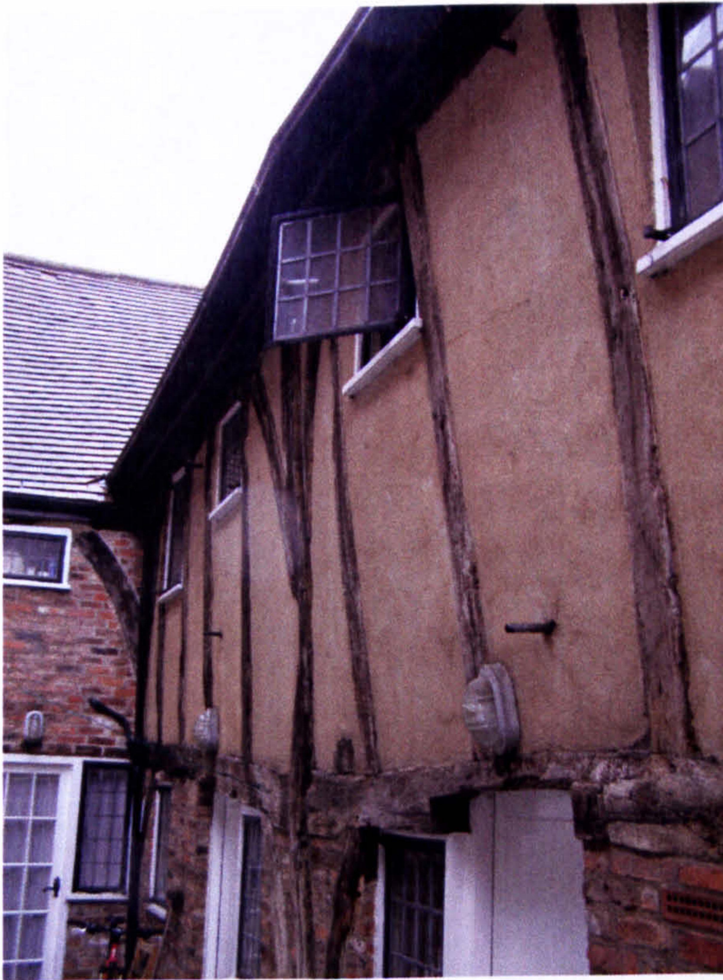
Fig. 81. 1 and 2 All Saints' Lane, first-floor north wall.
