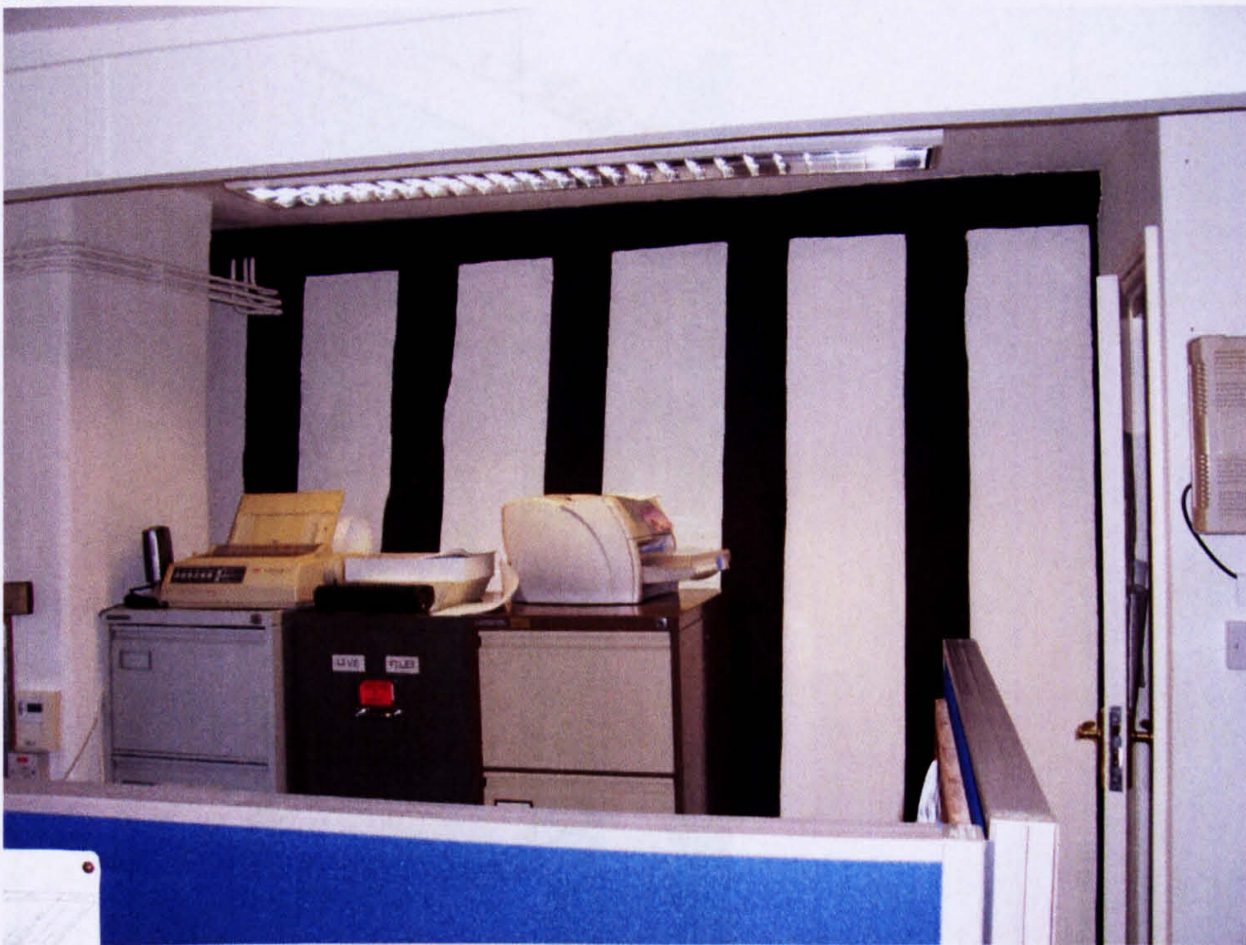
Fig. 22. 15 Bedford Street: exterior view (from extension) of original north wall at first-floor level.
