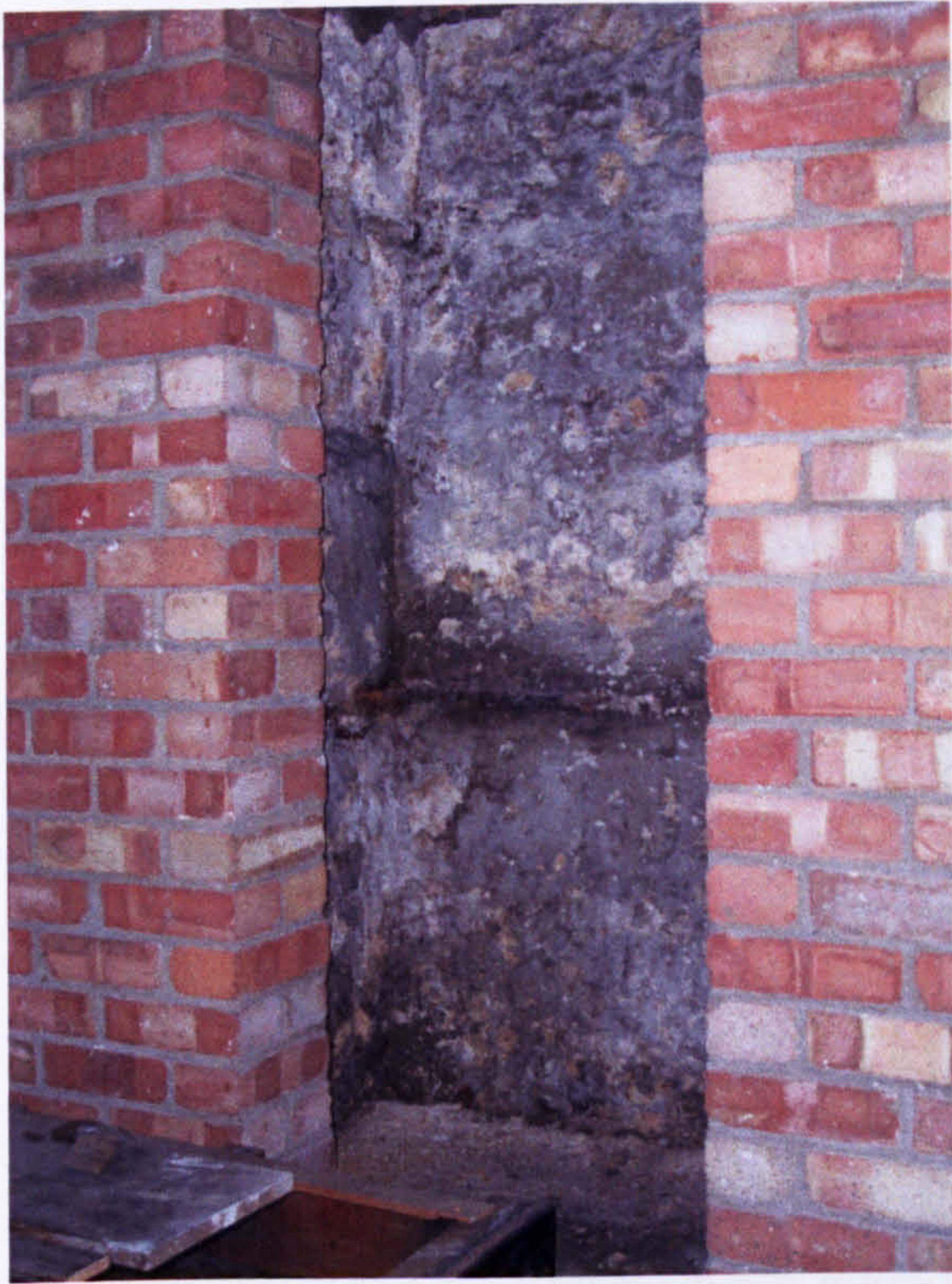
Fig. 44b. 8 Charing Cross: continuation of south wall, showing flint material behind brick pillars.
