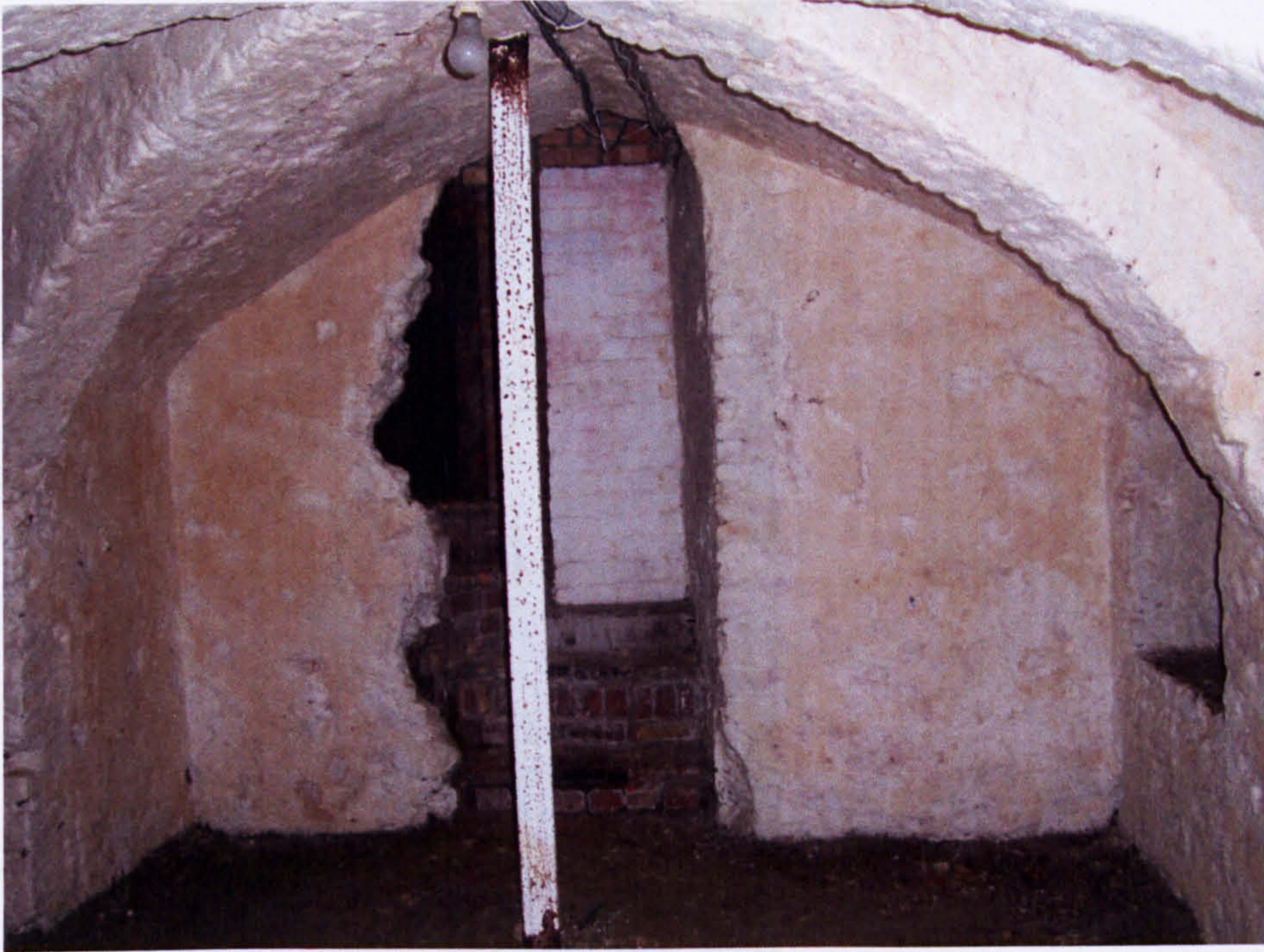
Fig. 26. 15 Bedford Street: entranceway into cellars in south wall of undercroft.
