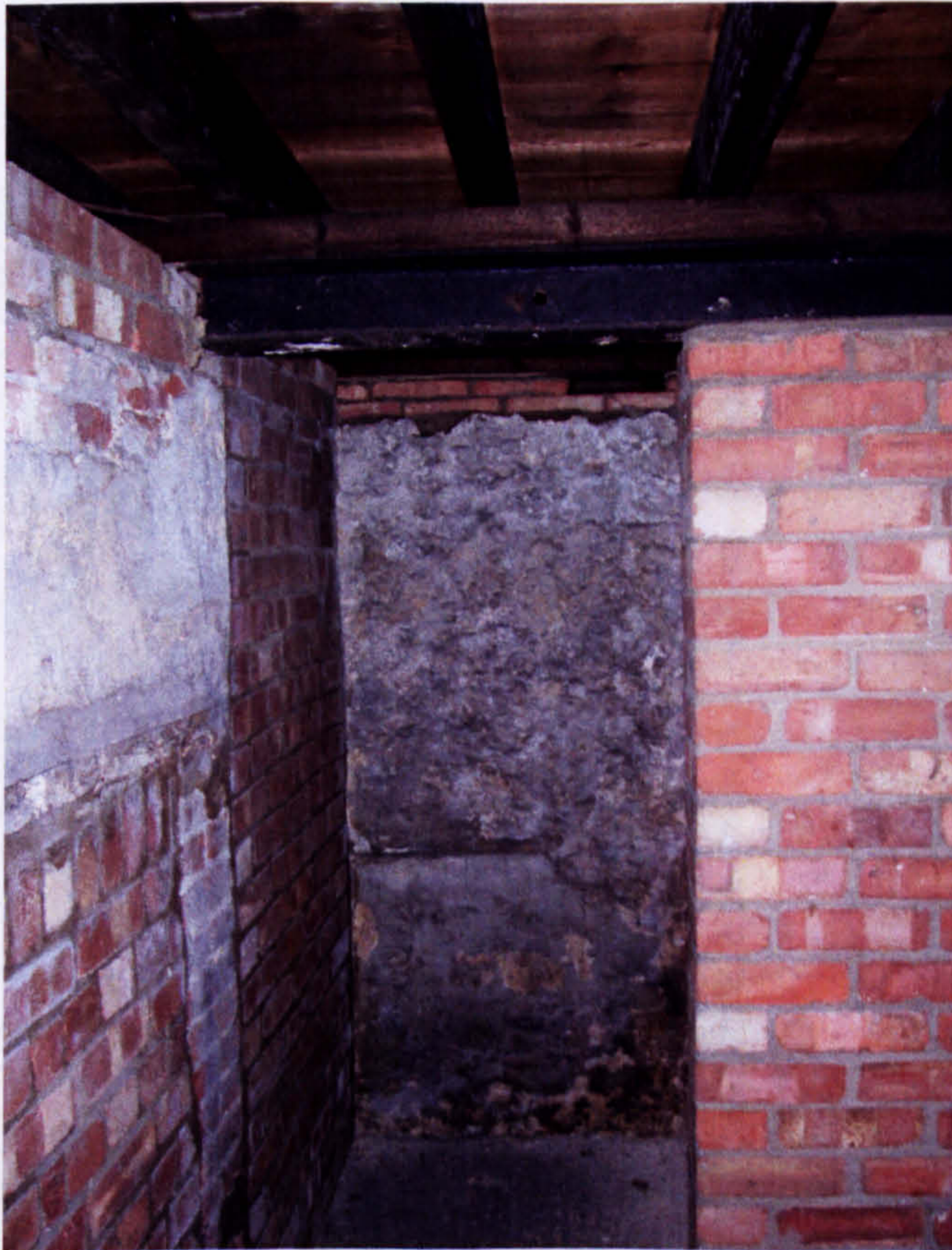
Fig. 44a: 8 Charing Cross: south-east corner of cellar, showing flint south wall.
