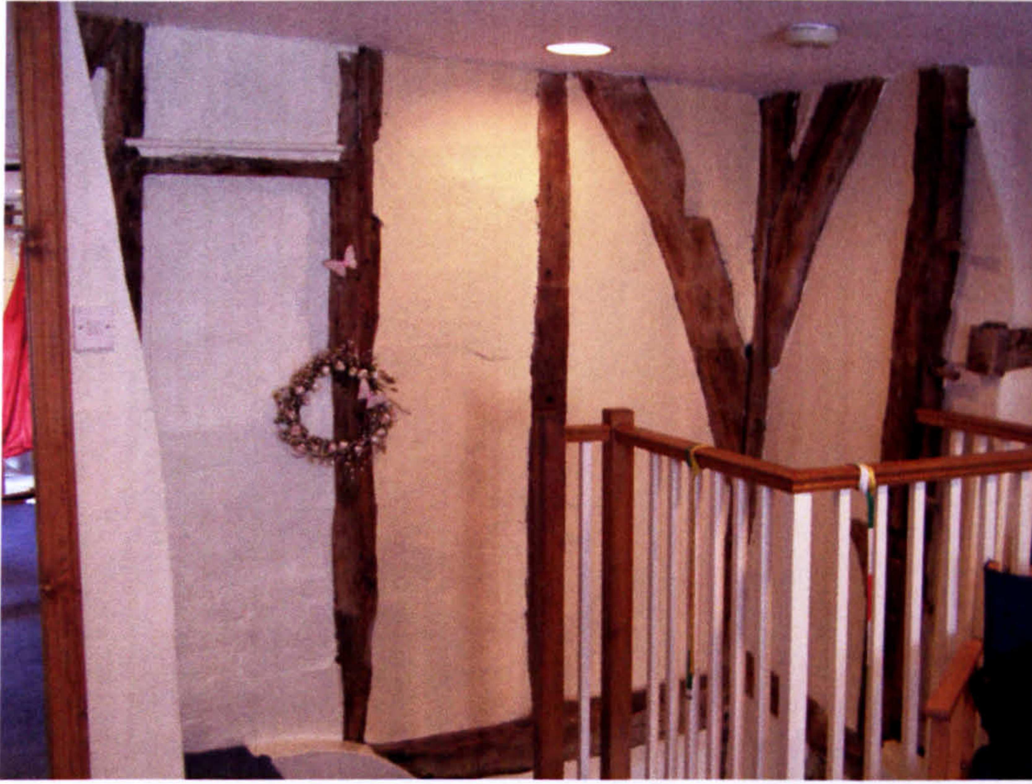
Fig. 78. 64 Goodramgate: first-floor level, west wall.
