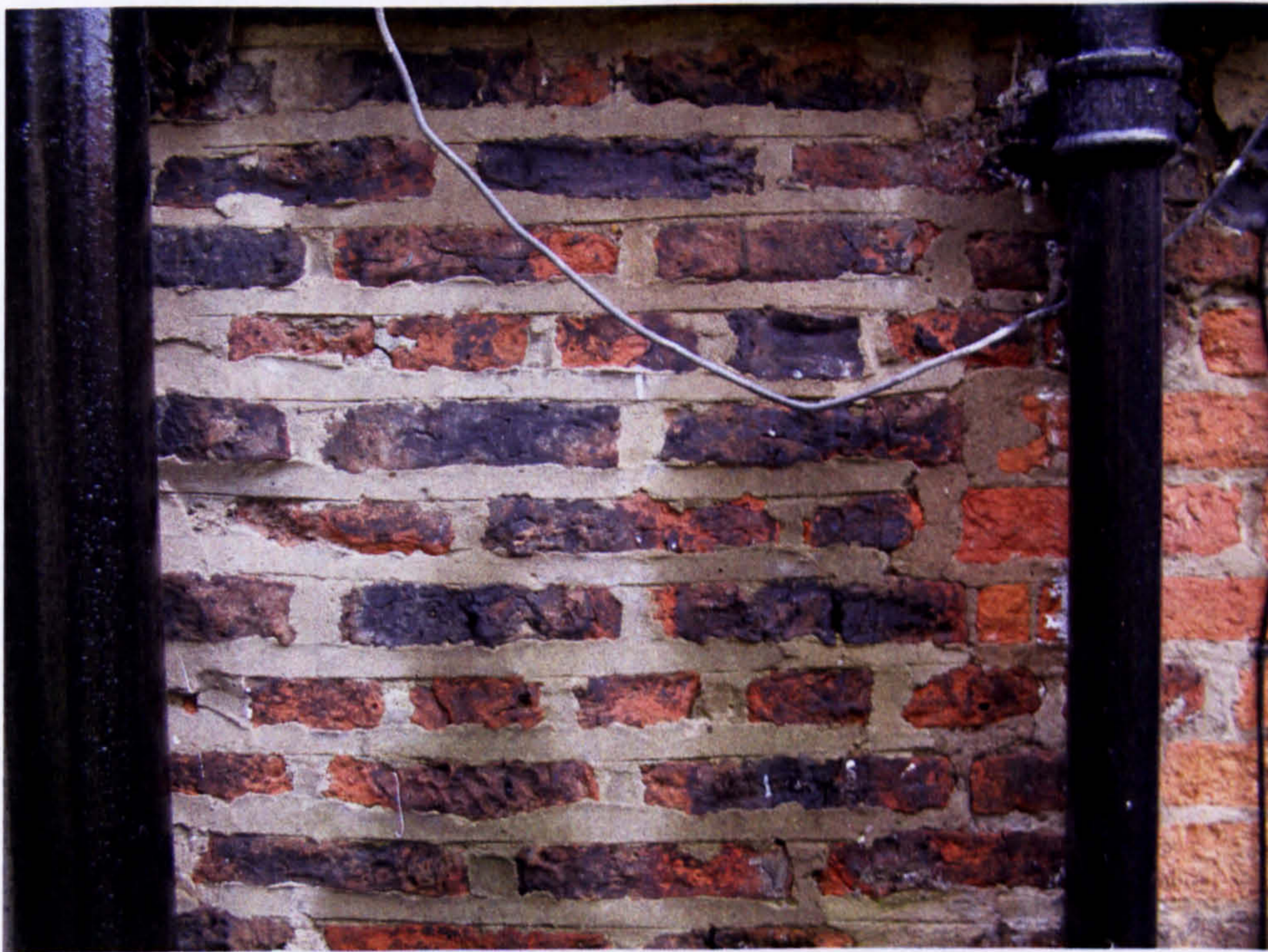
Fig. 63c. 68 Goodramgate: detail of brickwork on west wall at ground-floor level.
