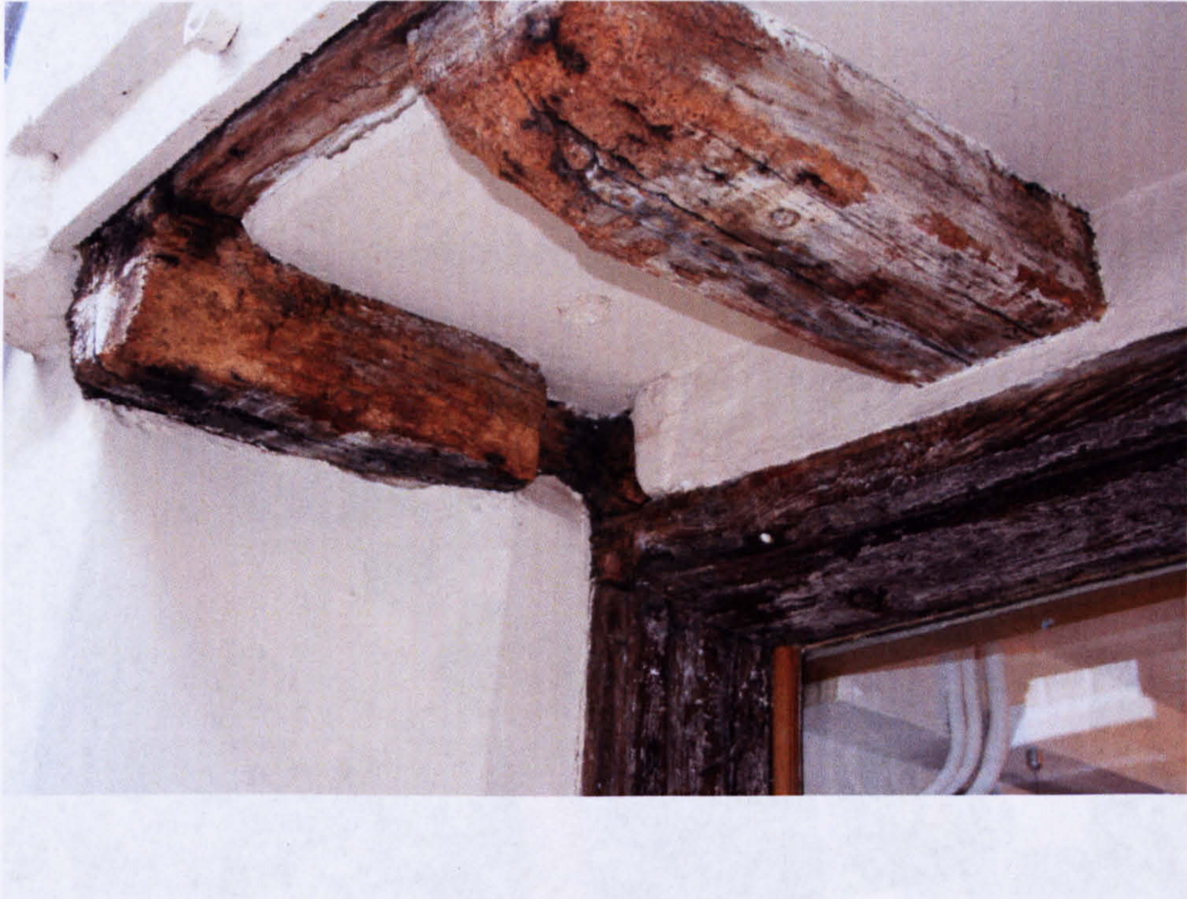
Fig. 19. 15 Bedford Street: west end of jetty.
