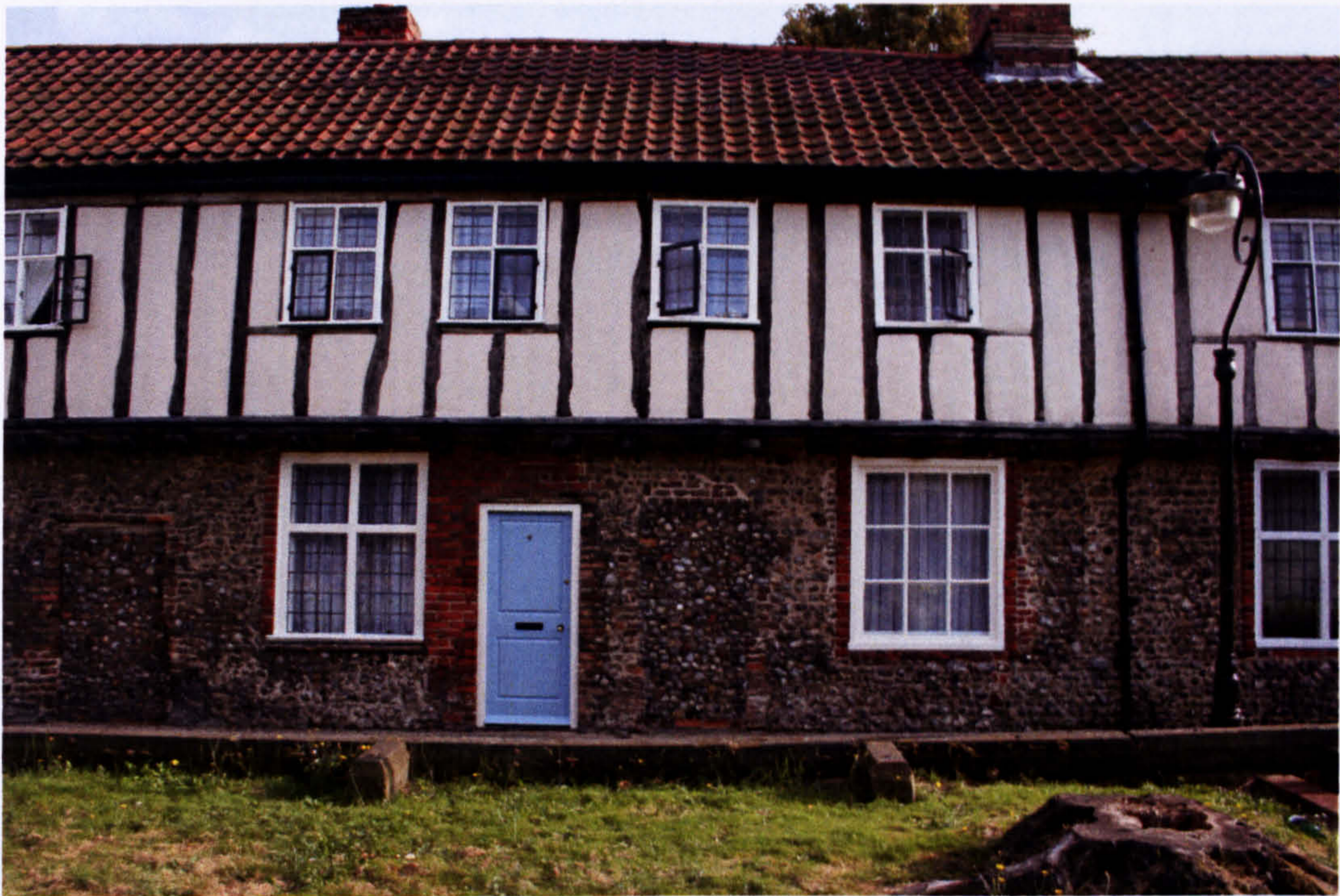
Fig. 48c. 4 Gildencroft: current and blocked-up ground-floor doorways.
