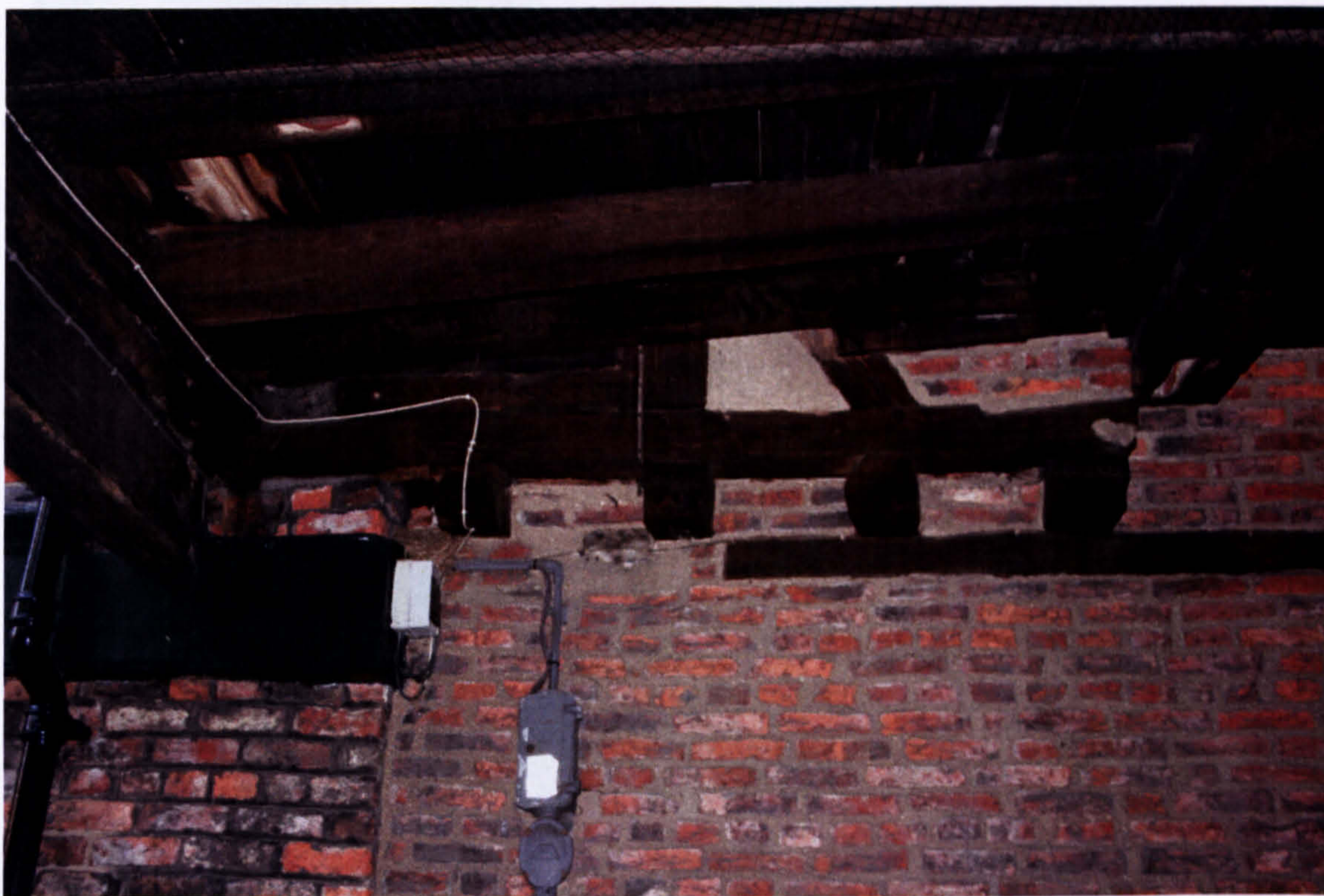
Fig. 12a. Remains of the Jetty at 11-12 College Street, York.
