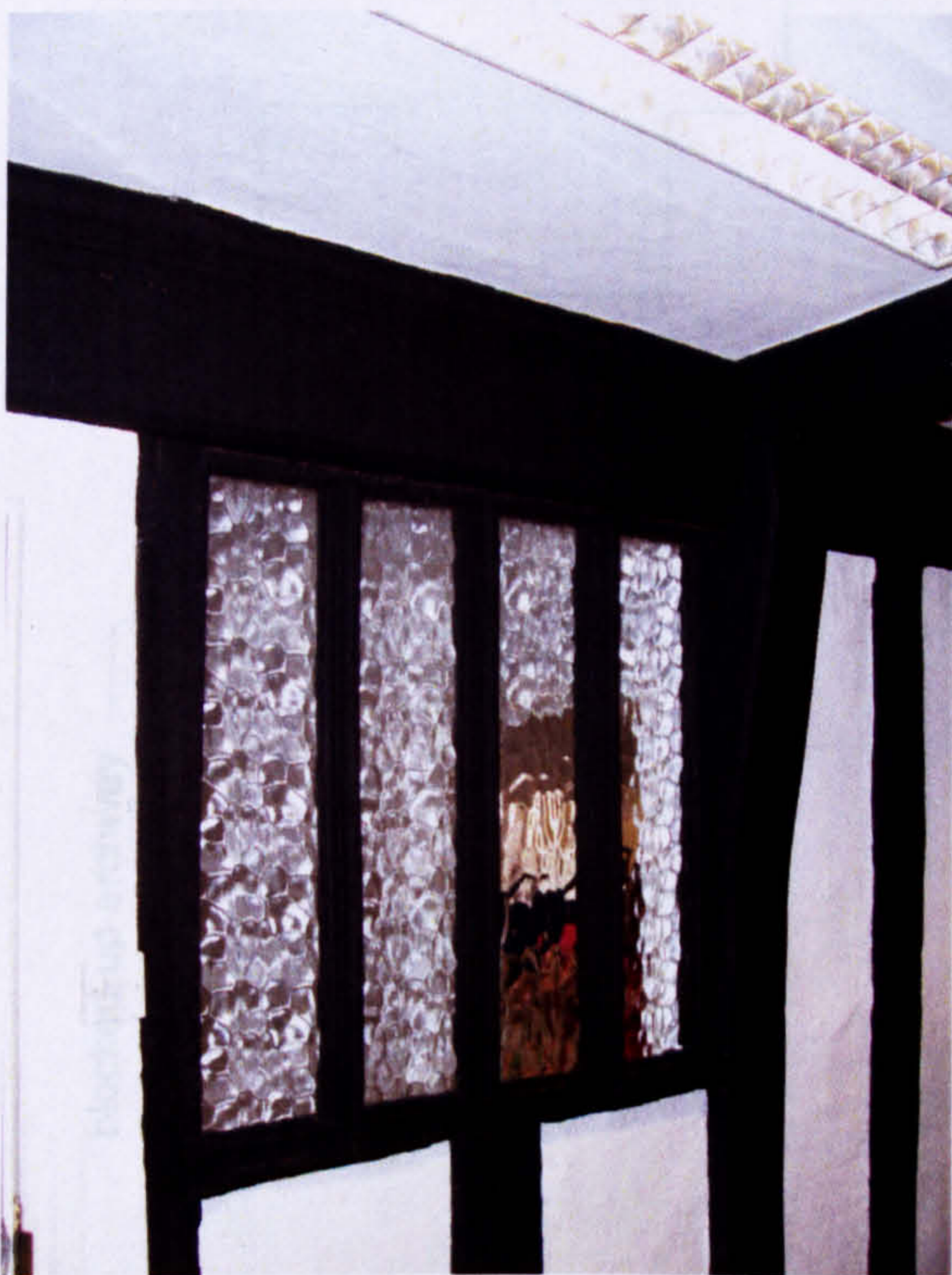
Fig. 24. 15 Bedford Street: mullioned window, north wall.
