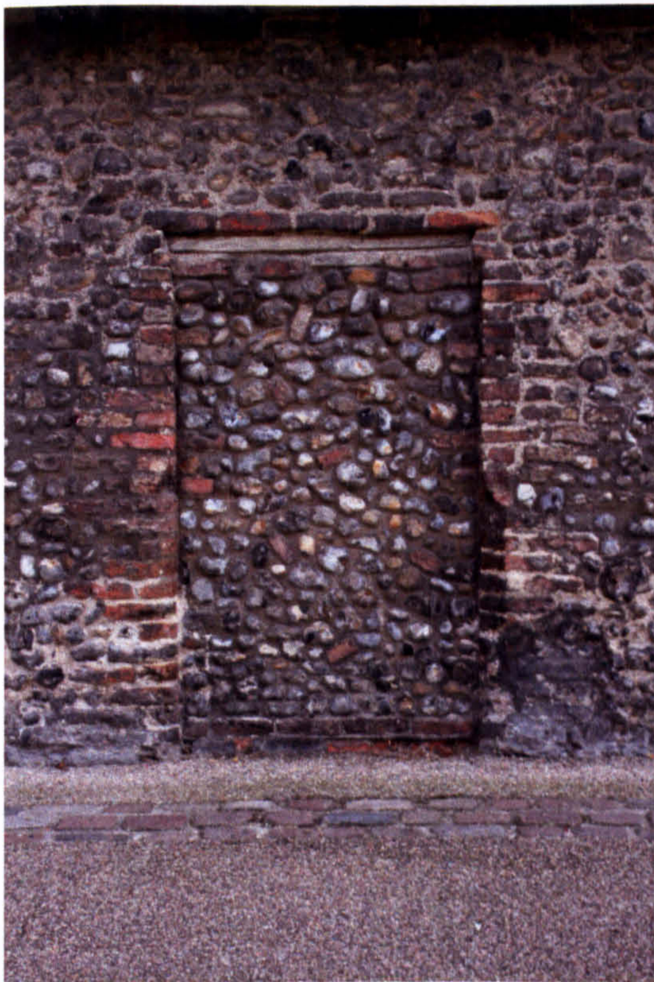
Fig. 48b. 2 Gildencroft: blocked-up ground-floor doorway.
