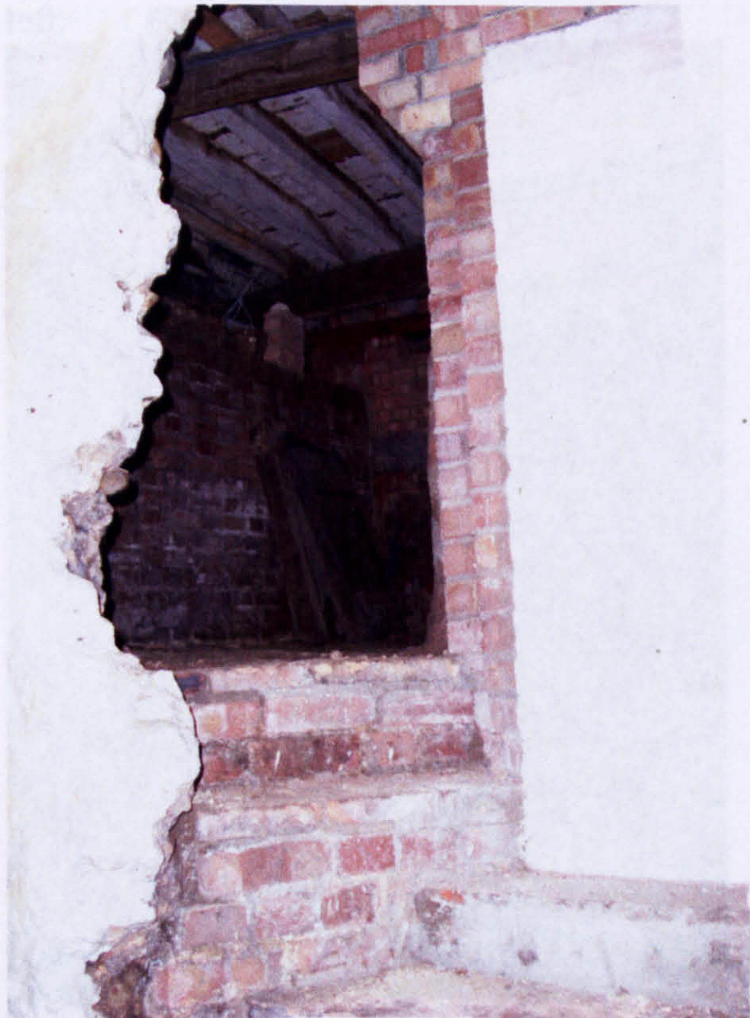
Fig. 27. 15 Bedford Street: view from undercroft entranceway into cellar 2.
