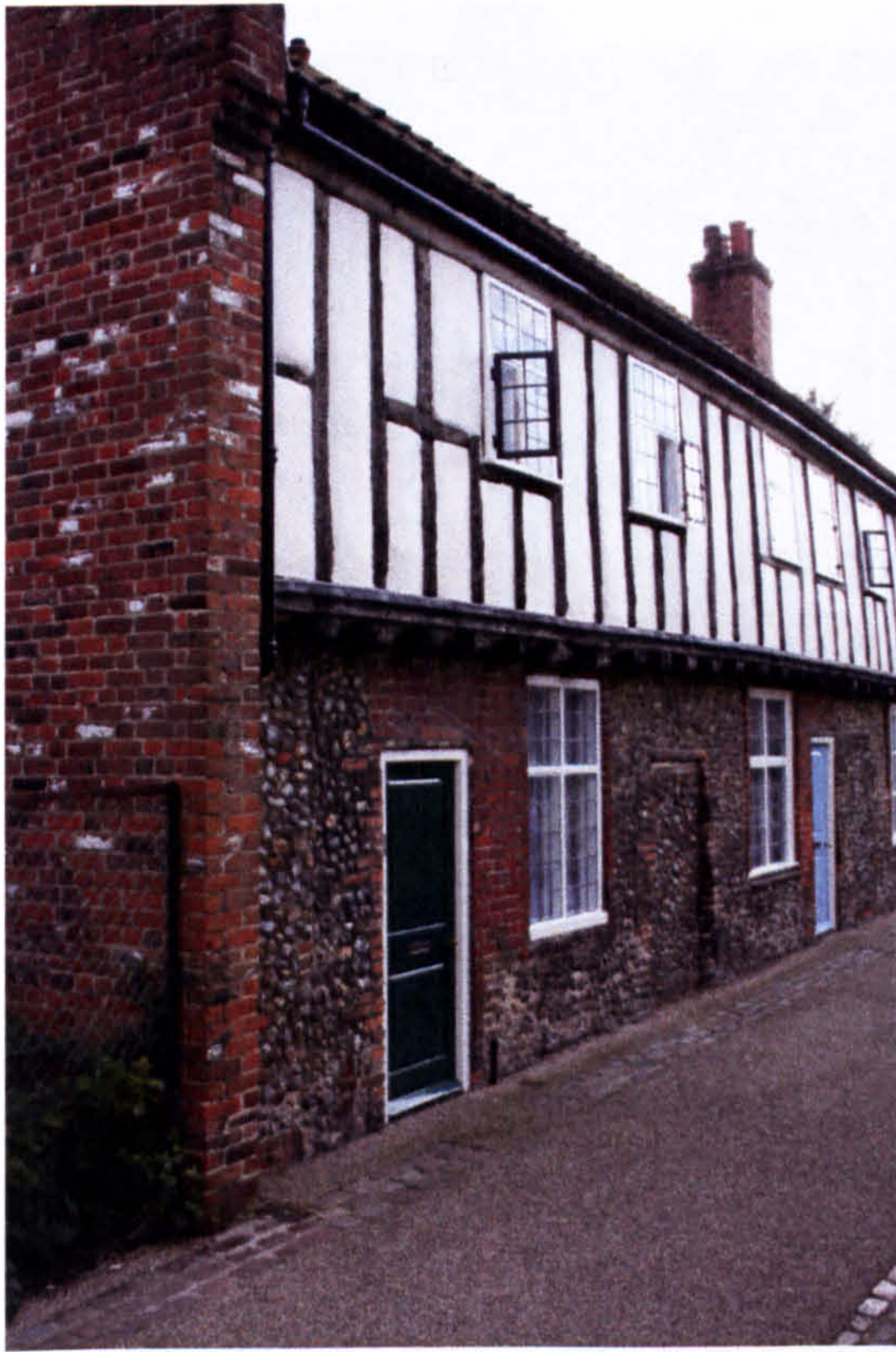
Fig. 48a. 2 Gildencroft: current and blocked-up ground-floor doorways.
