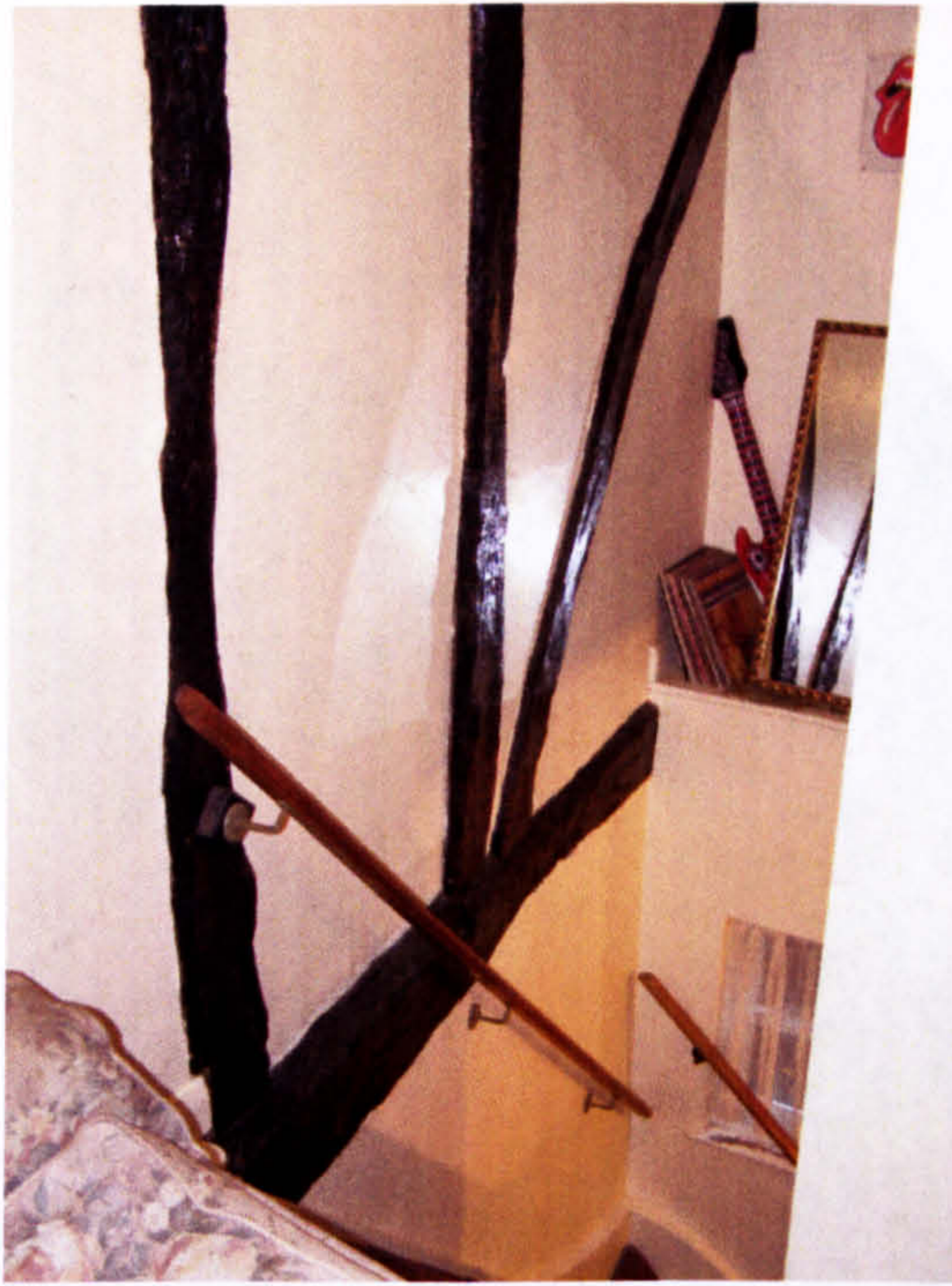
Fig. 86. 1 All Saints' Lane: first-floor level, east truss.
