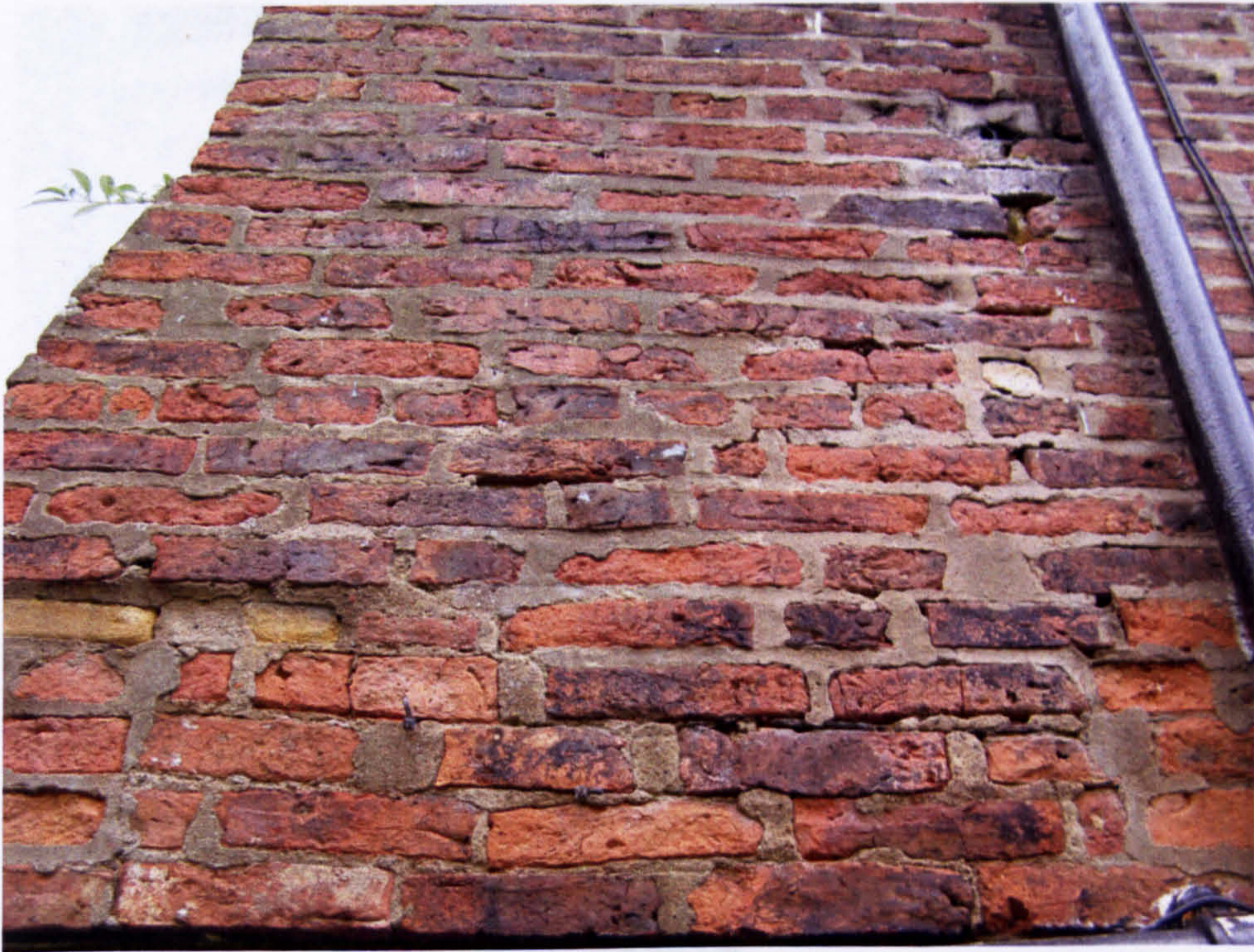
Fig. 63b. 68 Goodramgate: detail of brickwork on west wall at first-floor level.
