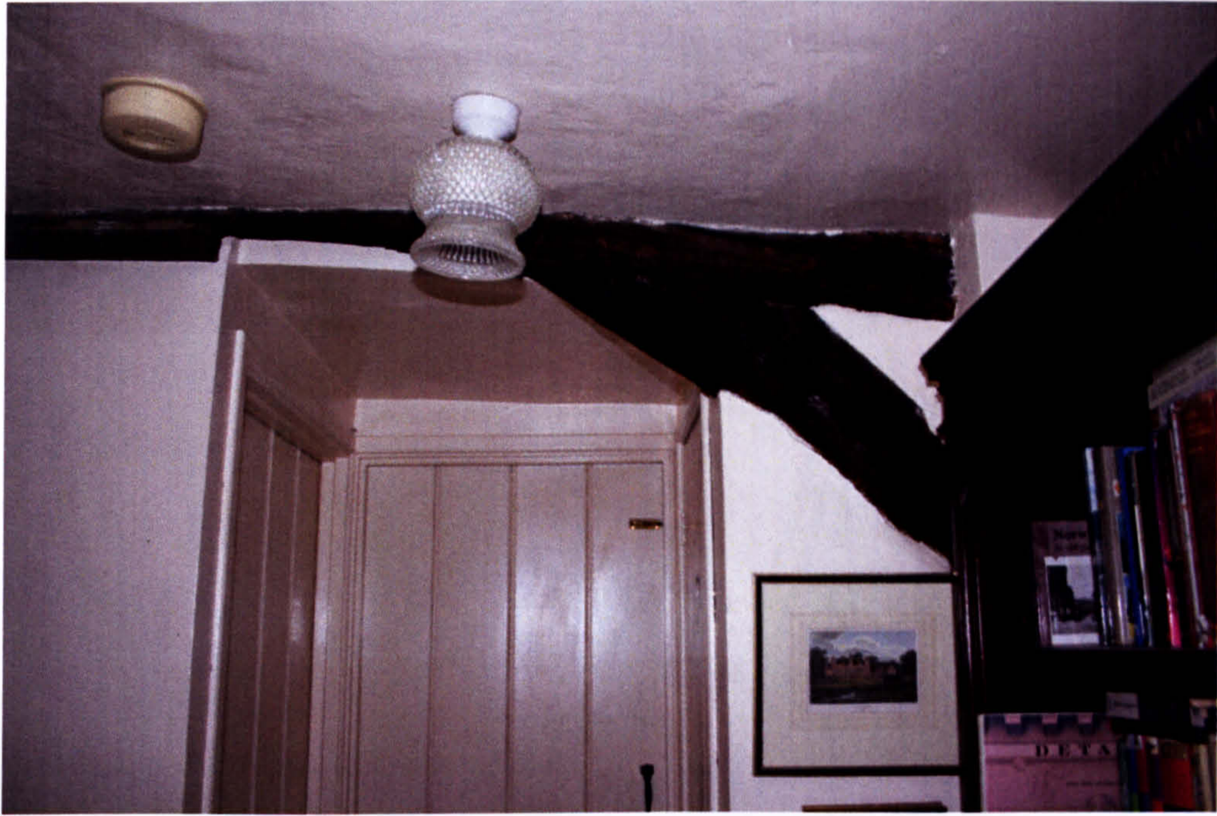
Fig. 58. 10 Gildencroft: first-floor level, central truss.
