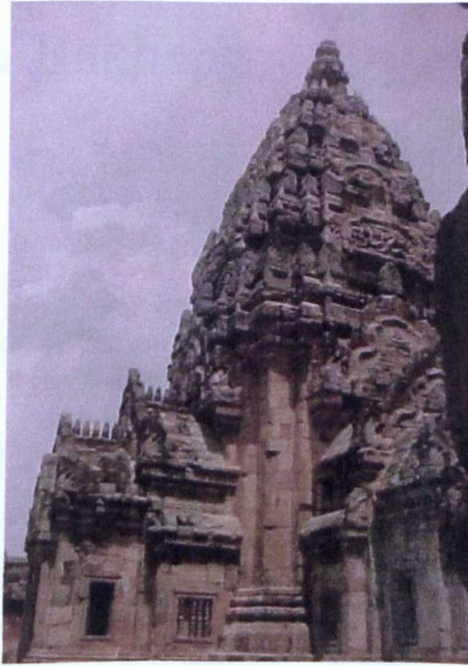
Figure 1.1: The Principal Tower of the Phimai Complex after anastylosis restoration, 1964-1969. (in June 2000)
