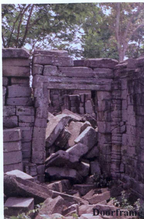
Figure 1.35: Door jamb composed of stone blocks (Banteay Chmar in 2002)
