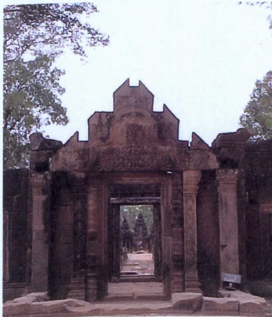
Figure 1.22: Evidence of wooden beam inserted in gable (Banteay Srei in 2002)
