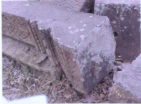
Tenon at the bottom of a shaft (Falling column in Banteay Srei in 2002)
