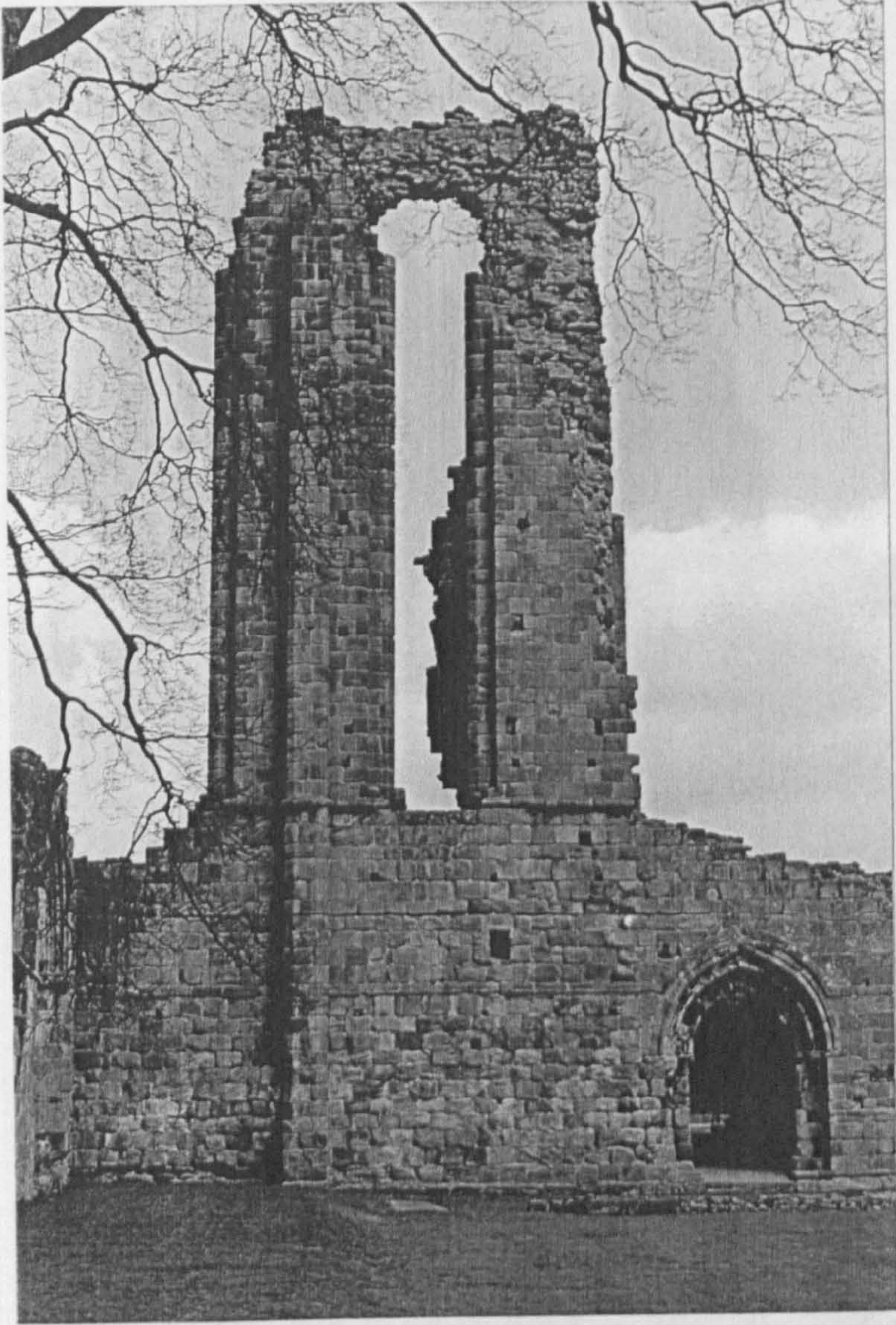
Figure 86: South transept west wall, external.
