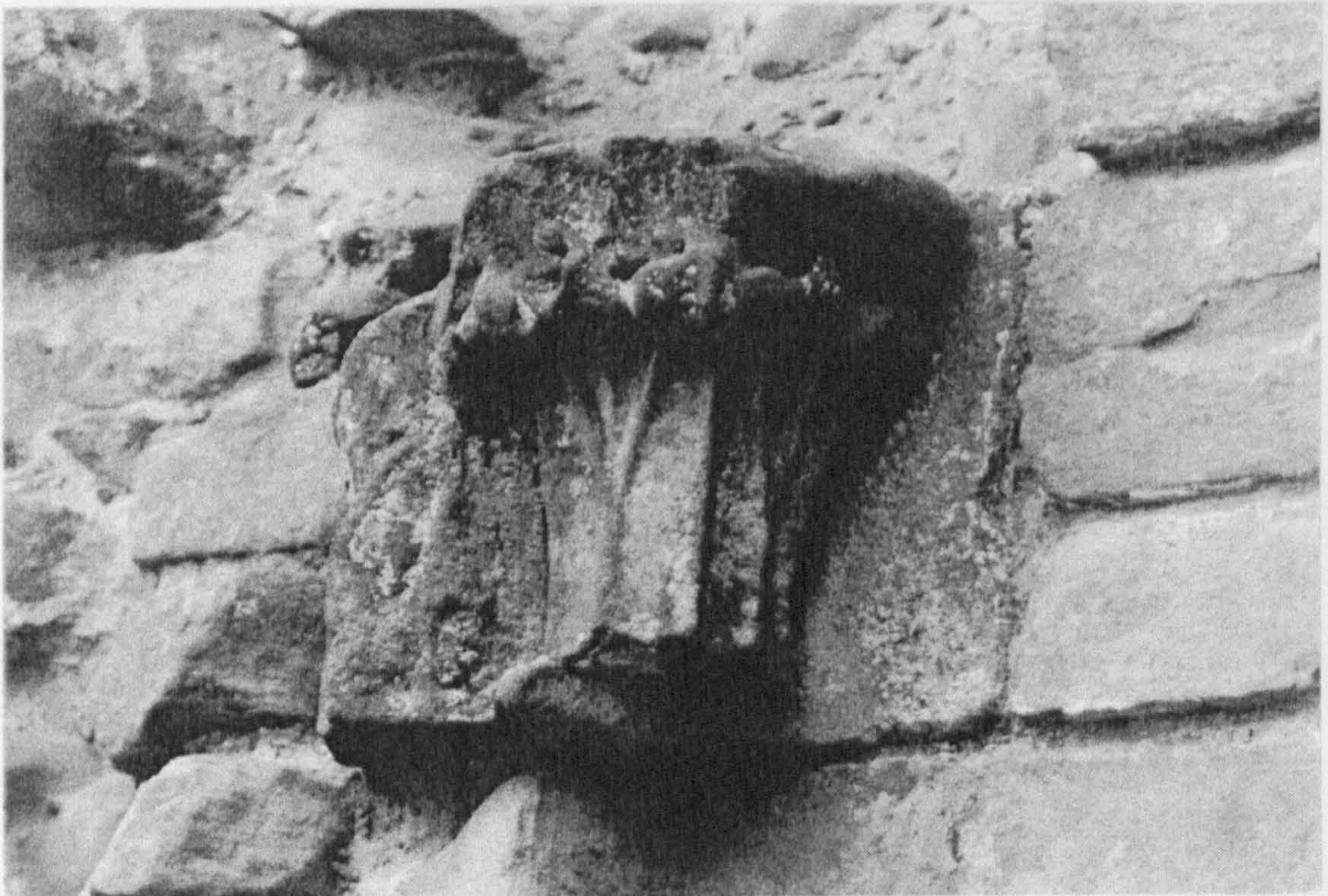
Figure 53: Chapter house, south-west vault respond capital.
