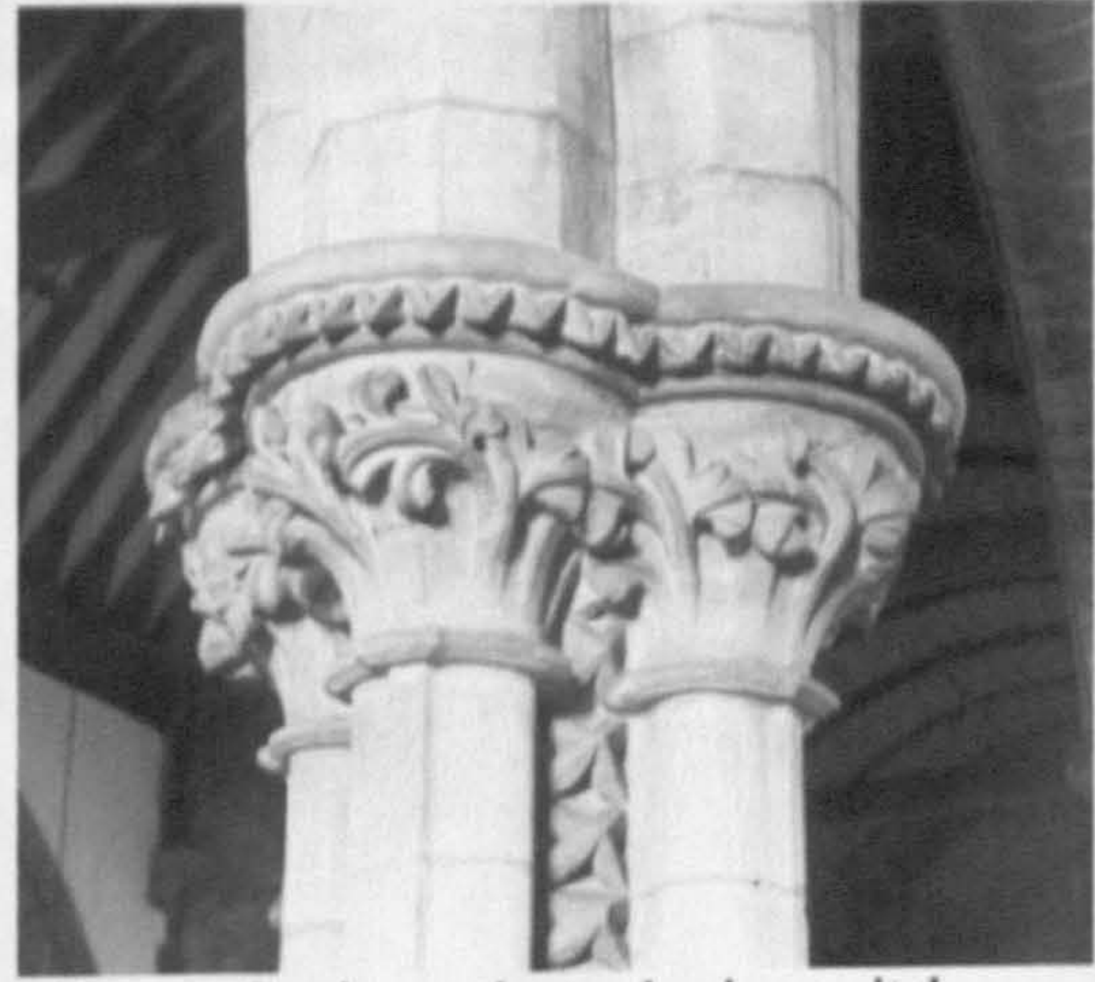
Thornton Curtis, south arcade pier capital
