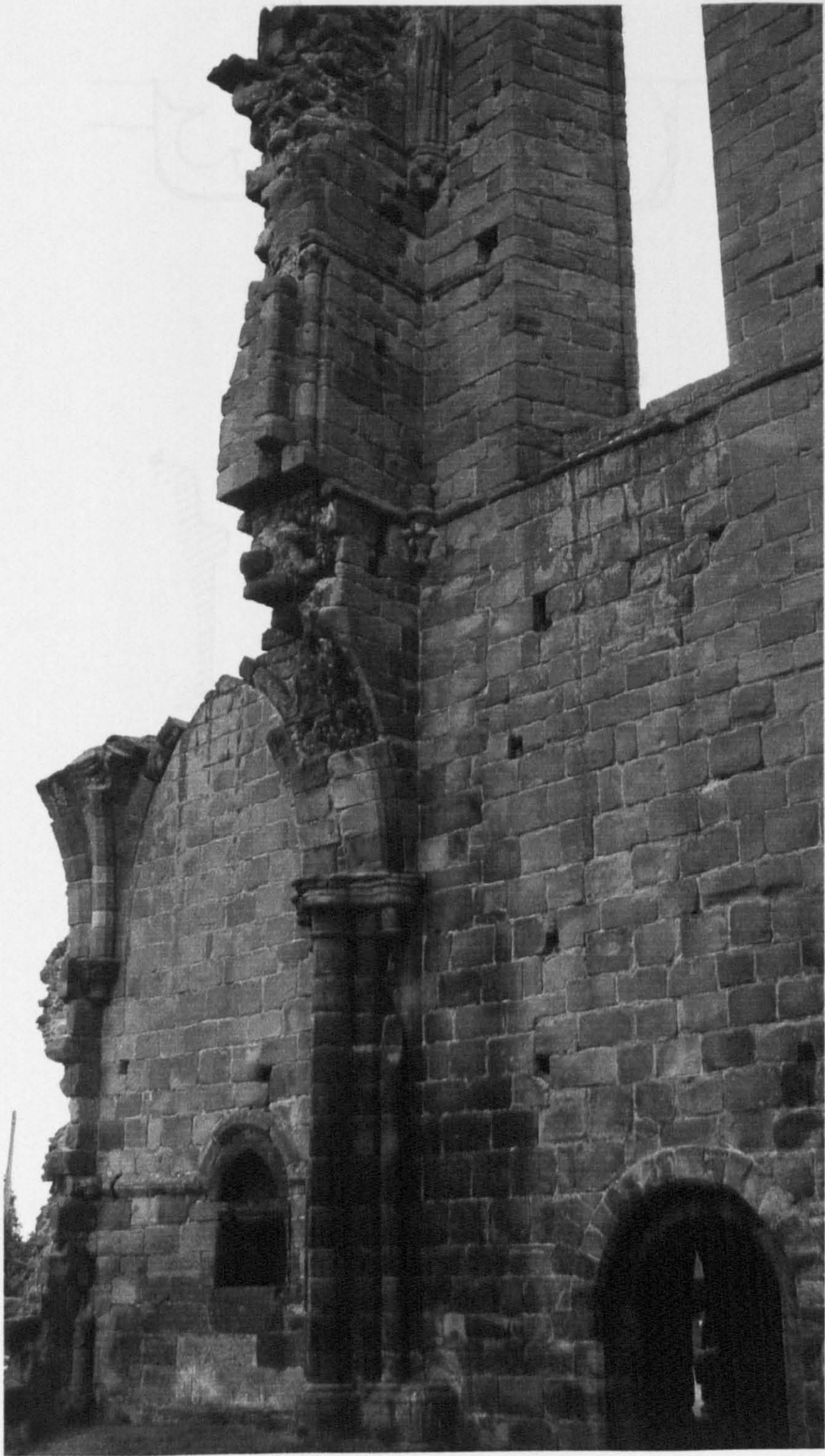
Figure 90: South-east corner of south transept, showing stub of arcade and triforium.
