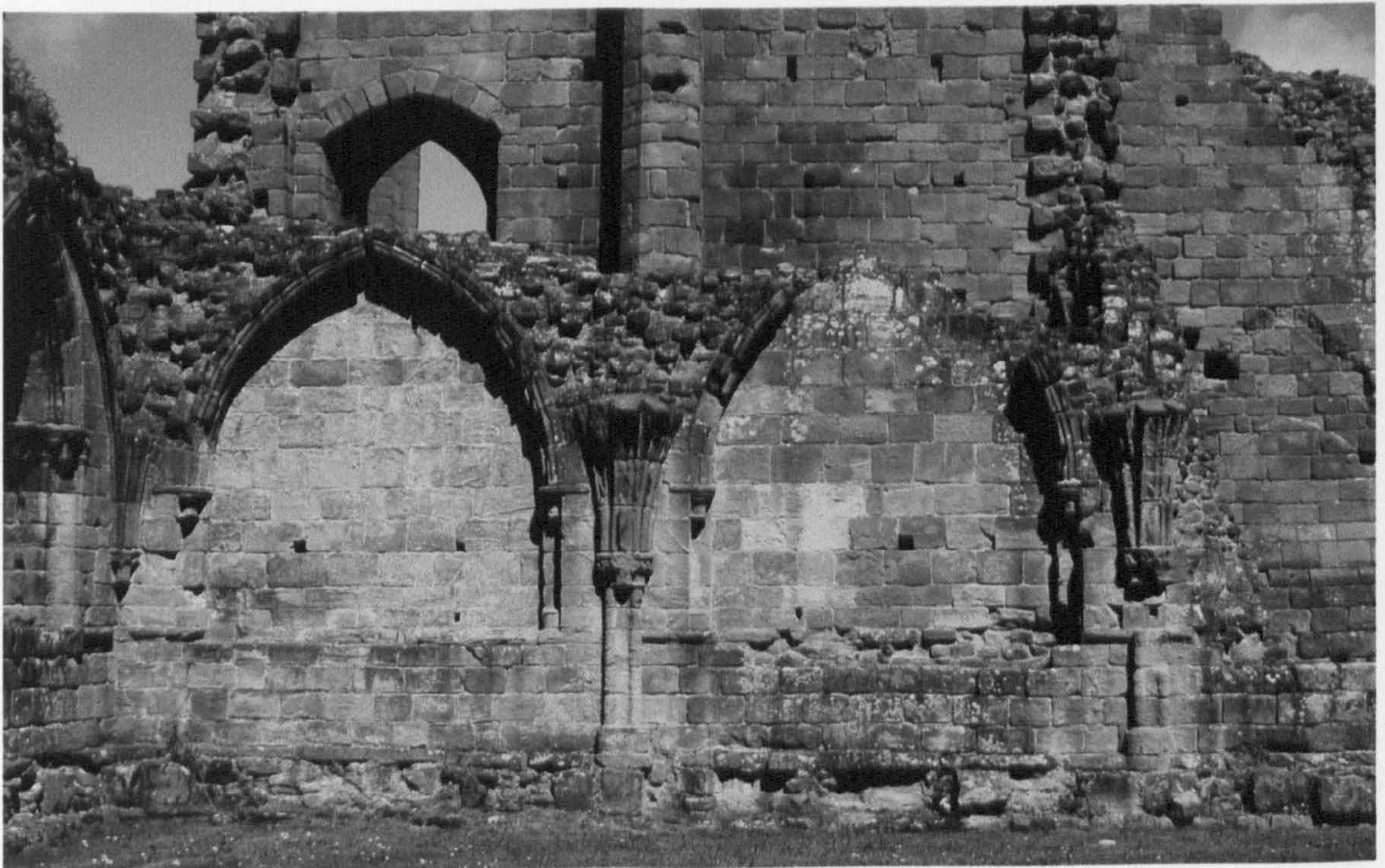
Figure 51: Chapter house, north wall, internal.
