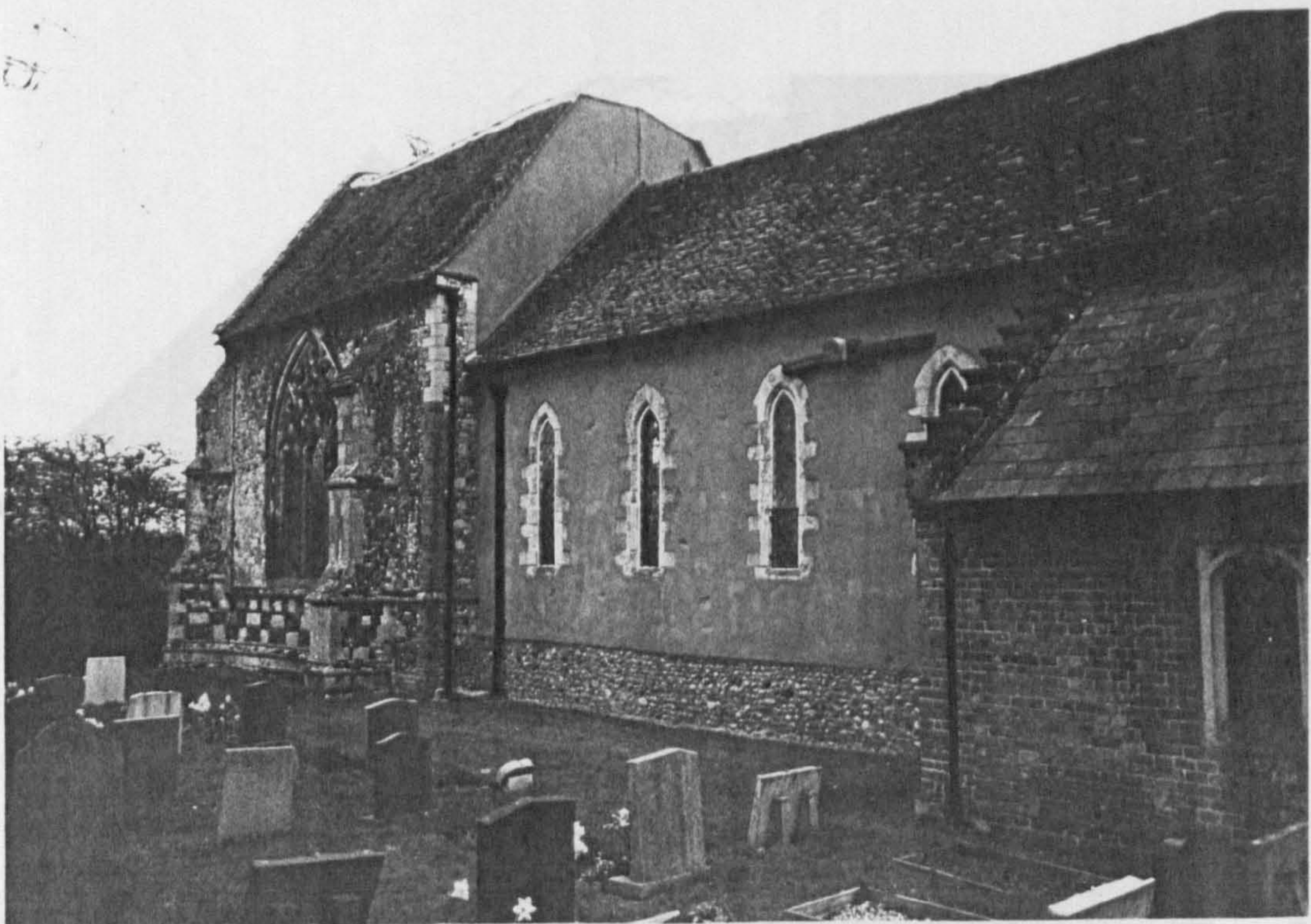
Figure 26: Tilty gatehouse chapel from north-west. The fourteenth-century chancel can be seen on the right side. (Photo: Bob Hall).
