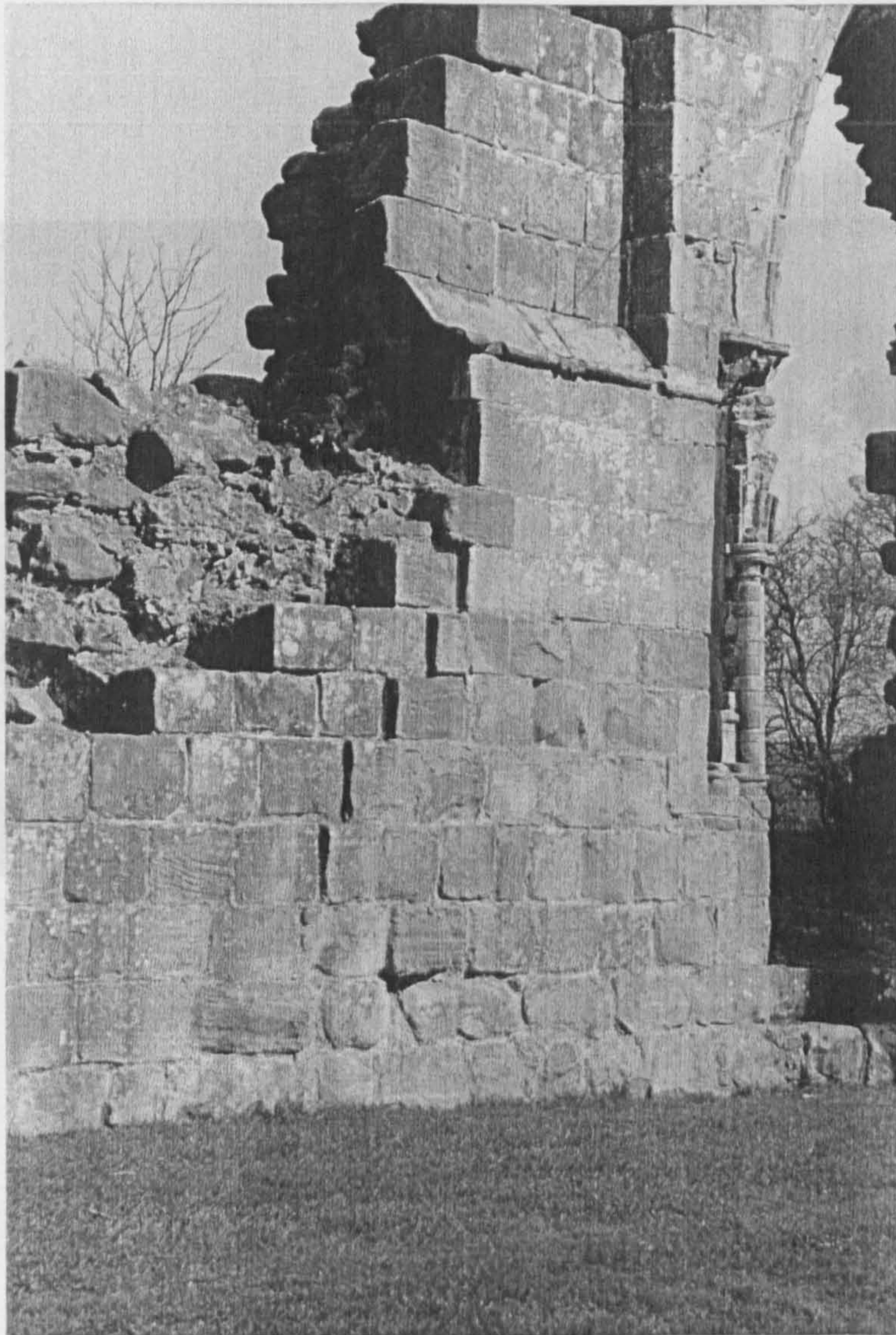
Figure 34: Wall to west of processional door, showing misalignment of ashlars.
