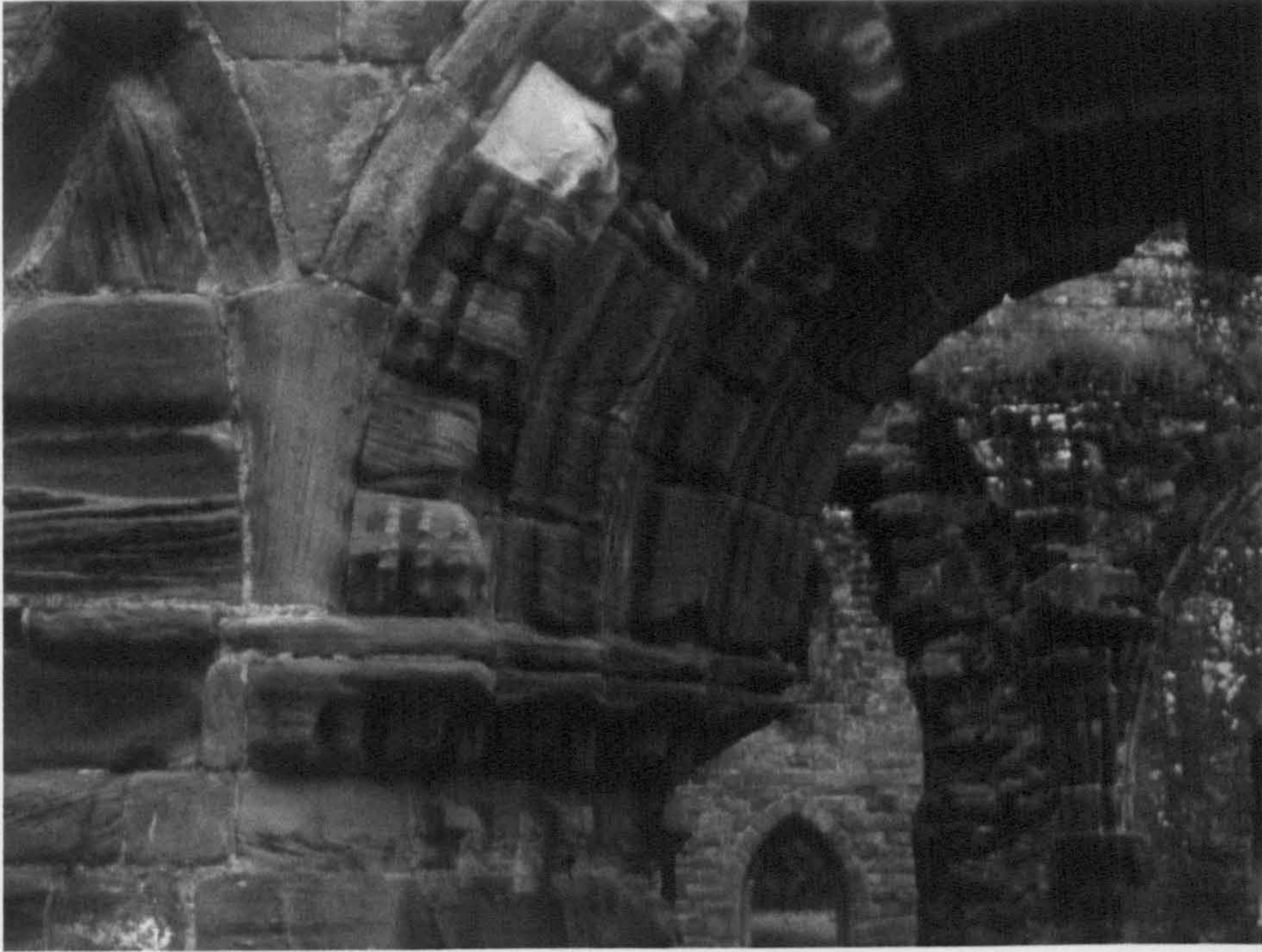
Figure 62: Furness Abbey, parlour doorway, detail.
