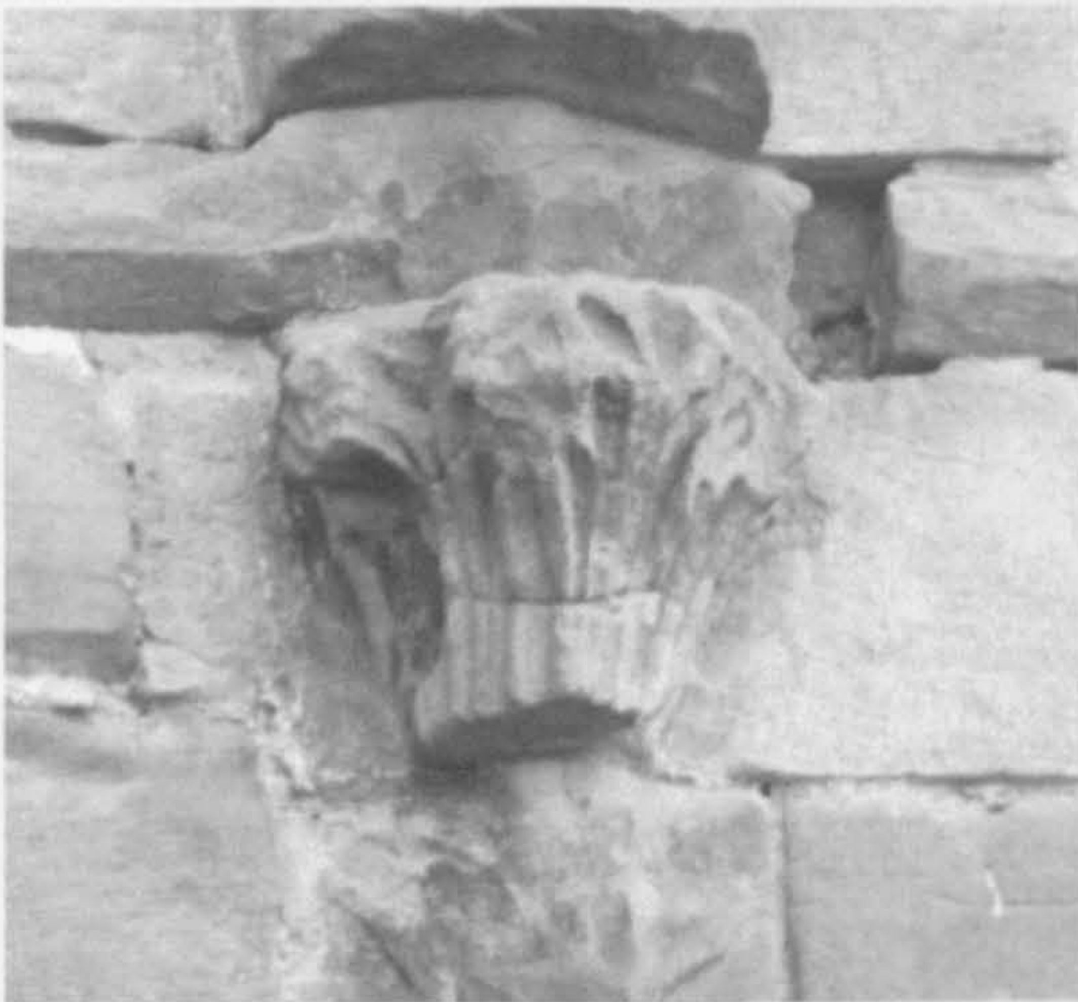
Croxden, corbel in west wall of south transept
