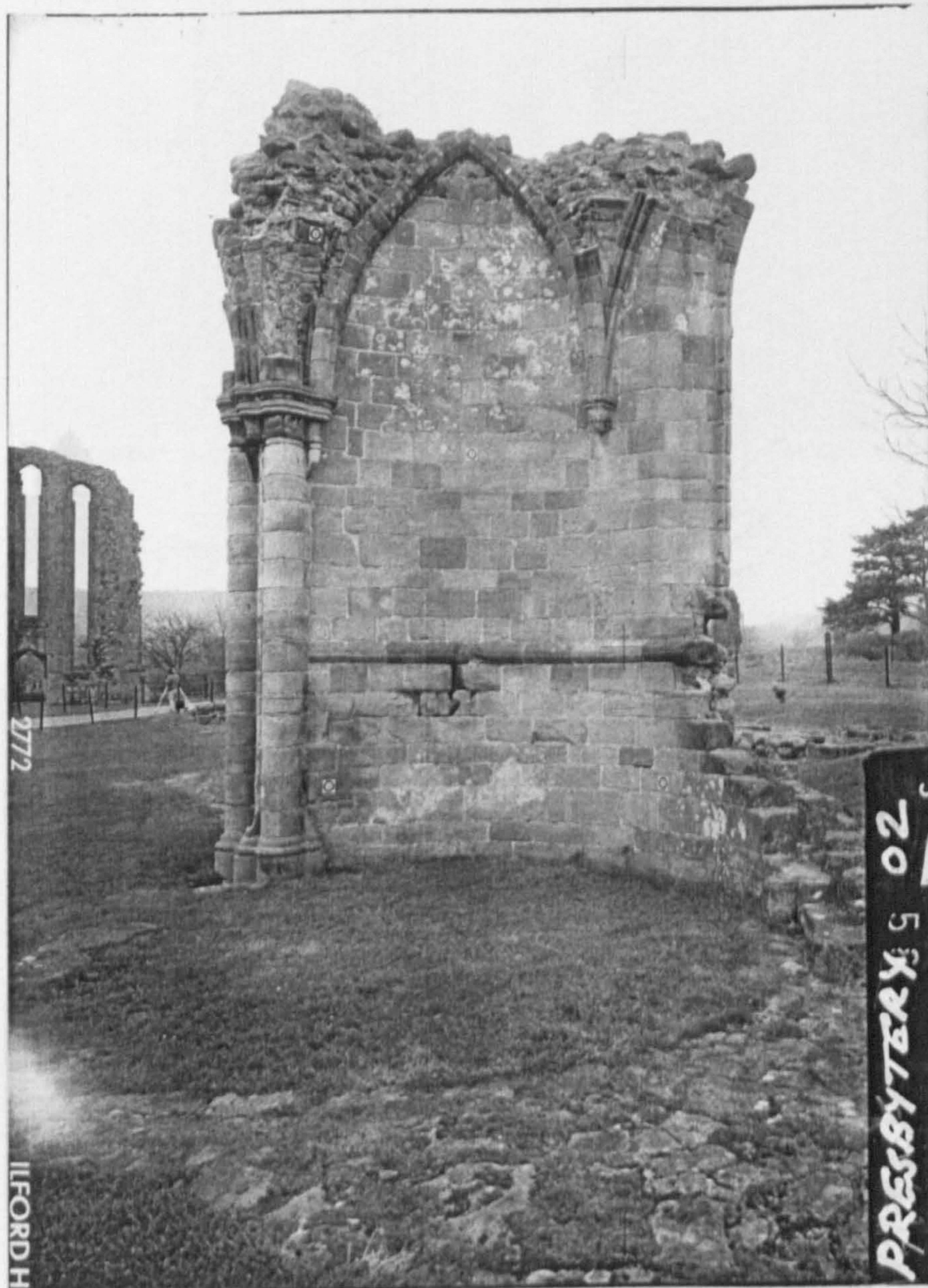
Figure 100: North chevet chapel, looking west. (Courtesy English Heritage).
