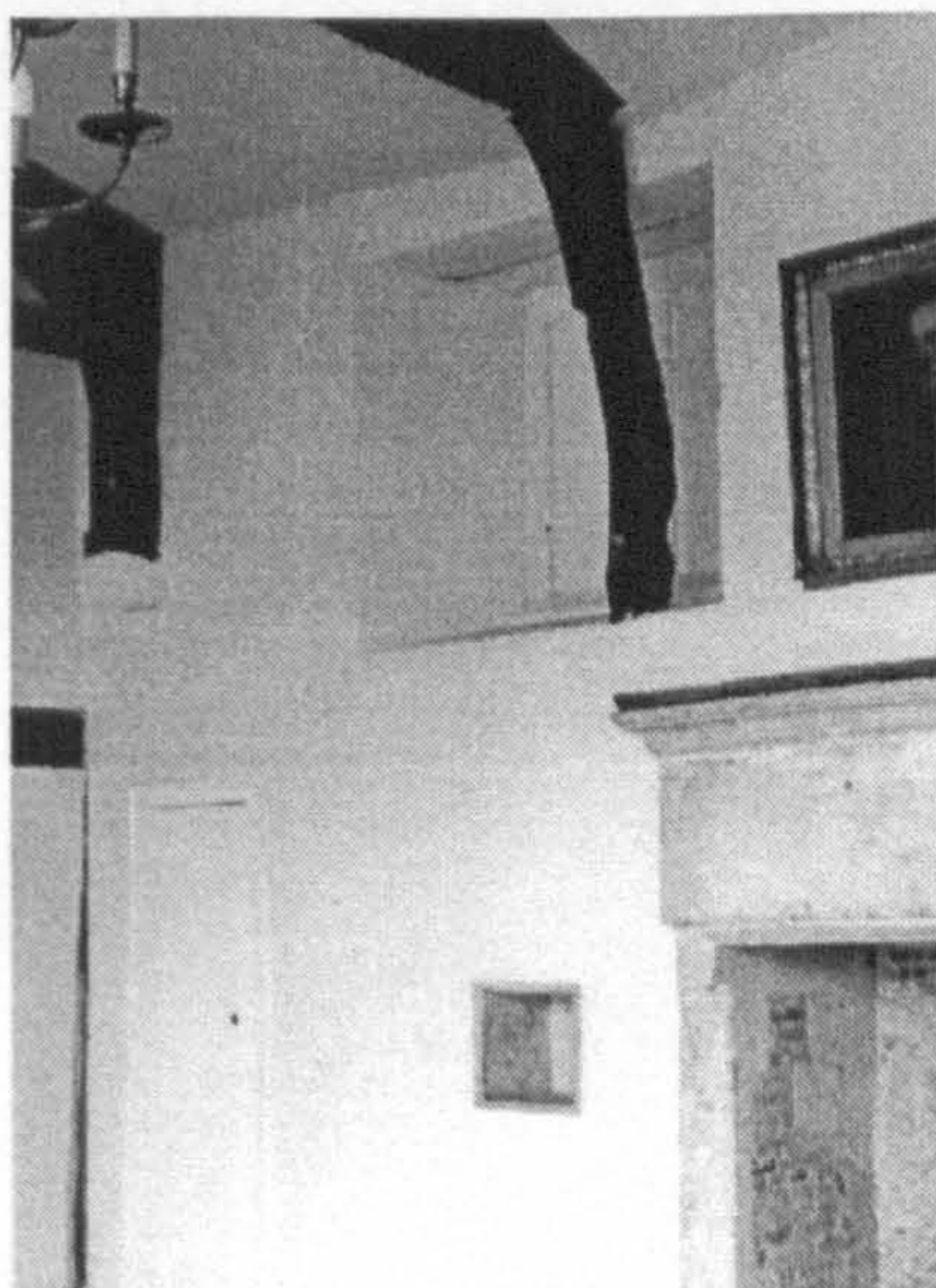
Fig. 206. Inserted window in the east wall of the Henry Room, necessitating the removal of a post and corbel for truss VI
