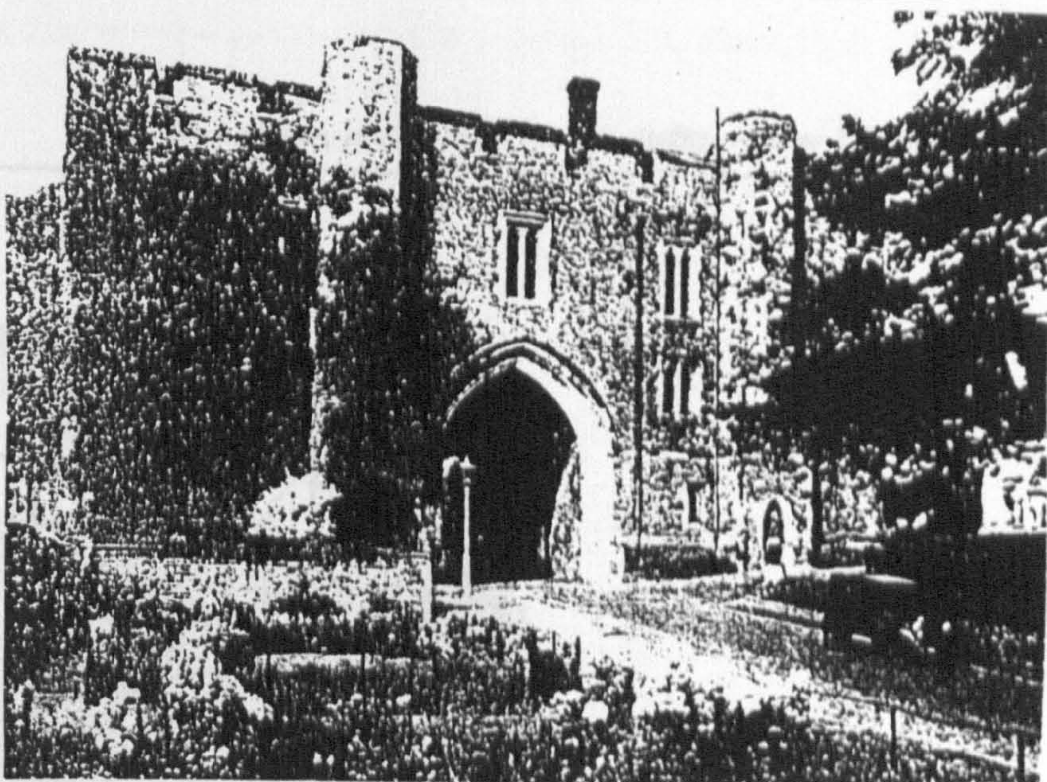
d. St Albans, great gatehouse, inner facade, fourteenth century (Watkins 1934, 33)
