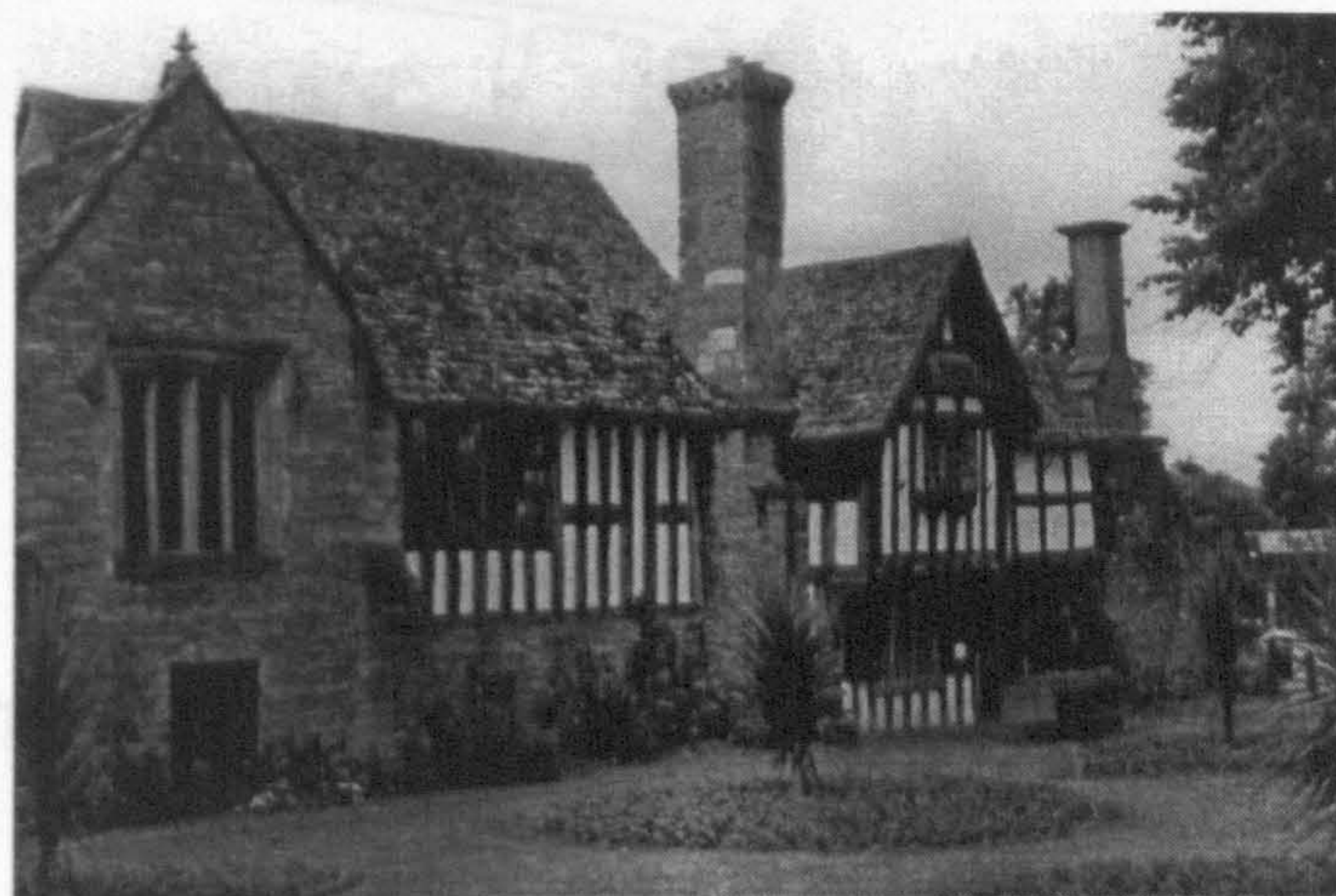
f. Evesham, view of the almonry, outer facade, facing southwest
