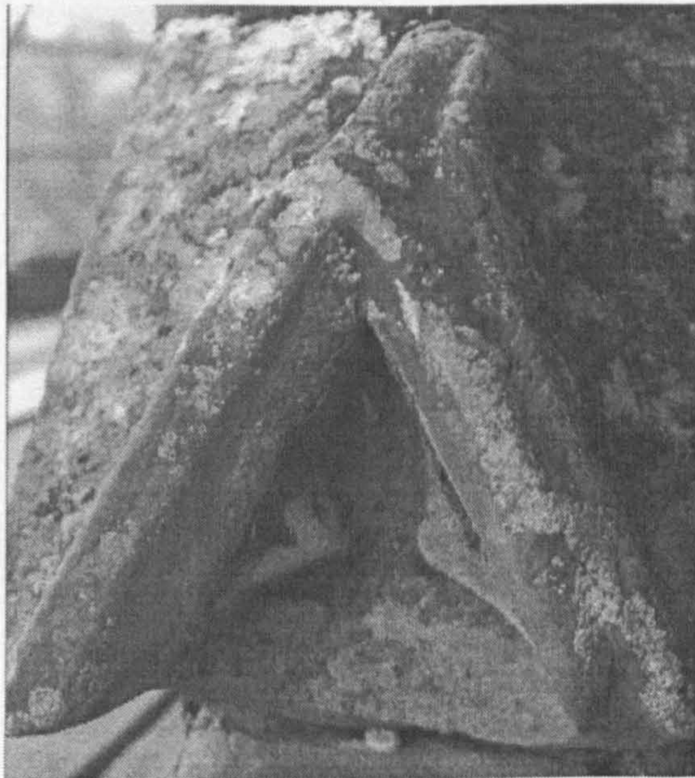
Fig. 137. Porch, gable window 2347 (internal), recut sill
