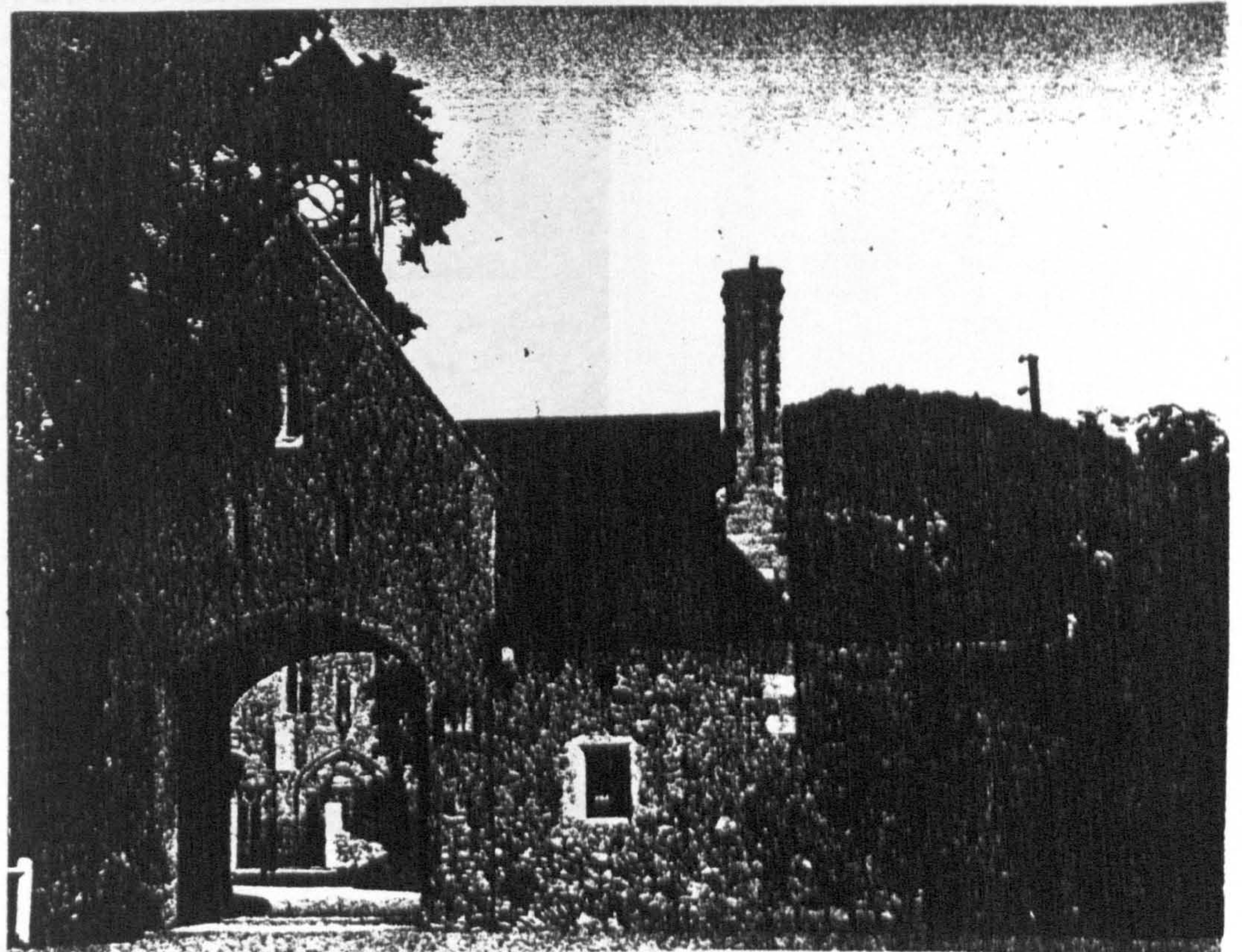
b. Beaulieu Abbey outer gatehouse, outer facade, early thirteenth century (Hope and Brakspear, 1906b, facing 142)
