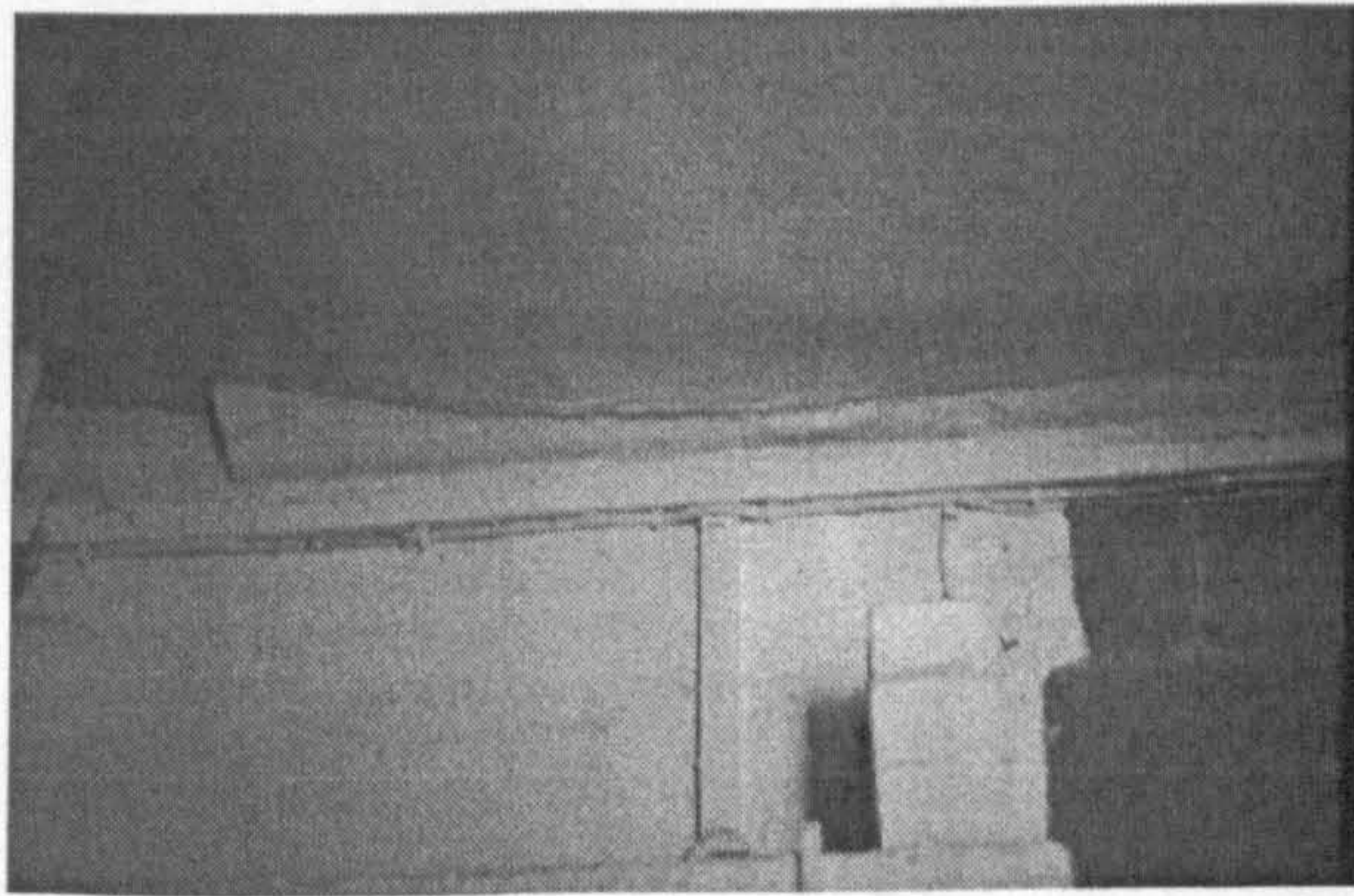
Fig. 131. Corbelling supporting first-floor doorway into hall
