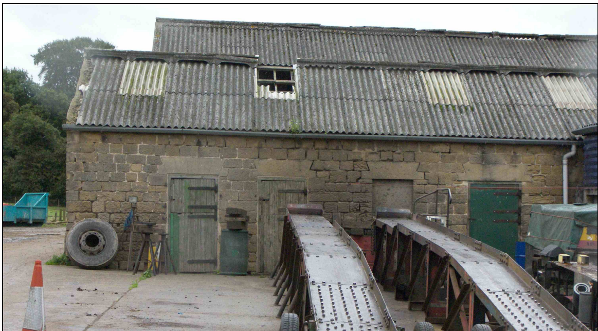
4.17 False voussoirs in the lintels of the stables at Lofthouse Grange Farm. This arrangement did not become a part of the local vernacular architecture until the final quarter of the eighteenth century.
