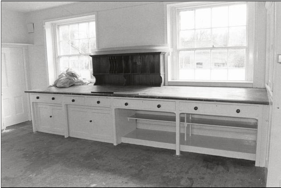
6.9 Office in the west of the workshop, facing south. It is unlikely that the desk is original (Lane 2008, reproduced courtesy of Scott Wilson Ltd)
