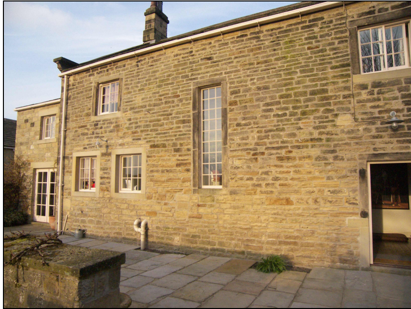
7.3 The rear elevation of Stables Farmhouse with a symmetrical layout. The doorway to the right has been extended from a former fenestration, while those on the ground floor in the left of the elevation have been inserted in the twenty-first century. A moulded kneeler is visible on the gable end.
