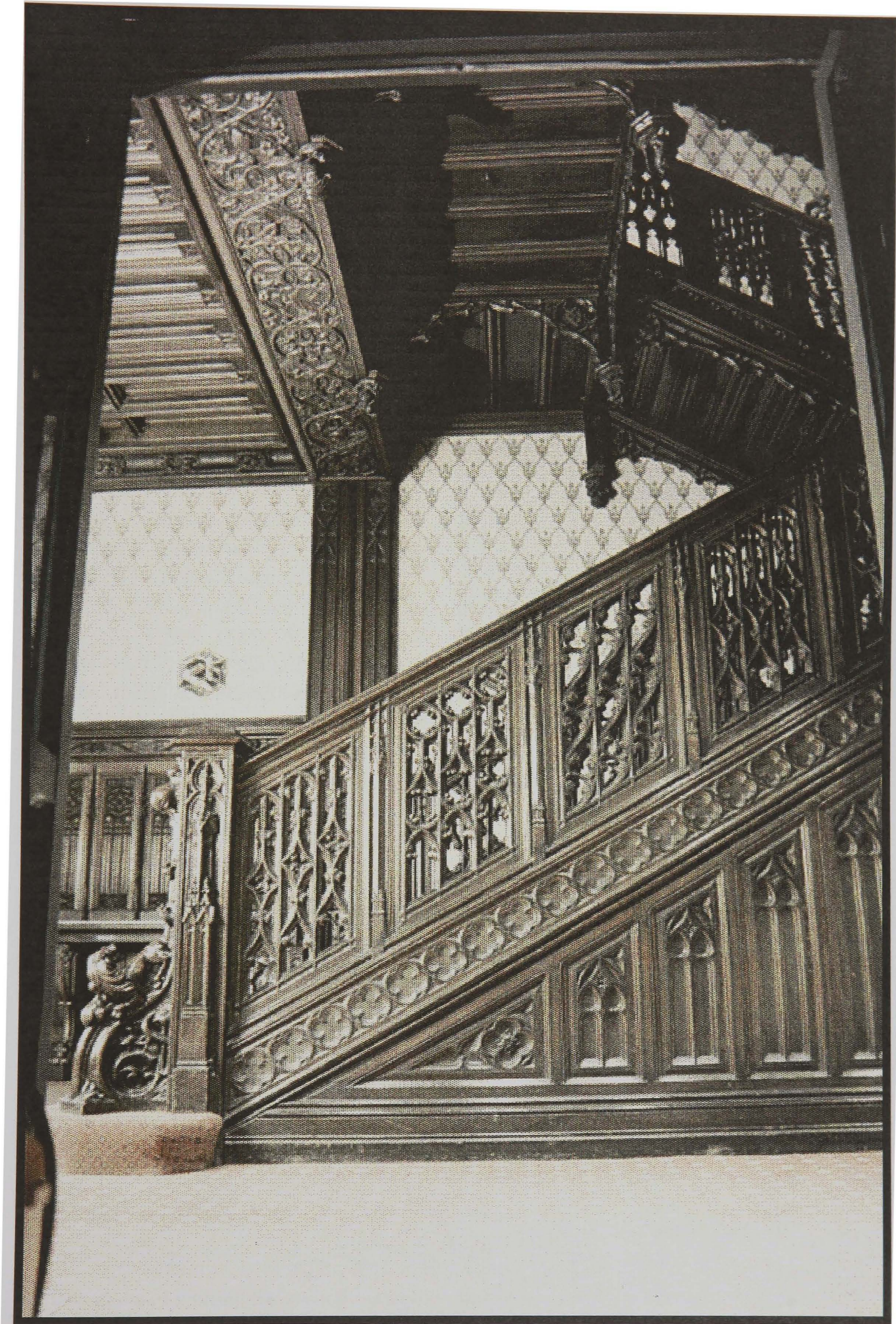
1206 - artists unknown No.46 Grosvenor St., Gothic Staircase (c.1904) (wall coverings - new).
