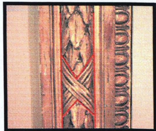
218 - Bèlanger Bagatelle, Salle à Manger, jamb detail in wood (red denotes carver's sections) writer's photo.
