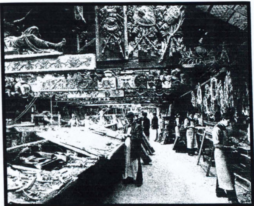
233 - Jackson & Sons "View of a Workshop for Making and Mounting Carton-Pierre and Composition Ornaments on to Wood or Plaster", historical photograph, NMR.
