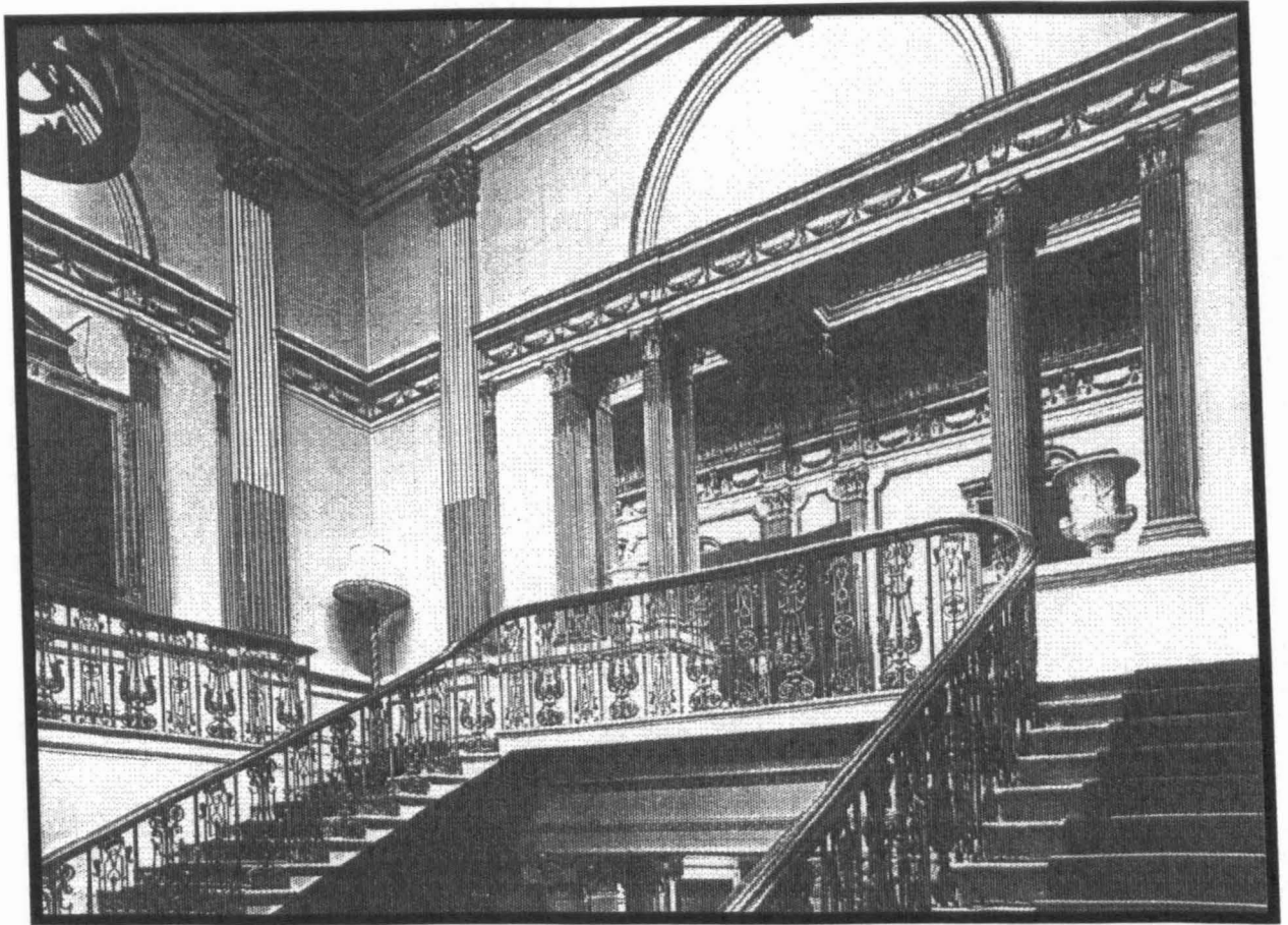
192 - B. D. Wyatt Londonderry House, Upper Staircase Hall, H. Felton (July 1962) NMR AA62/7580.
