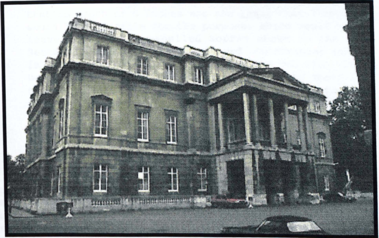
301 - B. D. Wyatt with R. Smirke Stafford House entrance façade, writer's photo.
