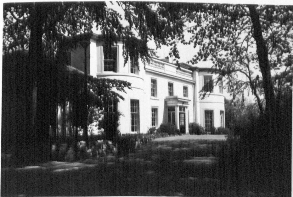
Photograph 27. GRANGE HOUSE, CHAPEL ALLERTON.
