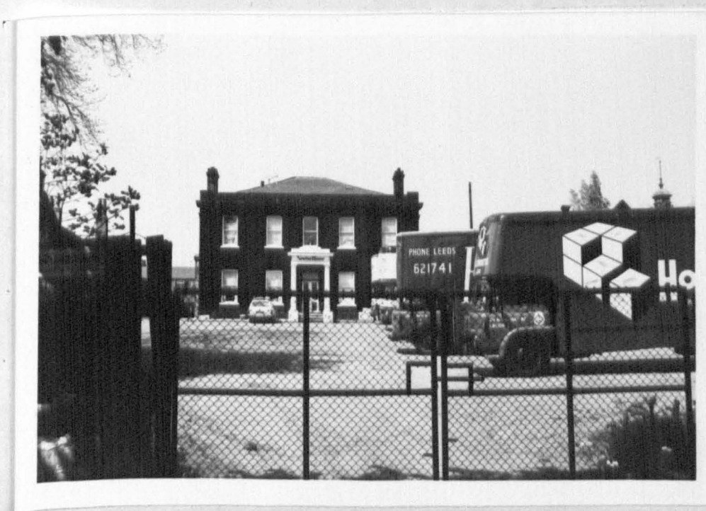
Photograph 8. NEWTON HOUSE, Spencer Place, c.1834 for H. GRESHAM, pawn-broker. (S.i.).
