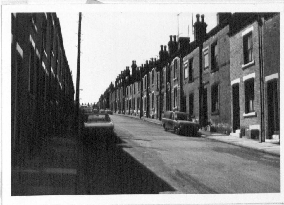
Photograph 23. NORTHBROOK STREET, through houses, 1876-. Plots were still unbuilt on in 1897.
