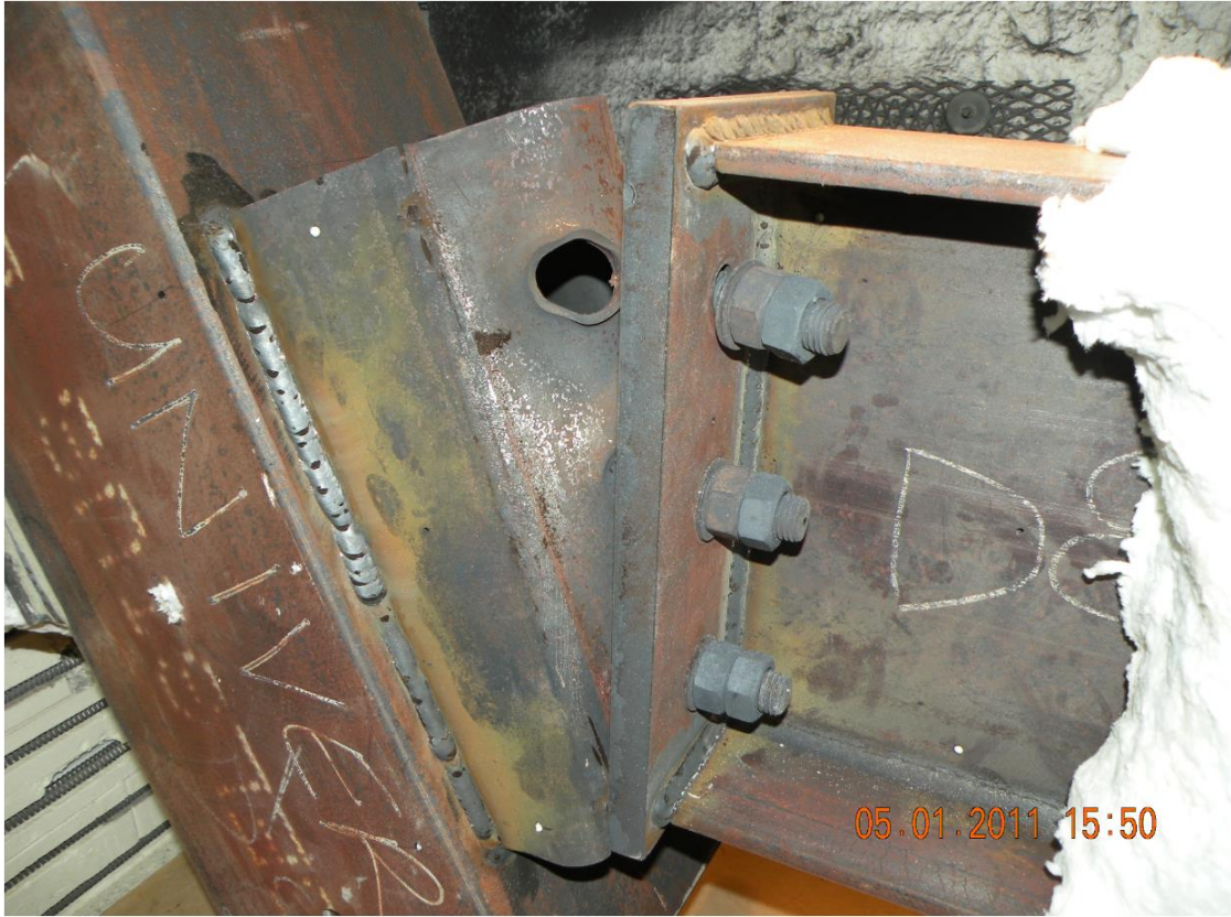
Figure 173: SCFT-RC200_550_55_04-01-2011 side view 2 after test
