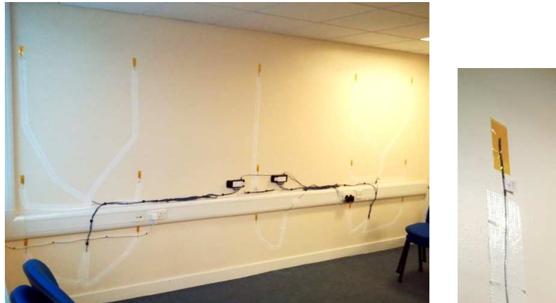
Figure 5.17 Internal view of the observed wall with green wall test beds (first floor). The ends of internal thermocouples were covered by Kapton (thermal insulating) tape in order to minimise the influence of the indoor ambient air temperature.
