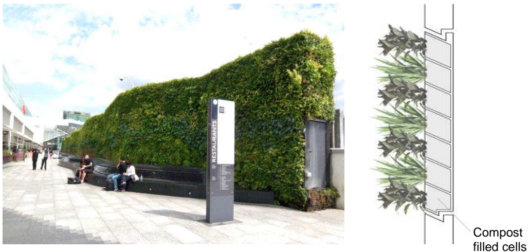
Figure 2.10 A 170-meter long living wall at Westfield Shopping Centre in London made up of more than 5,000 compost-based modules and 200,000 individual plants (left). Sectional drawing of a typical modular panel encasing organic substrate in individually divided cells (right)
