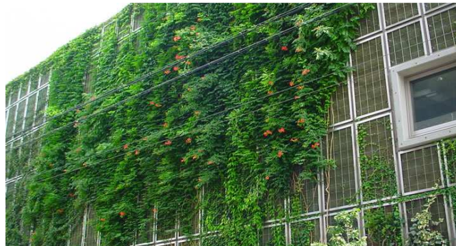
Figure 2.7 The green façade of the Chikusa theatre in Nagoya, Japan. Panels made of wire and fibrous foam are mounted on the external walls to ensure sufficient foliage cover across the three-story building (2012)
