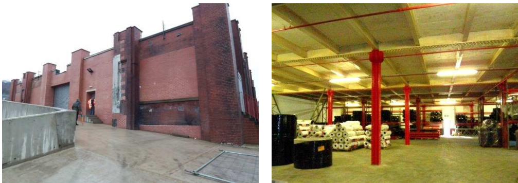
Figure 4.4 Exterior and interior views of the monitored building (2010)
