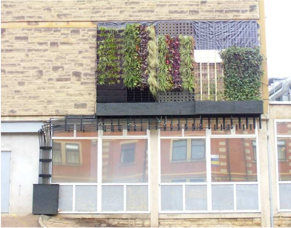
Figure D- 5 The test beds on completion (2012)
