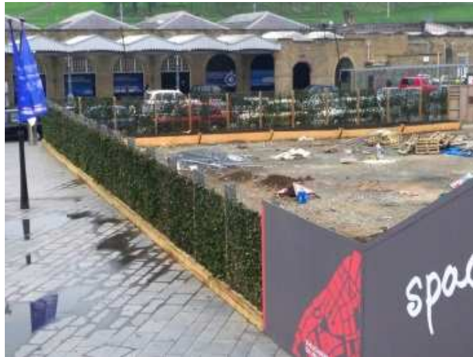
Figure 7.3 Ivy screens installed at Shef square shortly after the installation (April 2010)
