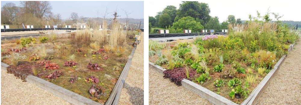
Figure 4.3 Monitored green roof in April (left) and August 2012 (right)
