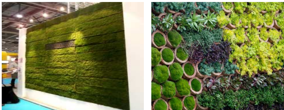
Figure 2.14 'Moss wall' exhibited at Ecobuild London, green moss is grown on the panels made of compressed recycled plastic (left, 2011), and a green wall exhibited at the Chelsea Flower Show designed to require little irrigation by using moss and succulents growing inside terracotta tubes (right, 2013)
