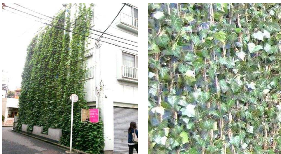
Figure 2.9 Twining climber, morning glory, grown around a vertical wire support structure on a building in Yokohama, Japan (left) and 'green screen' with pre-grown ivy on trellises (right) (2013)
