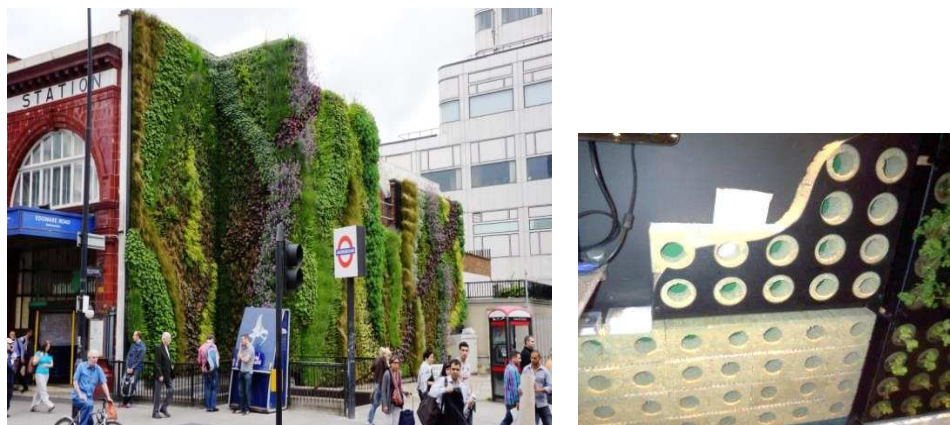
Figure 2.11 Hydroponic living wall installed at Edgware Road Tube Station, London with 14,000 plants of 15 different species (left) (Biotope Ltd 2014) and components of hydroponic living wall panels (right) (2011)
