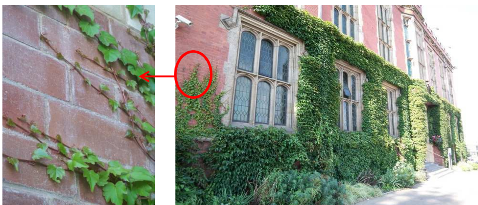
Figure 2.6 Self-climber cover on a building of the University of Sheffield (right) and a close up image of young ivy vines (left) (2009)
