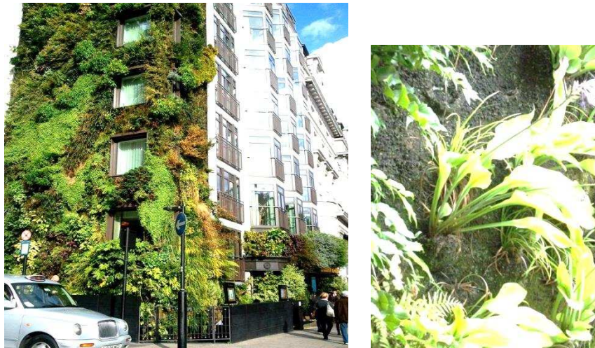
Figure 2.13 Patric Blanc's felt based living wall installed at the Athenaeum hotel in Piccadilly, London. 280 varieties of plants are used to withstand the elements on the exposed eight story wall and create a three-dimensional vertical garden (2011)
