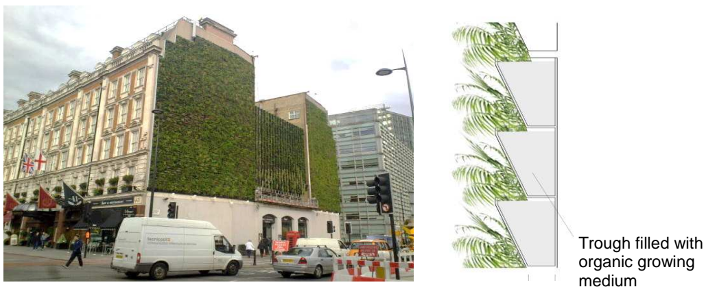
Figure 2.12 Trough system installed on the Palace Hotel in Victoria, London, consisting of 16 tons of compost accommodating 10,000 plants (left) and sectional drawing of a typical trough container system (right) (2013)
