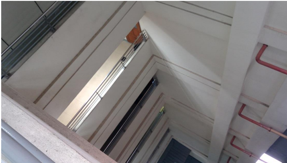
Figure 4.9. Open space between floors in Building B
