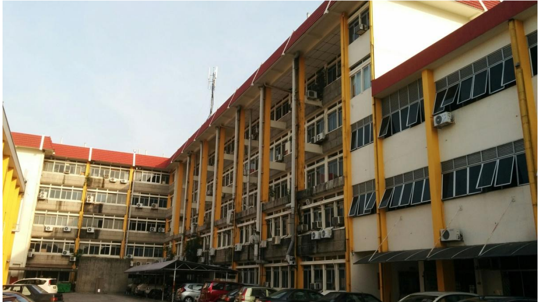
Figure B1.1. Building A
