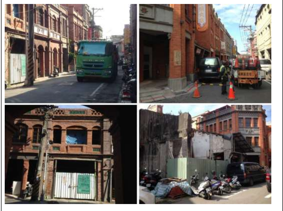
Figure 8.14 Scenes of renovation of buildings on Dihua Street.
