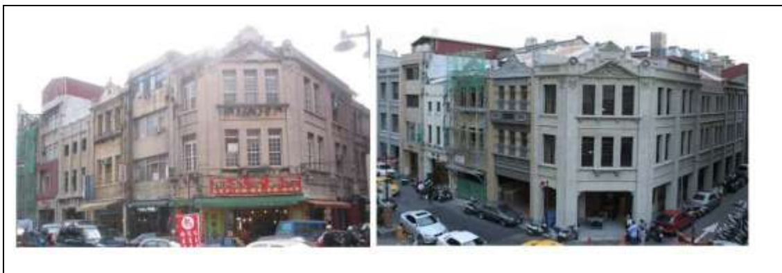
Figure 7.10 Before and after repair and maintenance.
