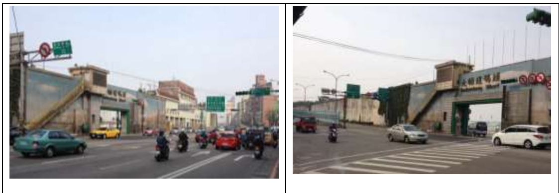
Figure 3.8 The 9.6 meter-high embankment and inter-city-link fast road (Huanhe North Road).
