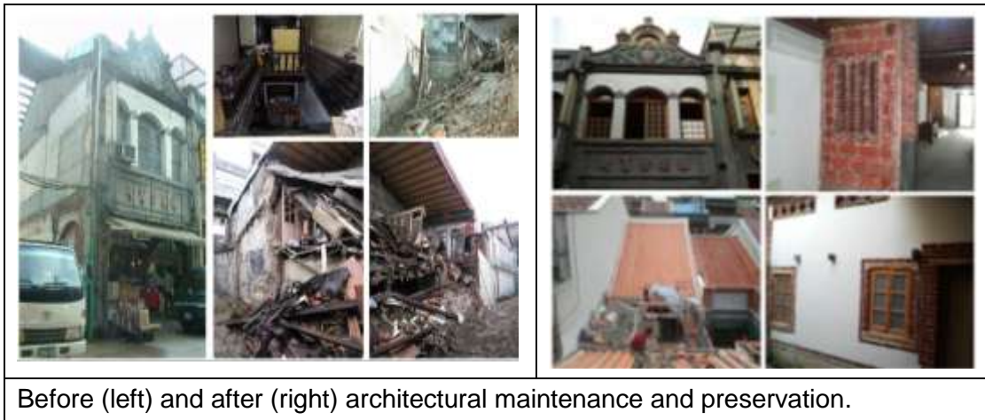
Figure 3.10 No. 117, Dihua Street.
