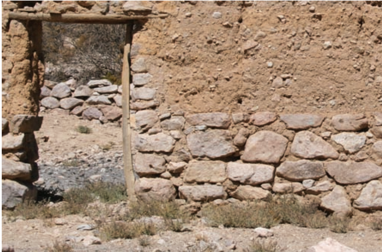
Fig. 3.27 Stone foundations.
