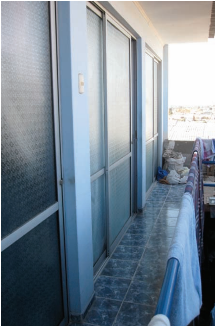
Fig. 5.32 Case 03, view of the rear room volume.
