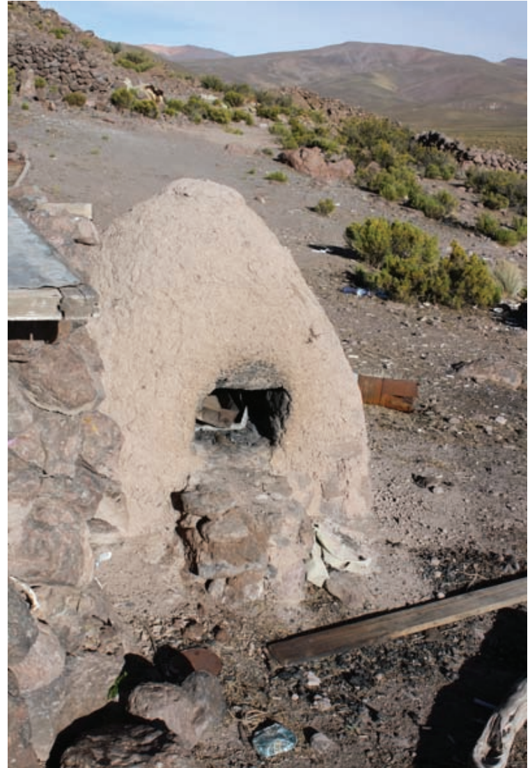
Fig. 3.23 External adobe oven in the patio.
