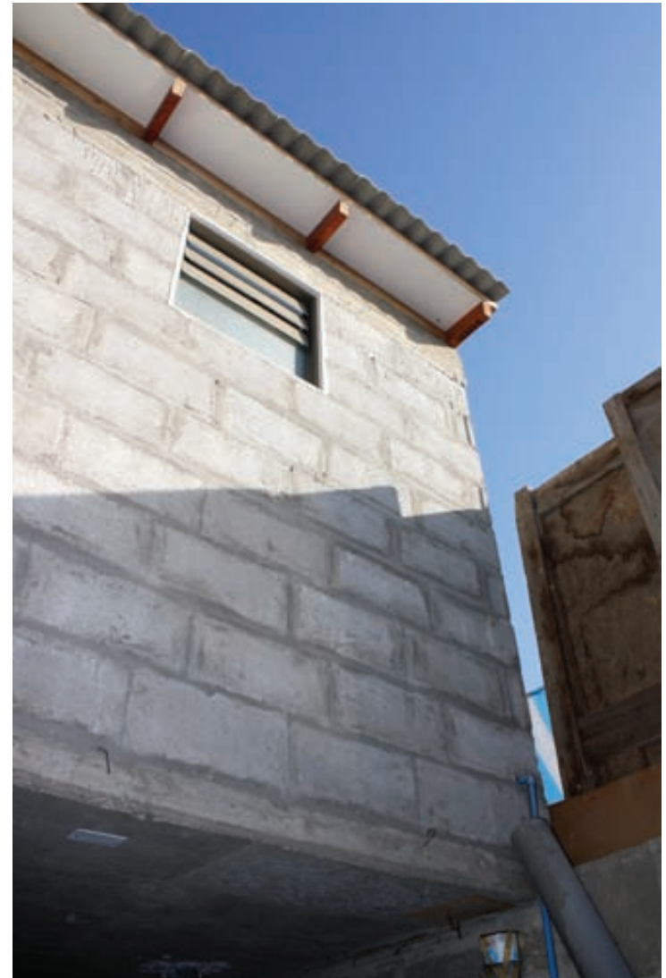
Fig. 5.44 Case 04, structure built on the upper floor.
