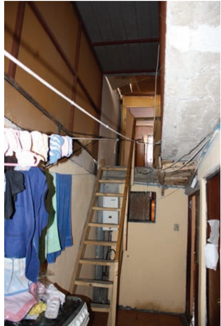
Fig. 5.82 Case 07, wooden staircases.
