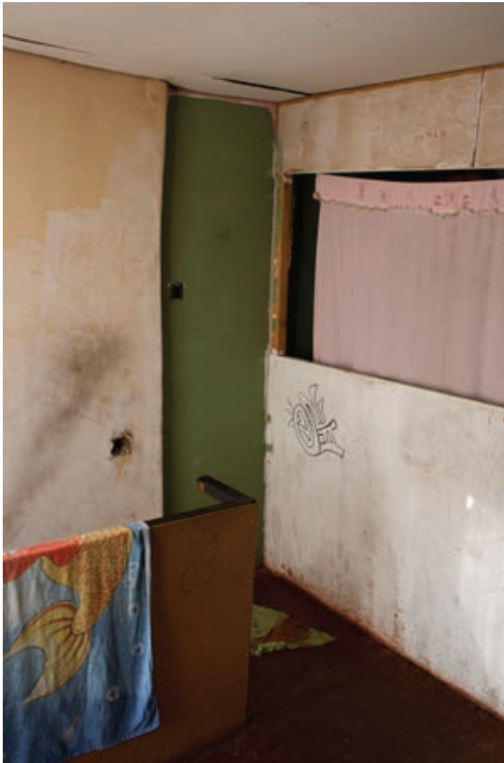
Fig. 5.69 Case 06, upper level rooms separated by light wooden partitions.
