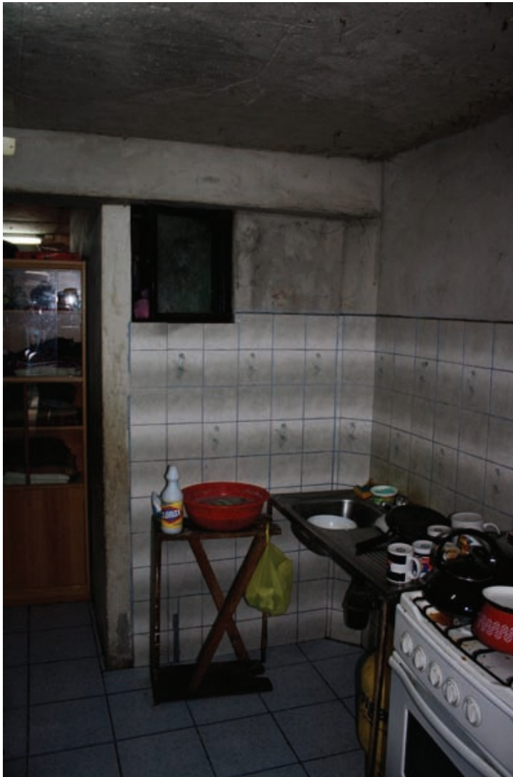
Fig. 5.11 Case 01, original structure bathroom window still exist and open to the new kitchen and dining area.
