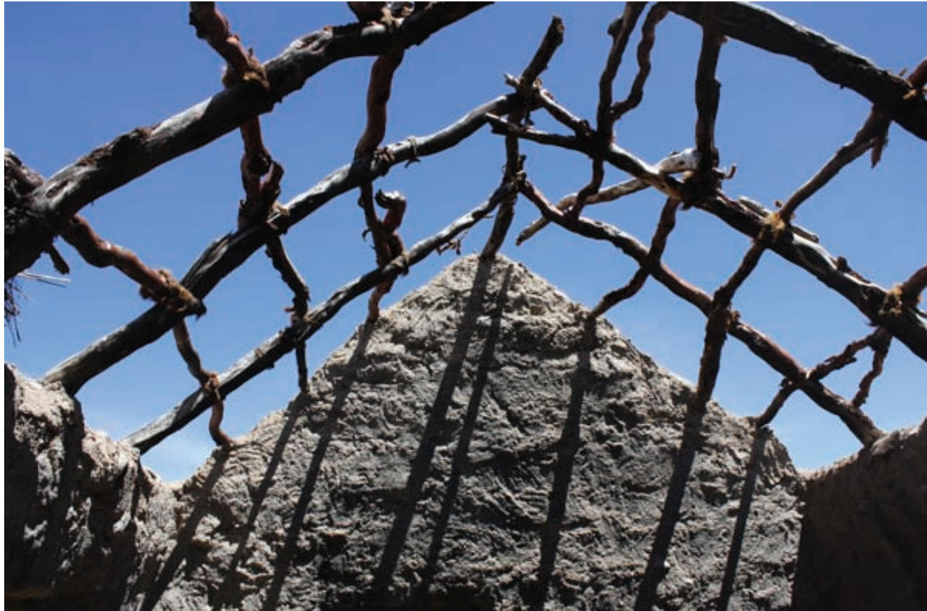
Fig. 3.30 Roof structure consisting in a wooden frame.
