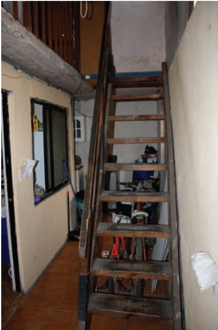
Fig. 5.81 Case 07, wooden staircases.
