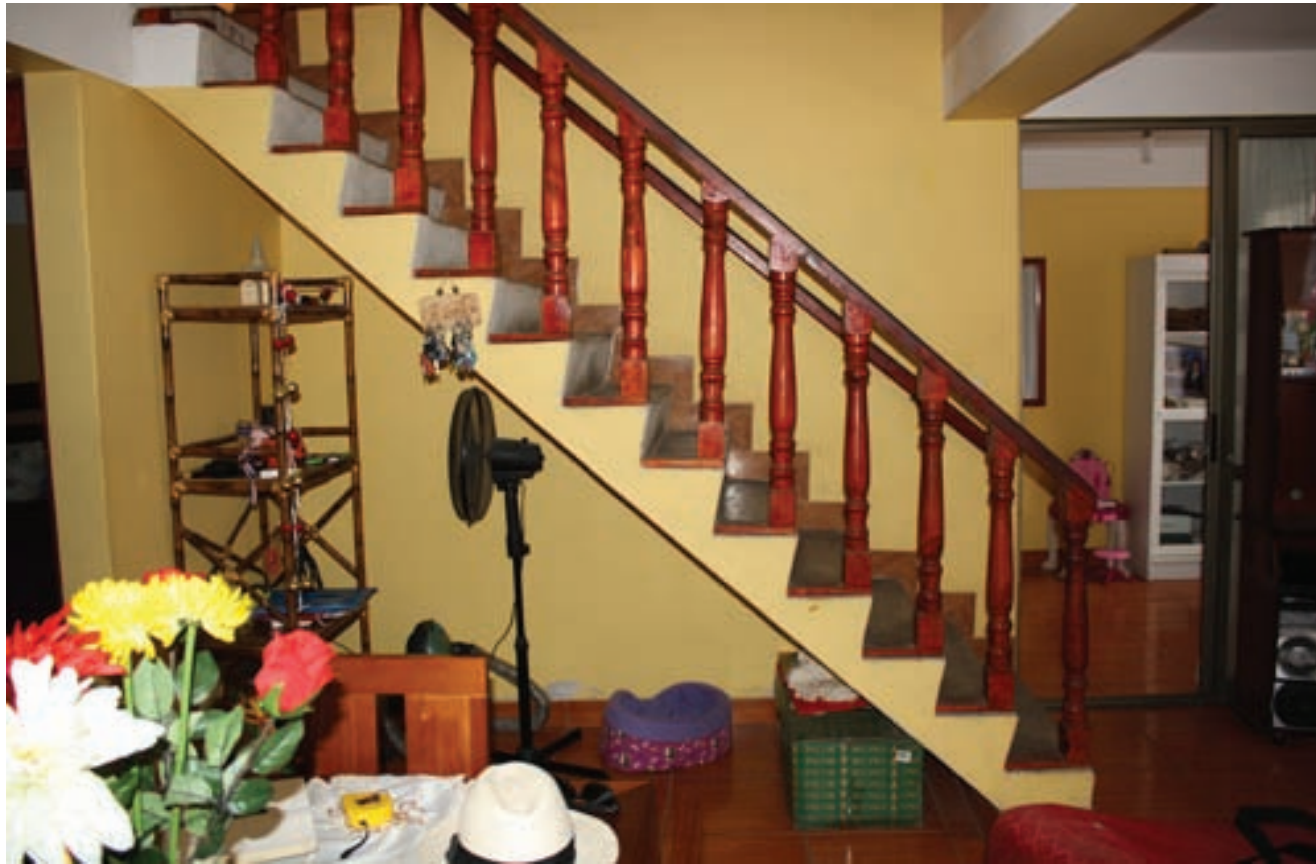
Fig. 5.88 Case 11, concrete staircase in the living + dining area.
