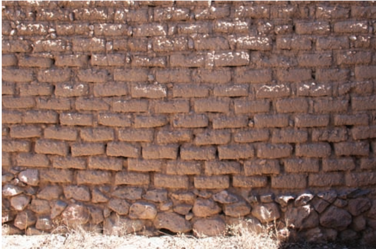
Fig. 3.16 A wall made of adobe bricks and stones.
