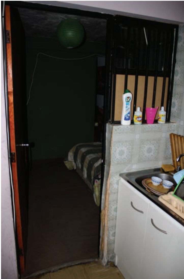
Fig. 5.41 Case 04, kitchen area and connection with the main bedroom.
