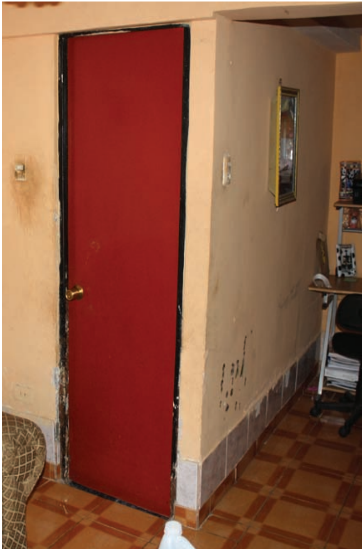
Fig. 5.23 Case 02, original bathroom on the ground floor.
