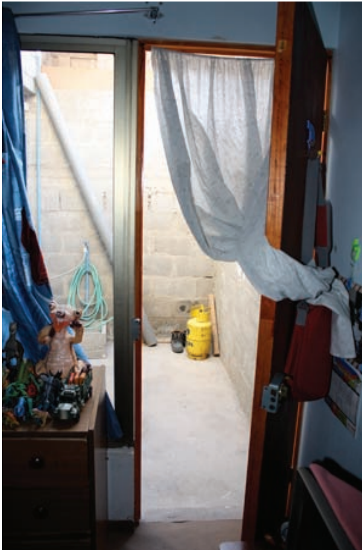
Fig. 5.52 Case 04, door from the bedroom to the backyard
