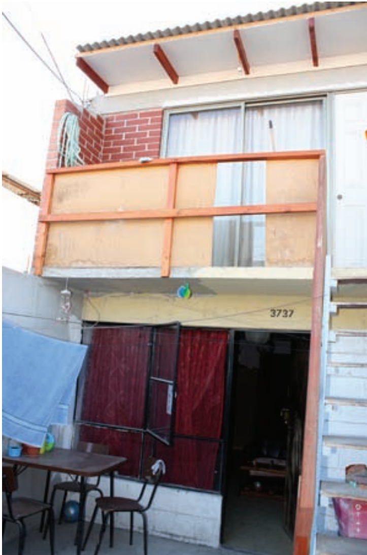
Fig. 5.45 Case 04, built second level.
