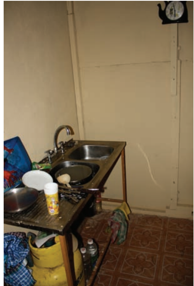
Fig. 5.60 Case 05, view of the kitchen space.
