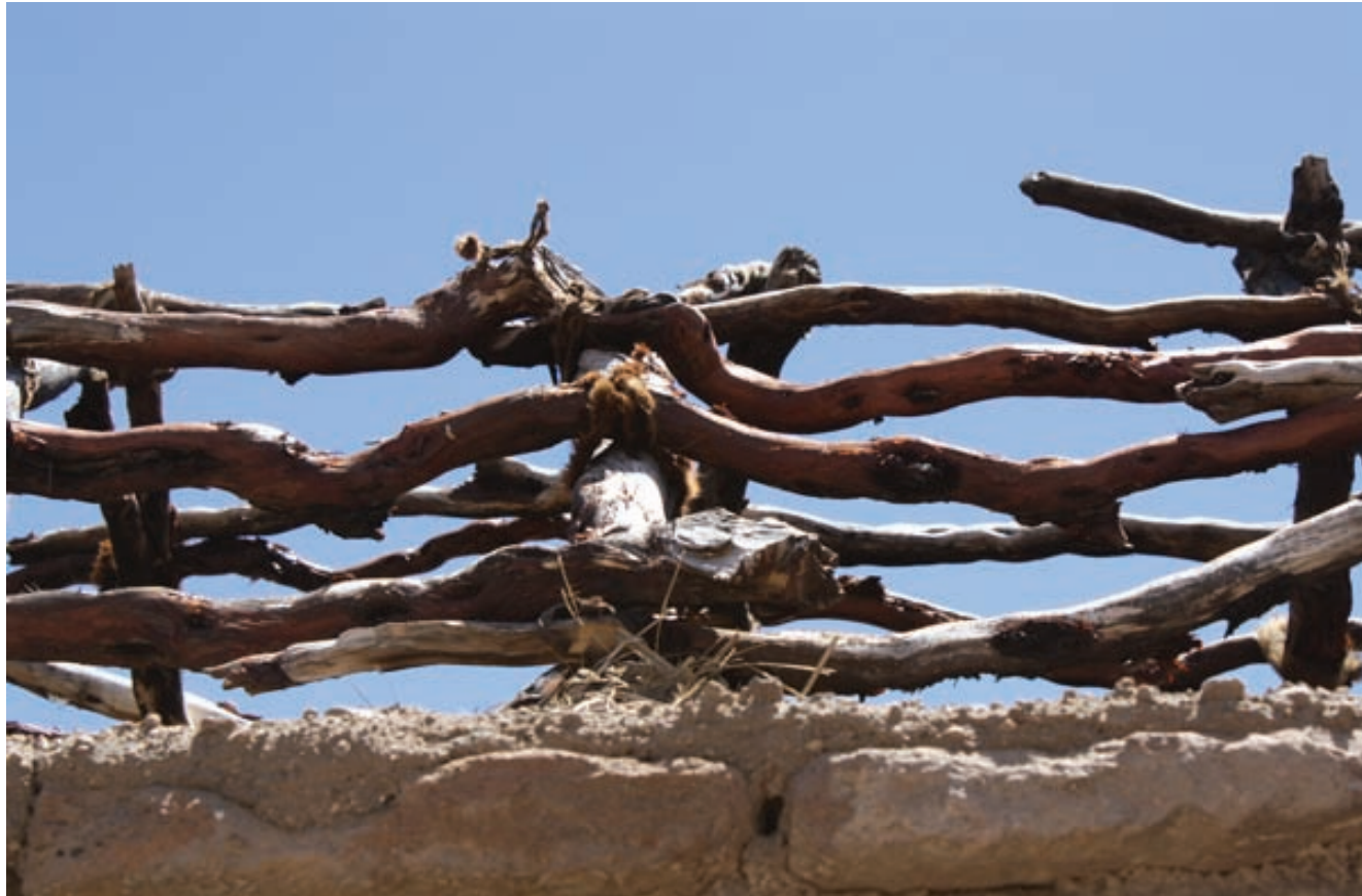
Fig. 3.31 The wooden frame is held by ropes or soaked leather strips.
