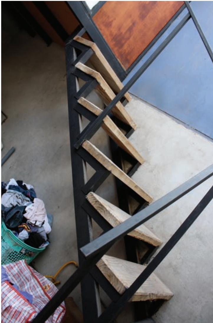
Fig. 5.21 Case 02, second staircase in the courtyard.
