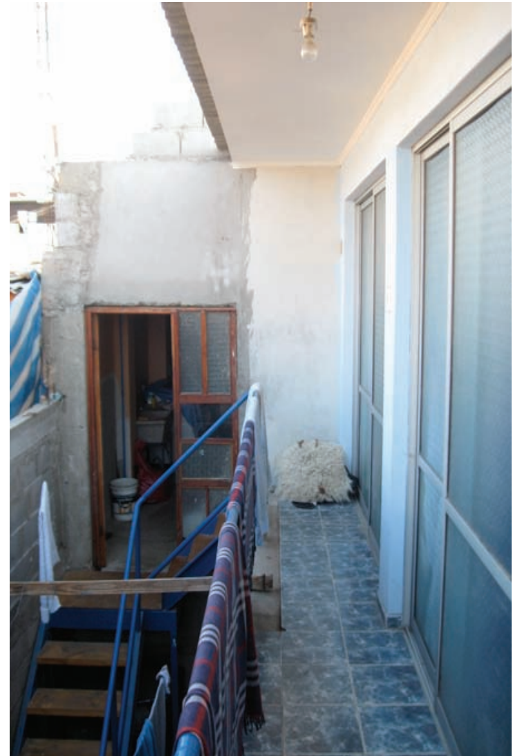
Fig. 5.31 Case 03, view of the rear room volume.
