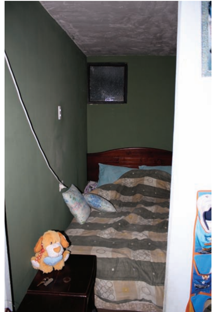
Fig. 5.40 Case 04, threshold between rooms, without door.
