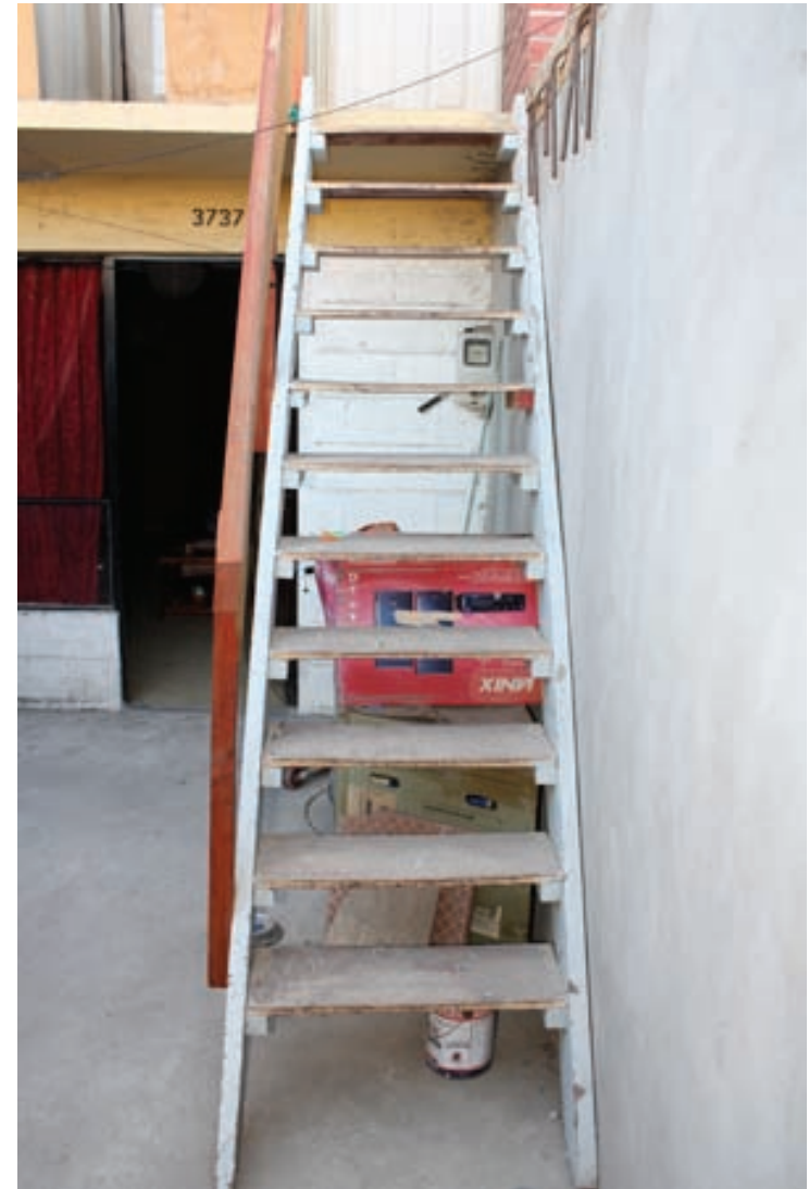
Fig. 5.46 Case 04, wooden staircase that connects to a balcony facing the front yard.
