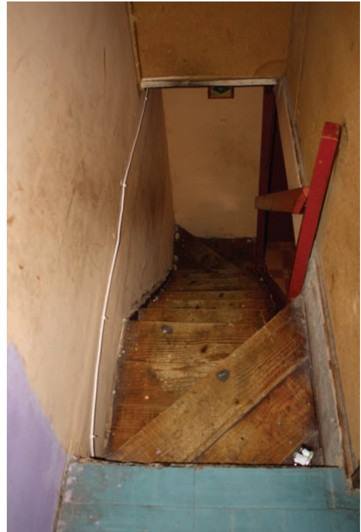
Fig. 5.17 Case 02, original staircase.
