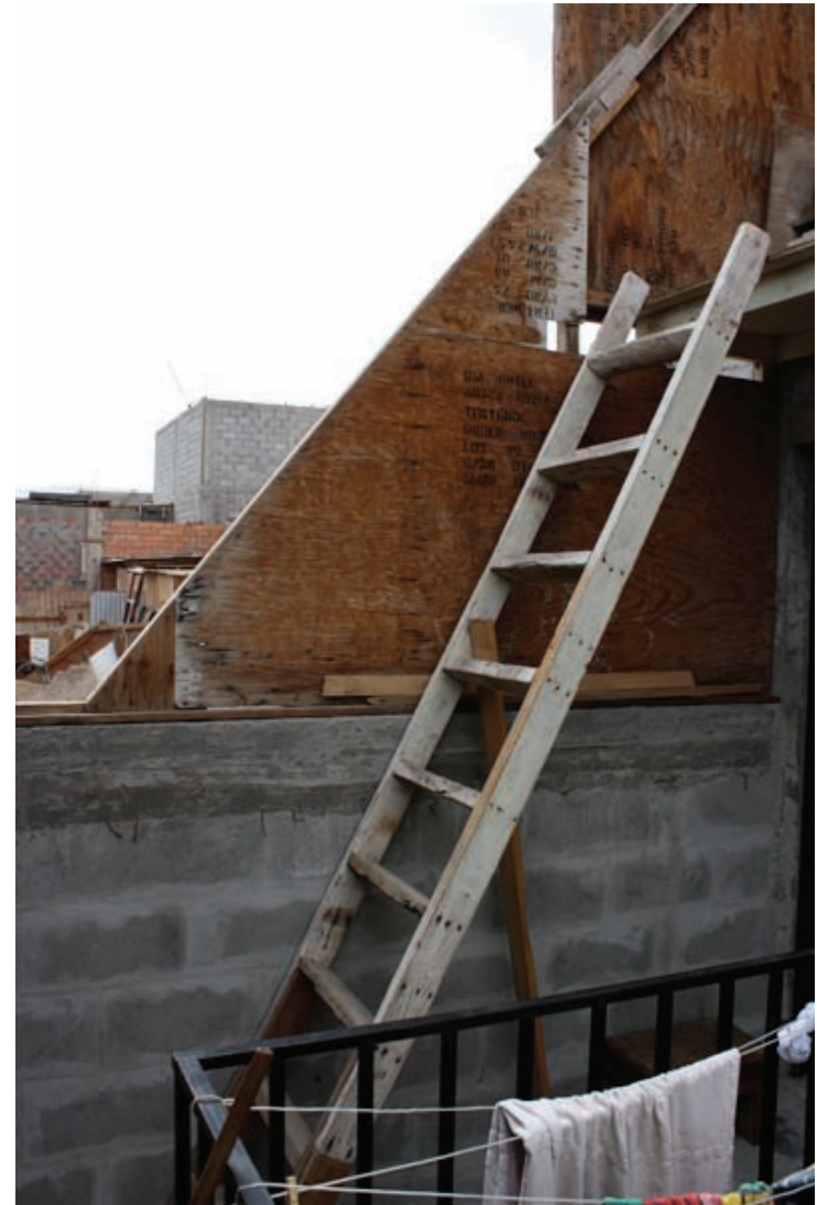
Fig. 5.8 Case 01, hand ladder to access the third level.
