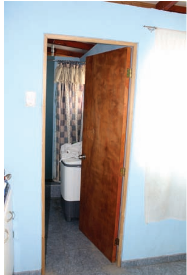
Fig. 5.53 Case 04, door between the kitchen area and the bathroom in the upper floor.
