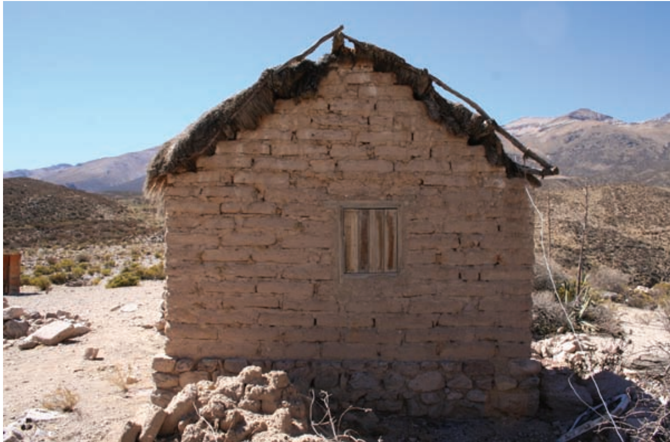
Fig. 3.29 A covered window in the uta.
