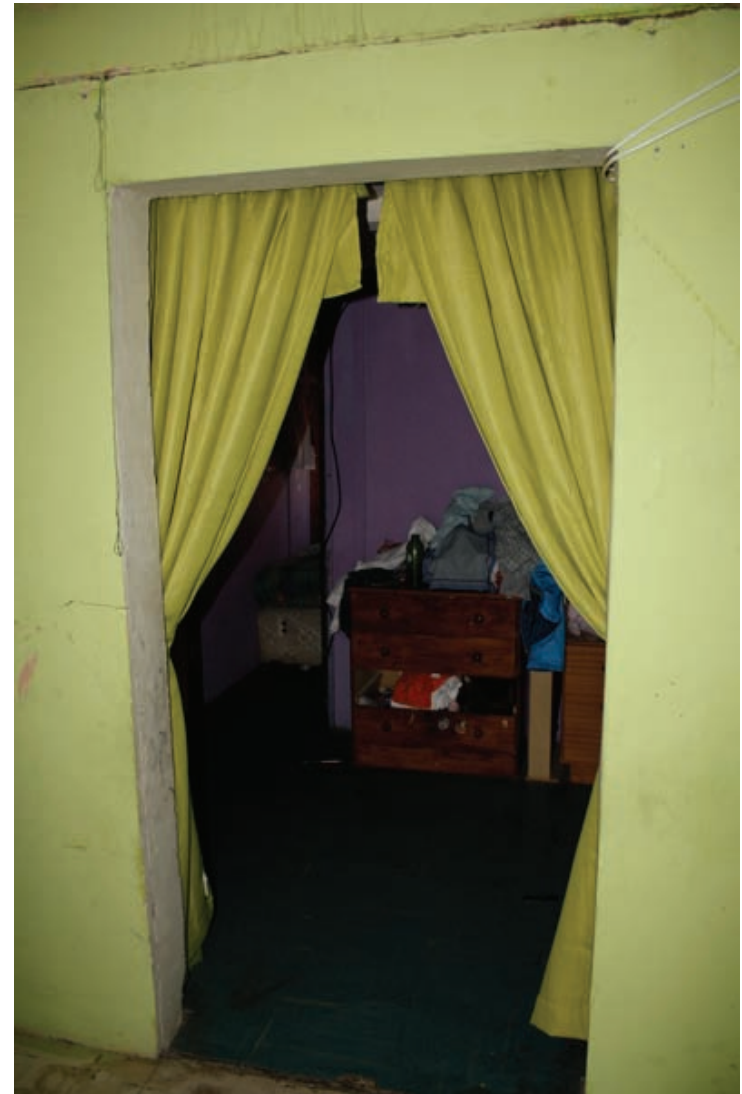
Fig. 5.19 Case 02, absence of doors between rooms.
