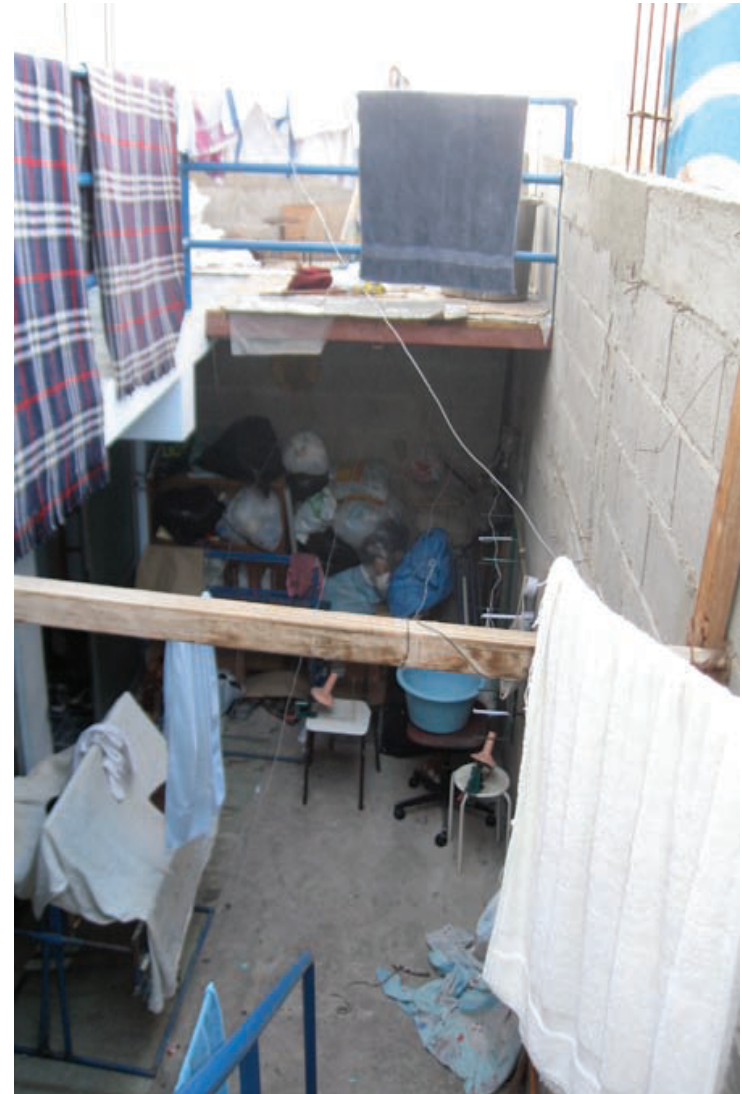
Fig. 5.35 Case 03, courtyard covered area.
