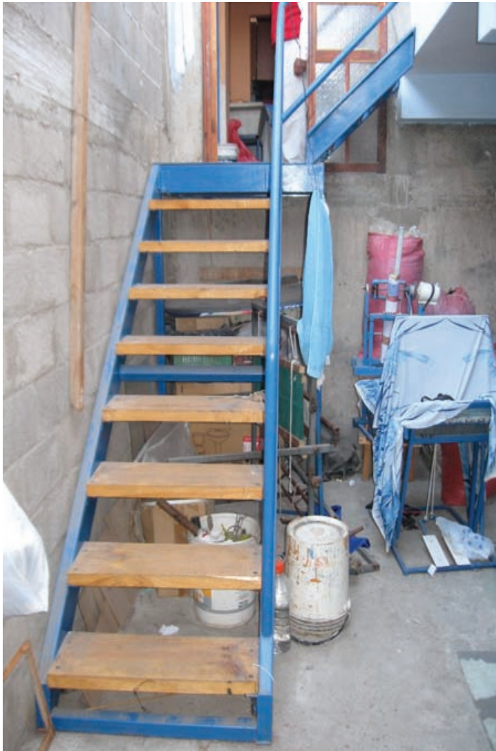
Fig. 5.30 Case 03, external staircase.
