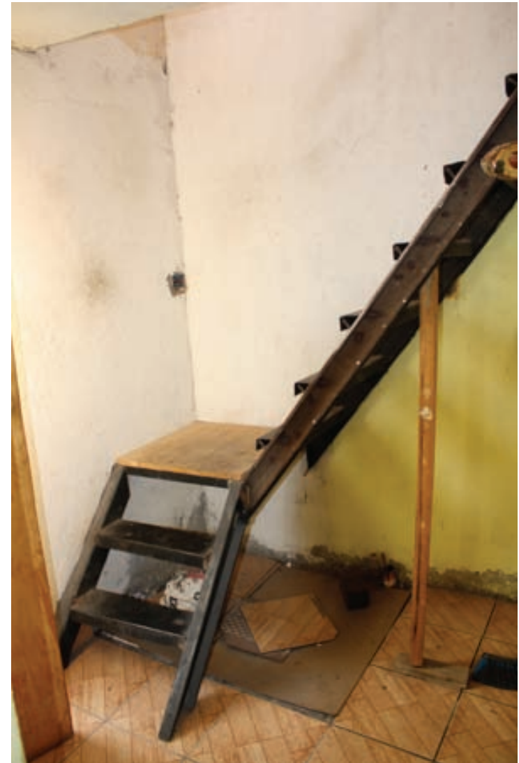
Fig. 5.68 Case 06, metal staircase that connects to the upper level.
