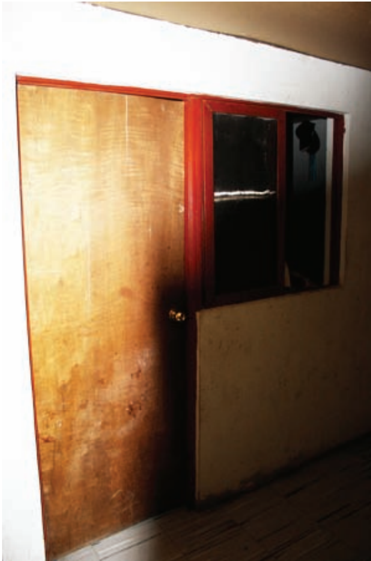
Fig. 5.65 Case 06, view of one of the enlarged bedrooms entrance.
