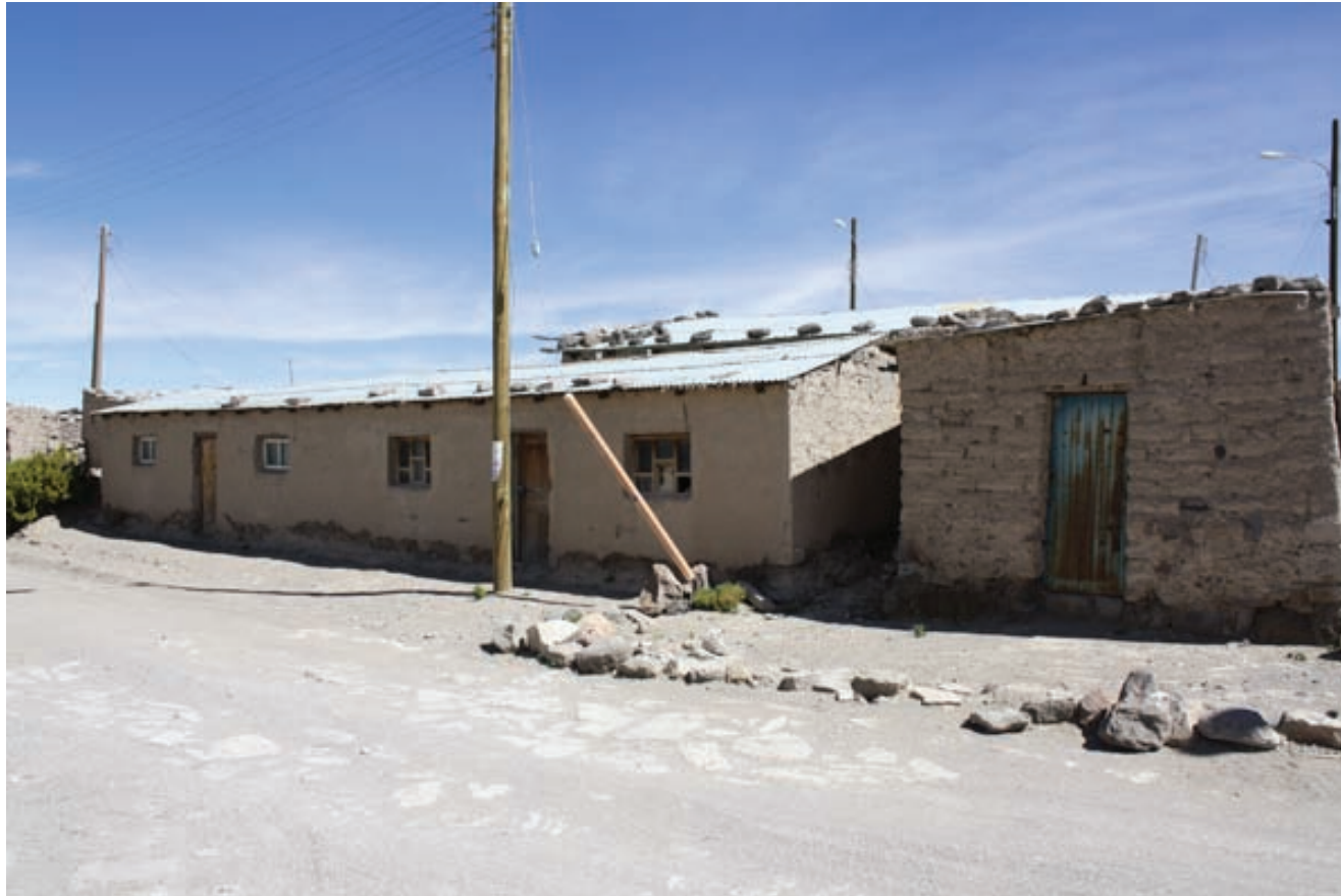
Fig. 3.4 House in the central and ceremonial town (marka)
