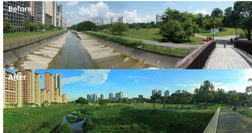
Figure 3.6: Photo showing the concrete canal passing through Bishan Park in 2008 (top) and the naturalized river after the transformation of the Bishan Park-Kallang River in 2011 (bottom). Source: Leonard Ng, Atelier Dreiseitl (2011)
