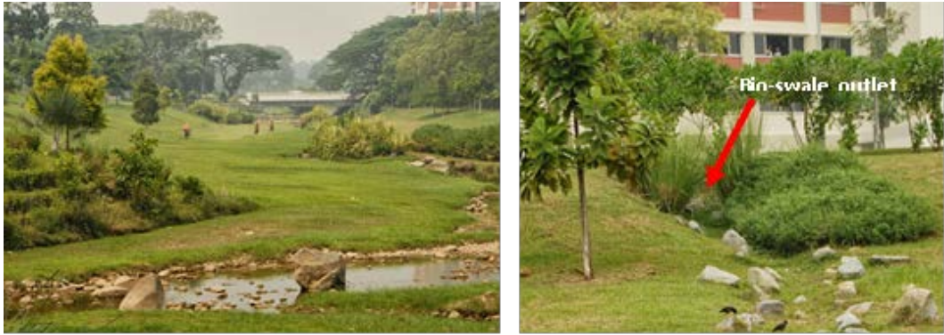
Figure 5.18: Photo showing the “smart mowing” at certain areas of the Kallang River (left) and the bioswale that requires regular de-silting (right).
