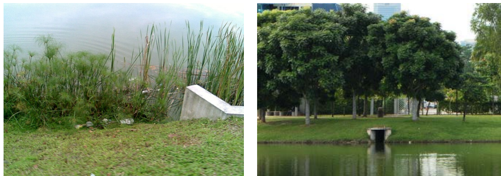
Figure 6.20: Photo showing rubbish trapped between the wetland plants at the ALG (left), requiring the park management to clear out the vegetation at drainage inlet sources into the lake (right)
