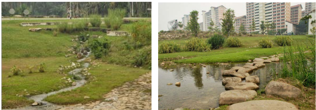
Figure 5.1: Photo showing the sustainable urban drainage system (SuDS) linked to the naturalized river for managing storm water (left); and the same space can be utilised by the public.
