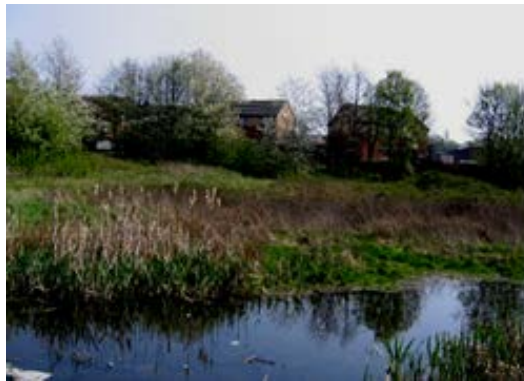
Figures 5.3: A photo showing the existing water source transformed into a retention pond as part of the SuDS component for the Manor Fields Park, using landscape for stormwater control and treatment, at the same time serving as a public amenity and creating habitats for wildlife. Source: Roziya Ibrahim (2013)
