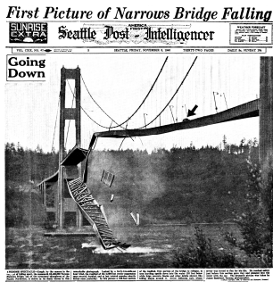
The infamous Tokoma Narrows Bridge collapsed in 1940 after violent torsions caused by winds [323].
