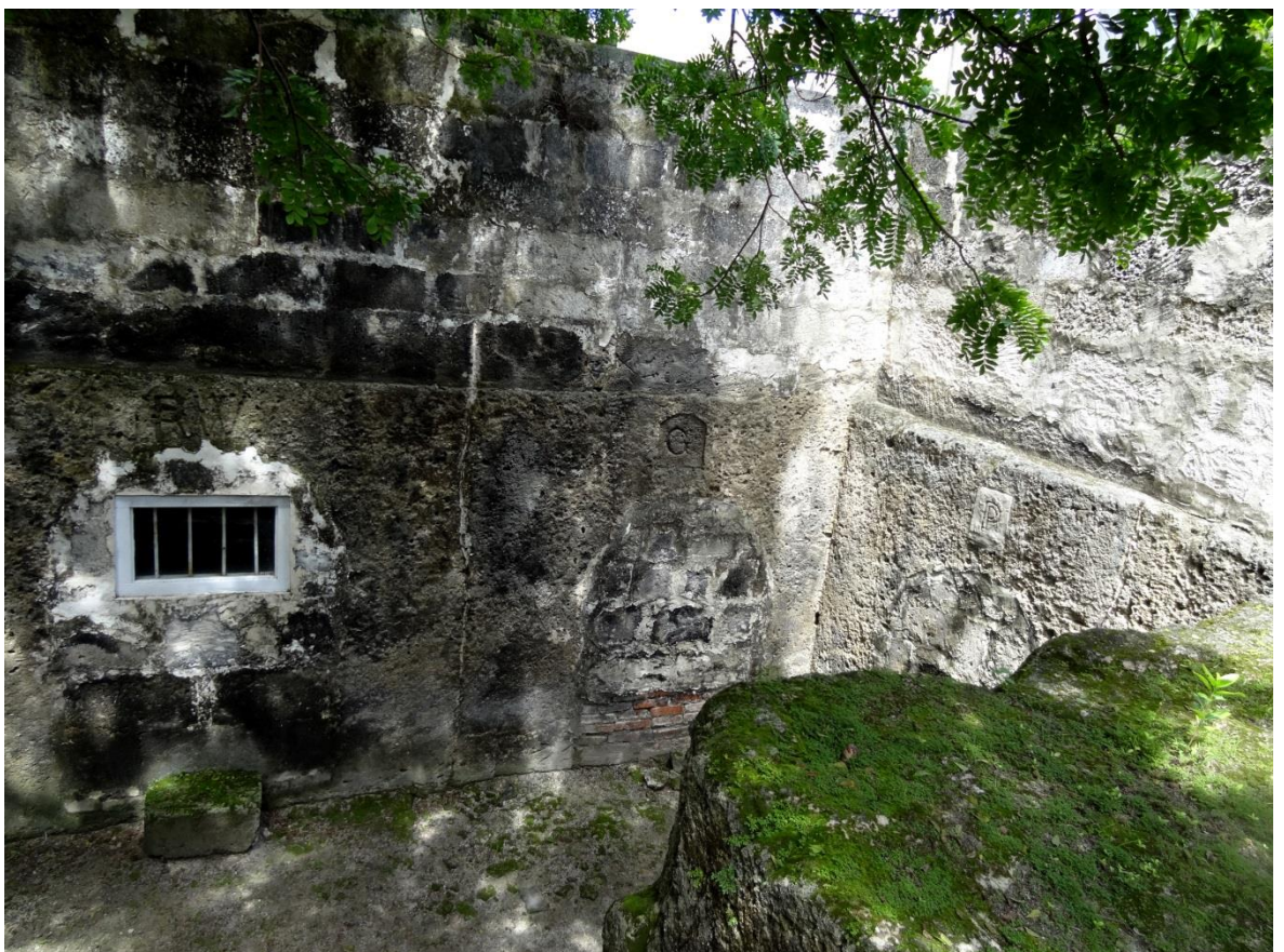
Figure 154 Interior of Quaker Burial vault in St. Philip's Parish.
