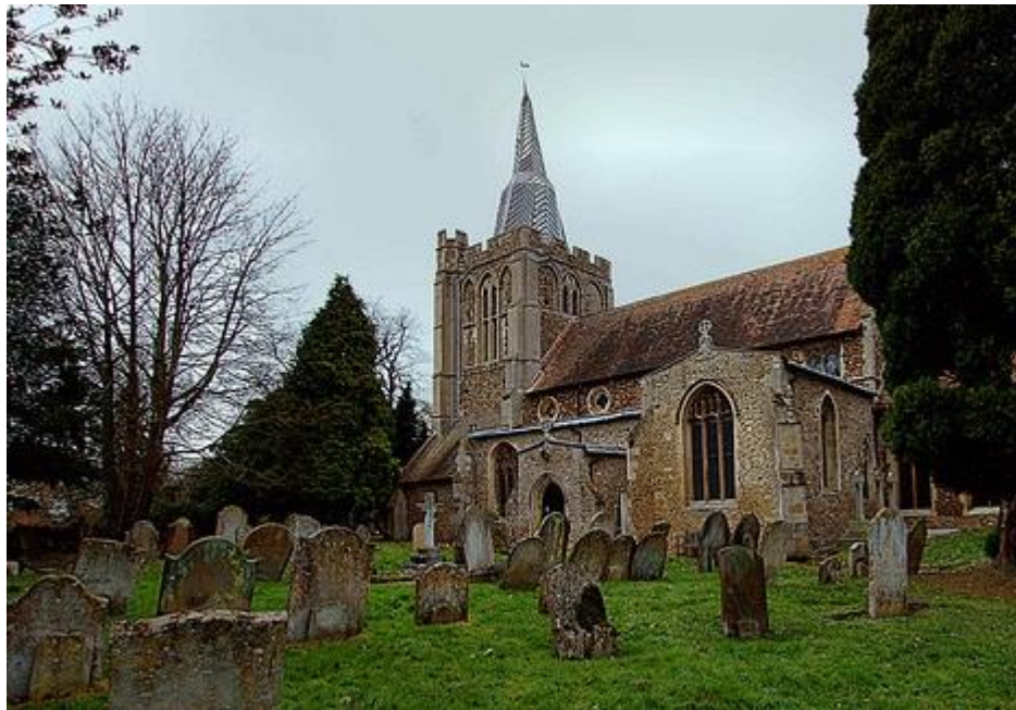
Figure 188 Exterior of the Church of St. Mary's and St. Helena's (Miller n.d.).
