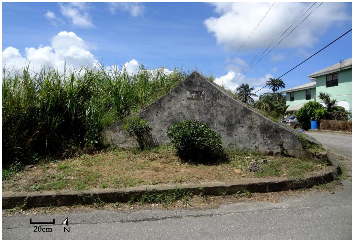
Figure 156 Williams Vault, from Welchman Hall Plantation.
