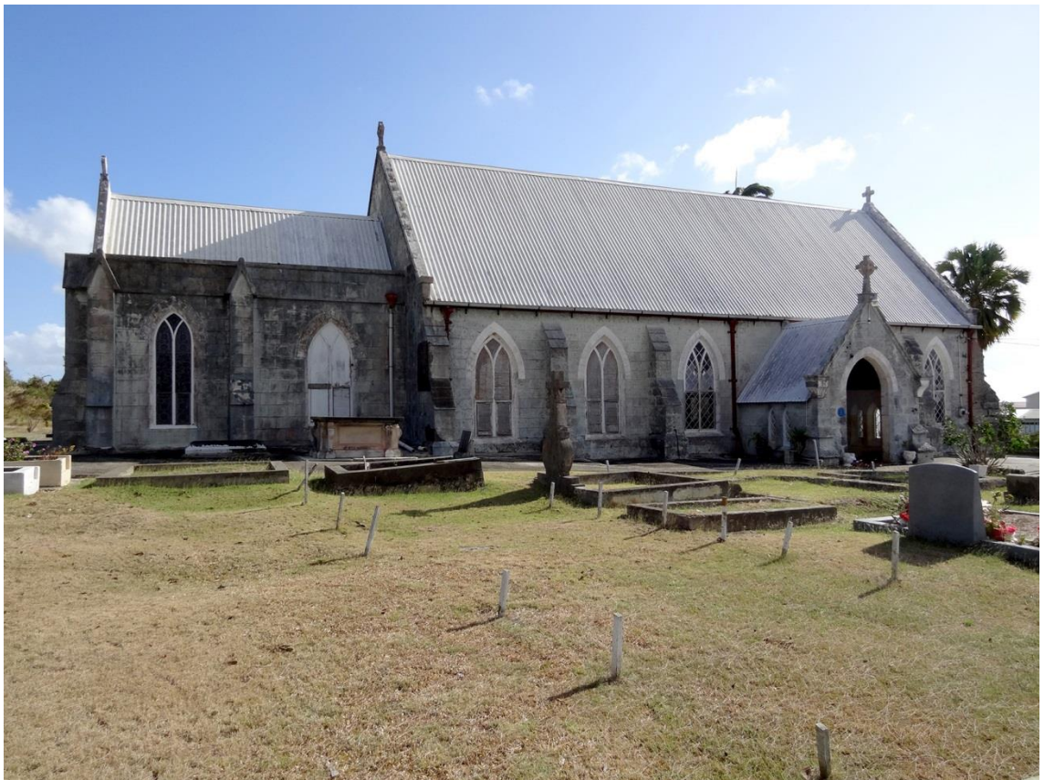
Figure 96 All Saints Chapel, St. Peter's Parish, Barbados. Northern side.
