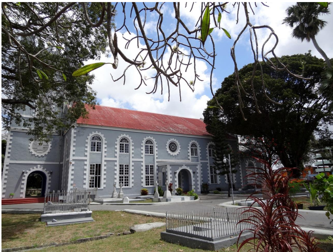
Figure 123 St. Mary's Chapel, Bridgetown, Barbados. View from southern section of churchyard.
