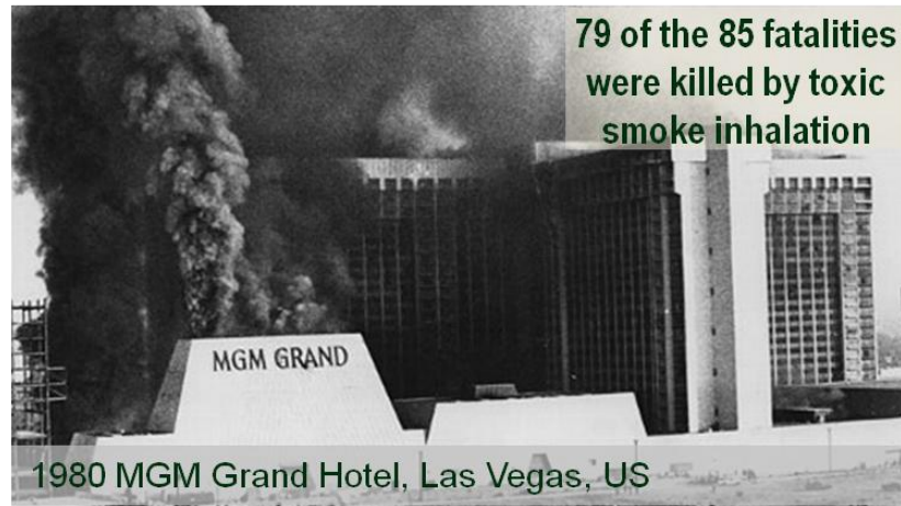
Figure 1-7: Picture of the MGM hotel during the fire showing the smoke dispersing from various areas in the building [18].
