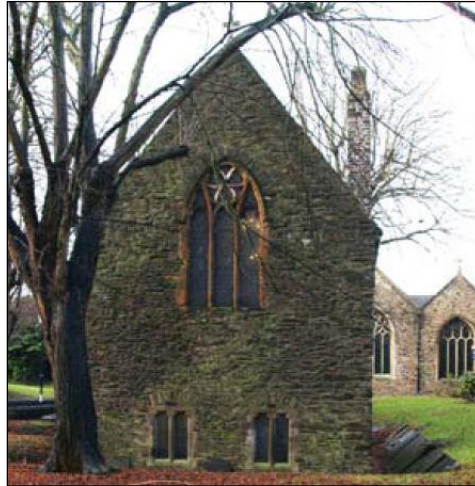
Fig. 5.4: St Anne's chancel chapel, Barnstaple from the east (Cox 2001: 7). Note the large east facing windows on both levels and deliberate slanting of ground level surrounding the building to allow light to enter the lower level and highlight the room from the exterior.
