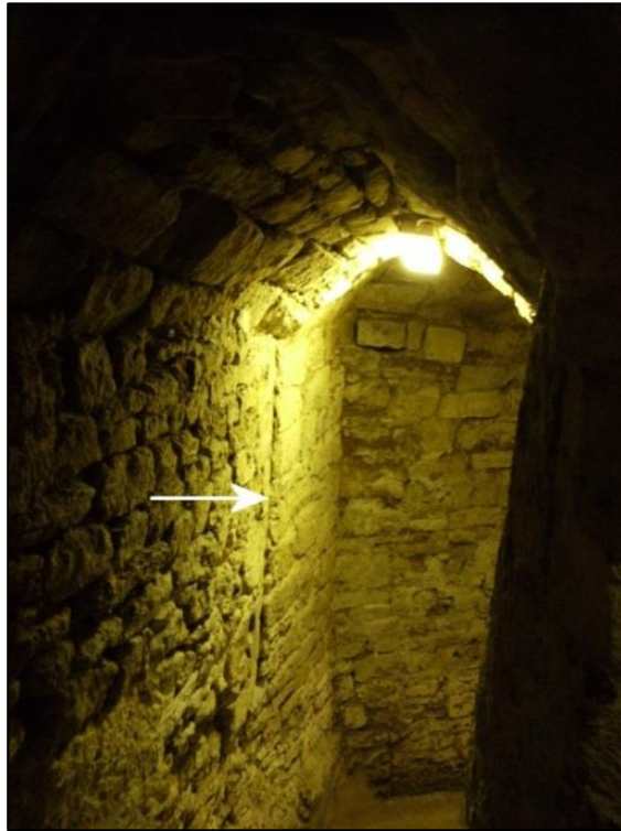
Fig. 5.30: The blocked up niche at the end of the staircase leading to the crypt (location indicated by arrow) (Photograph author's own)
