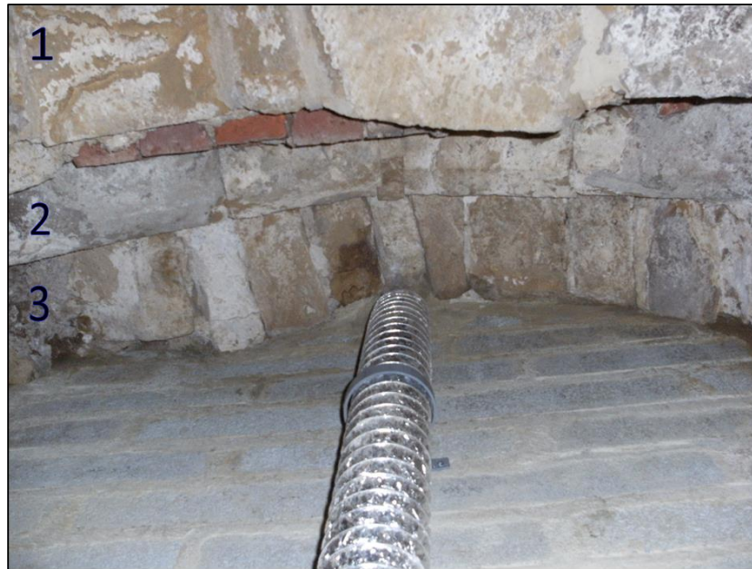
Fig. 5.21: One of the two windows in the south wall of the crypt, with the triple arches at their apex highlighted. Note the brickwork between the first and second arches that has not been dated but may date to the porch construction in the 19 th century, as it is of the same material (Photograph author's own)
