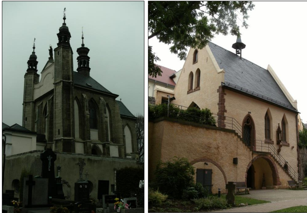
Figs 5.7 & 5.8: The charnel chapels of Kutná Hora, Czech Republic (left) and Oppenheim, Germany (right), both founded in 1400. Note the same architectural features of windows into the lower charnel rooms as in the English examples in Fig. 5.4. The upper levels of these buildings also served as chapels, with disarticulated bones stored in the lower rooms (Photographs author's own)
