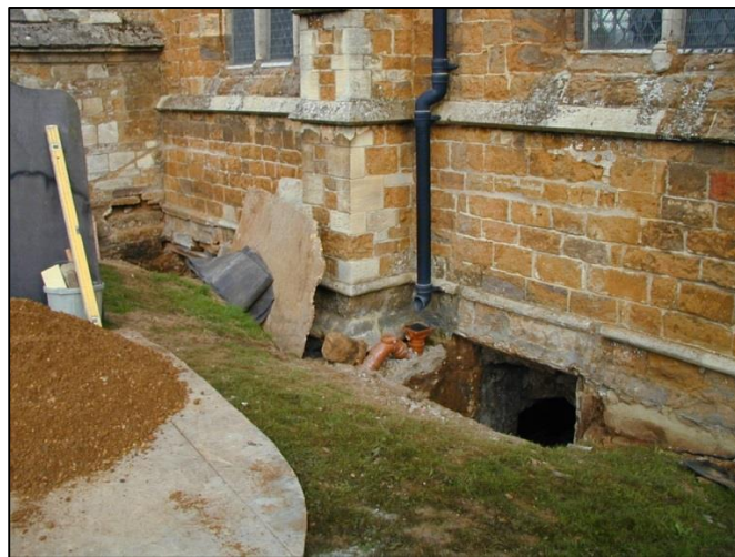
Figs. 5.19 & 5.20: The westernmost window into the crypt at the time the current ventilation system was installed (mid 1990's). Note the masonry extending outwards from the window and chamfered stonework and frame of the window (above). The stonework is visible from a depth of c. .3-.5 meters below current surface level of the cemetery and the interior of the crypt is visible from a significant distance away from the windows (below) (Photographs reproduced with permission of Rothwell Holy Trinity church authorities).
