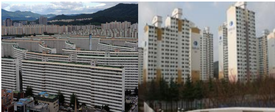
Figure 2.16 Image of apartment buildings with two types: corridor type (left) and stari type (right) (Source: http://news.naver.com/main/read.nhn?mode=LSD&mid=sec&sid1=101&oid=015&aid=0002204036 , http://www.hdapt.com/g4/bbs/board.php?bo_table=tb_apt_5&wr_id=66&top_menu=6&top_sub=3 )
