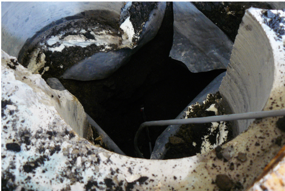
Figure 6.14: Installation of sensors at the test property.
