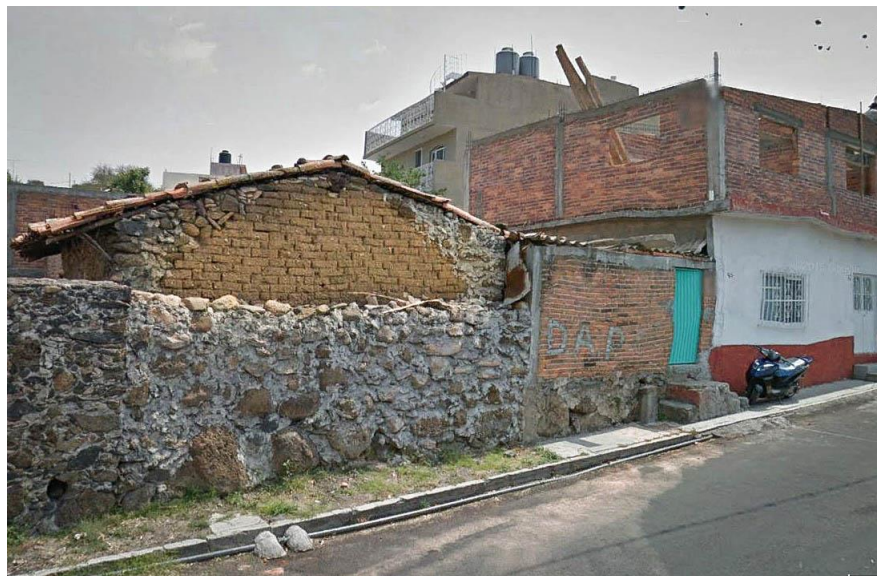
Figure 5.3 Adobe replaced by industrialized building materials
